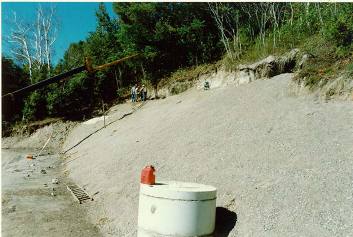
PHOTO 11: Crane Working at the Limit of its Reach.
