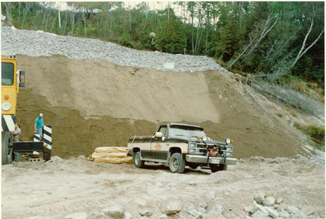
PHOTO 13: Topsoil in Place on Lower Slope.
