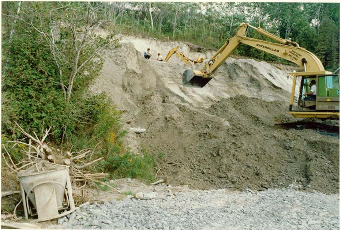
PHOTO 7: Cleaning and Grading Lower Slope.
