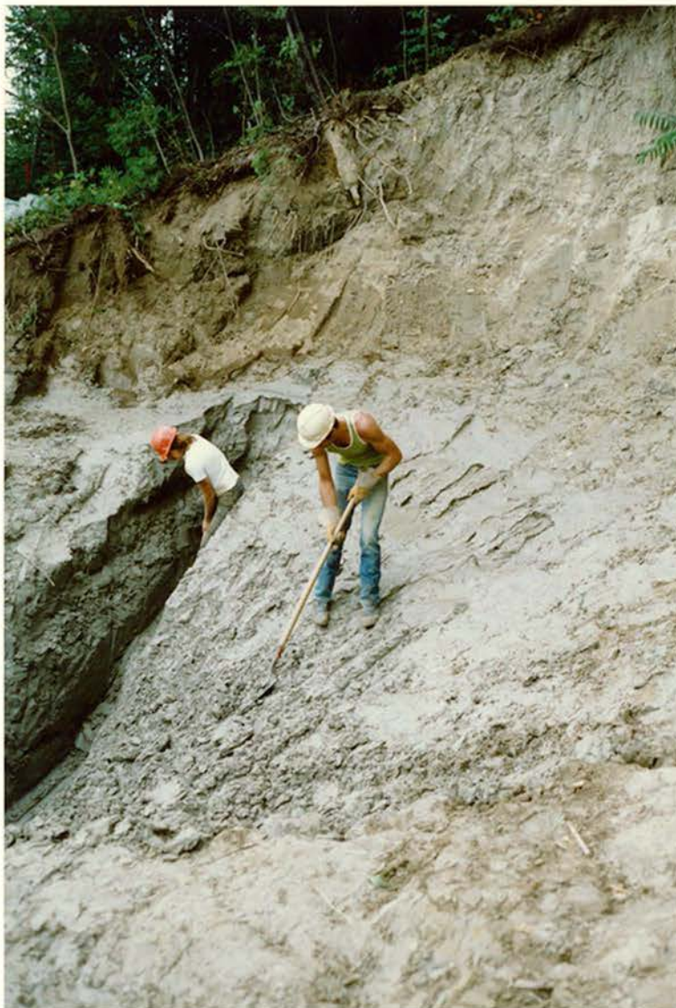
PHOTO 5: Excavation of Drainage Trench at West End of Site. Sloped Portion of Trench is in Lacustrine Silt.
