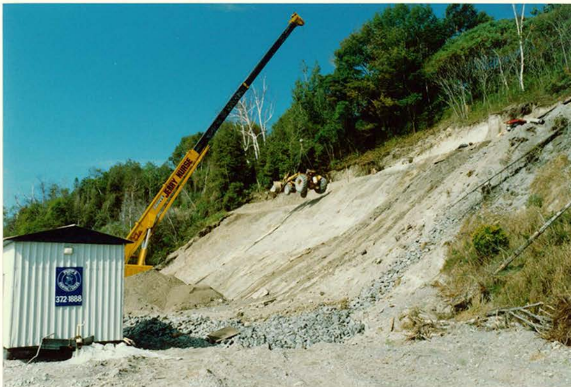
PHOTO 9: Demobilizing Case 580 Excavator (in two pieces).
