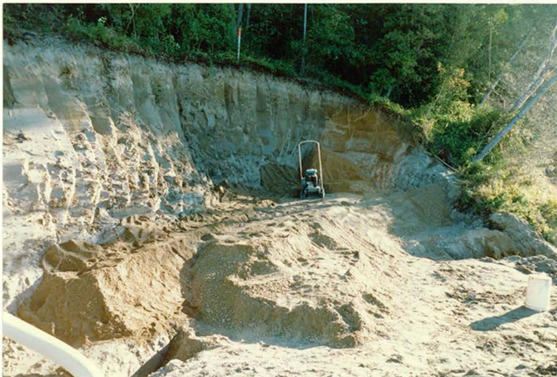
PHOTO 3: Initial Placement of Sand Filter and Granular "A" Material at East End. Note: part of this area was subsequently re-excavated to install the catch basin.
