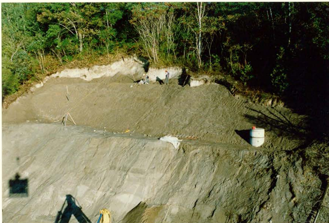
PHOTO 10: Nearing Completion of Sand Filter and Granular "A" Placement.
