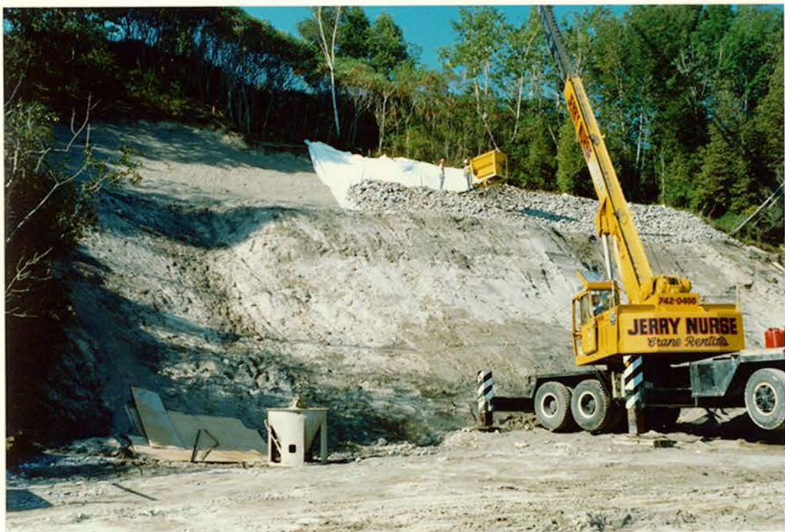
PHOTO 12: Rockfill Placement.
