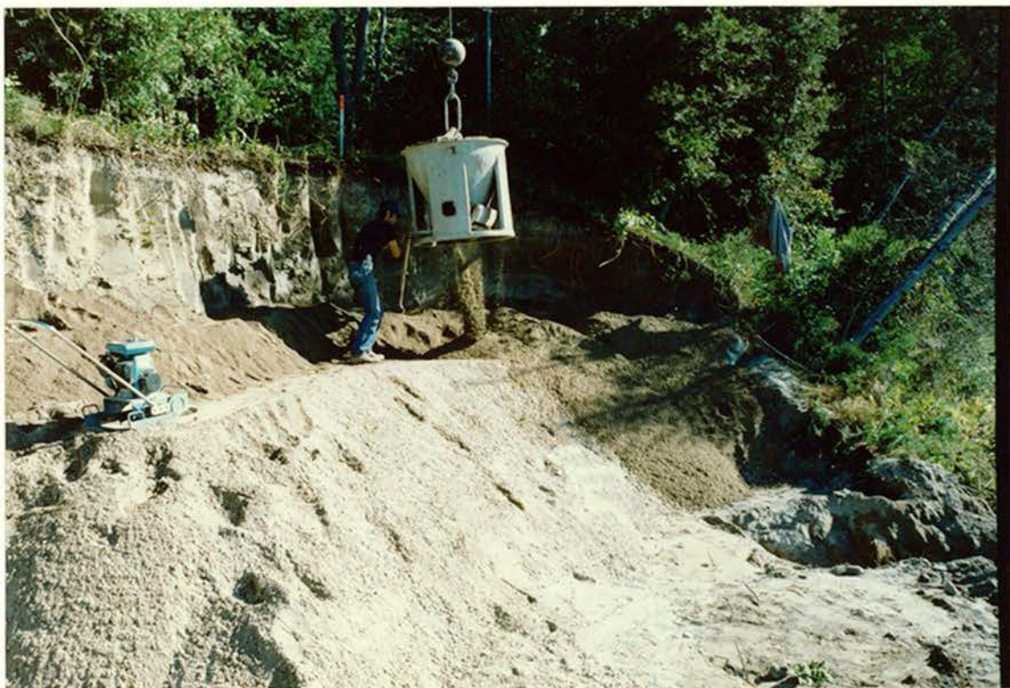
PHOTO 4: Initial Placement of Sand and Granular "A" Material at East End. Note: part of this area was subsequently re-excavated to install the catch basin.
