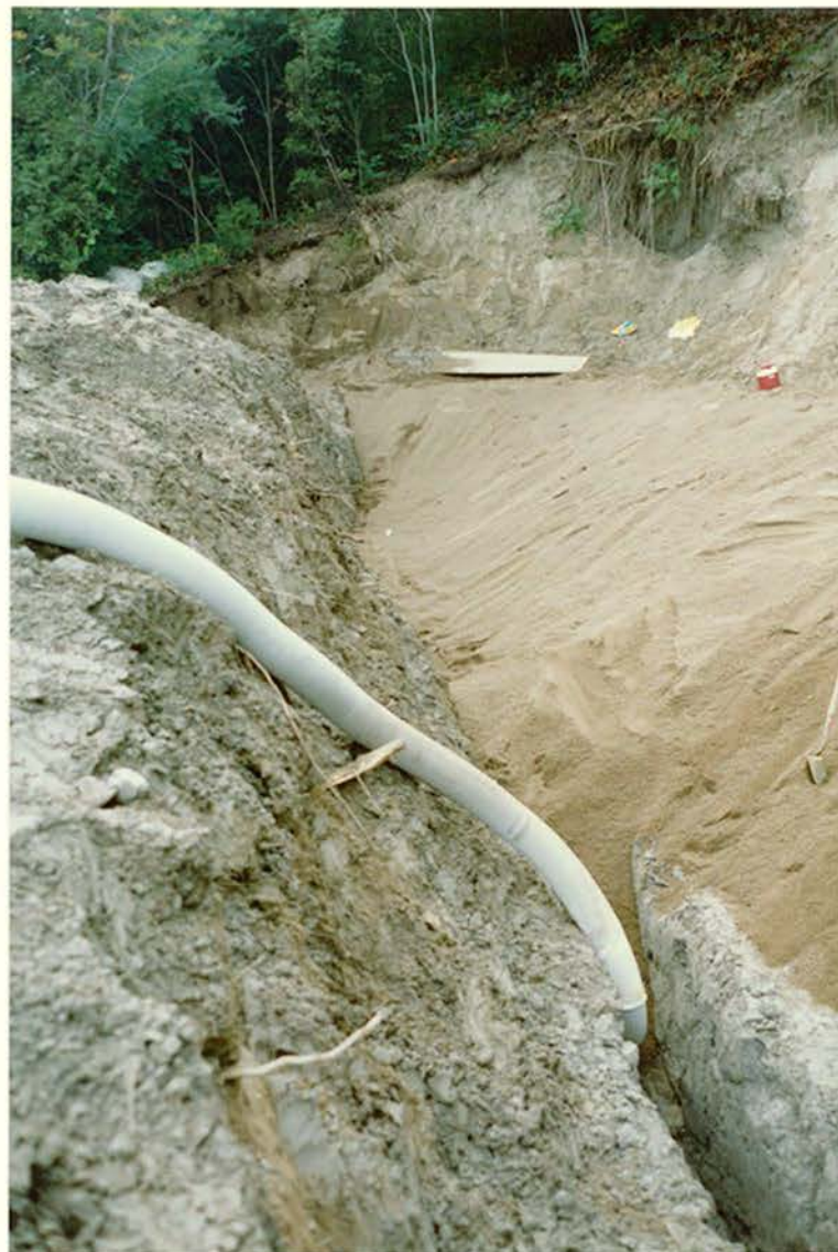
PHOTO 6: Drain Pipe and Initial Lift of Filter Sand in Place at West End of Site.
