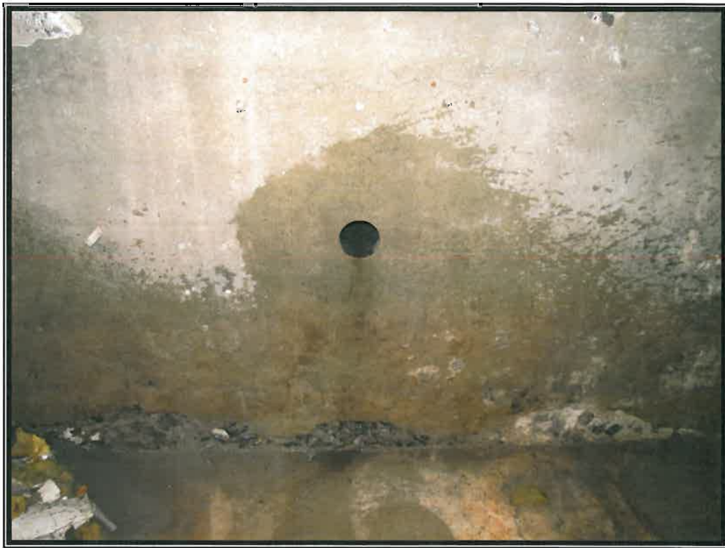
Picture 9 : Sample (C-2) of the front wall of the east building, below grade. (2013-06-06)
