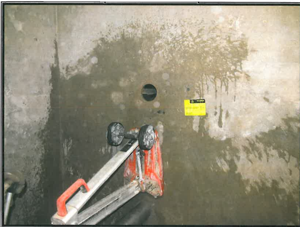
Picture 5 : Drilling of the exterior stone facing of the right wall of the east building (2013-06-06)
