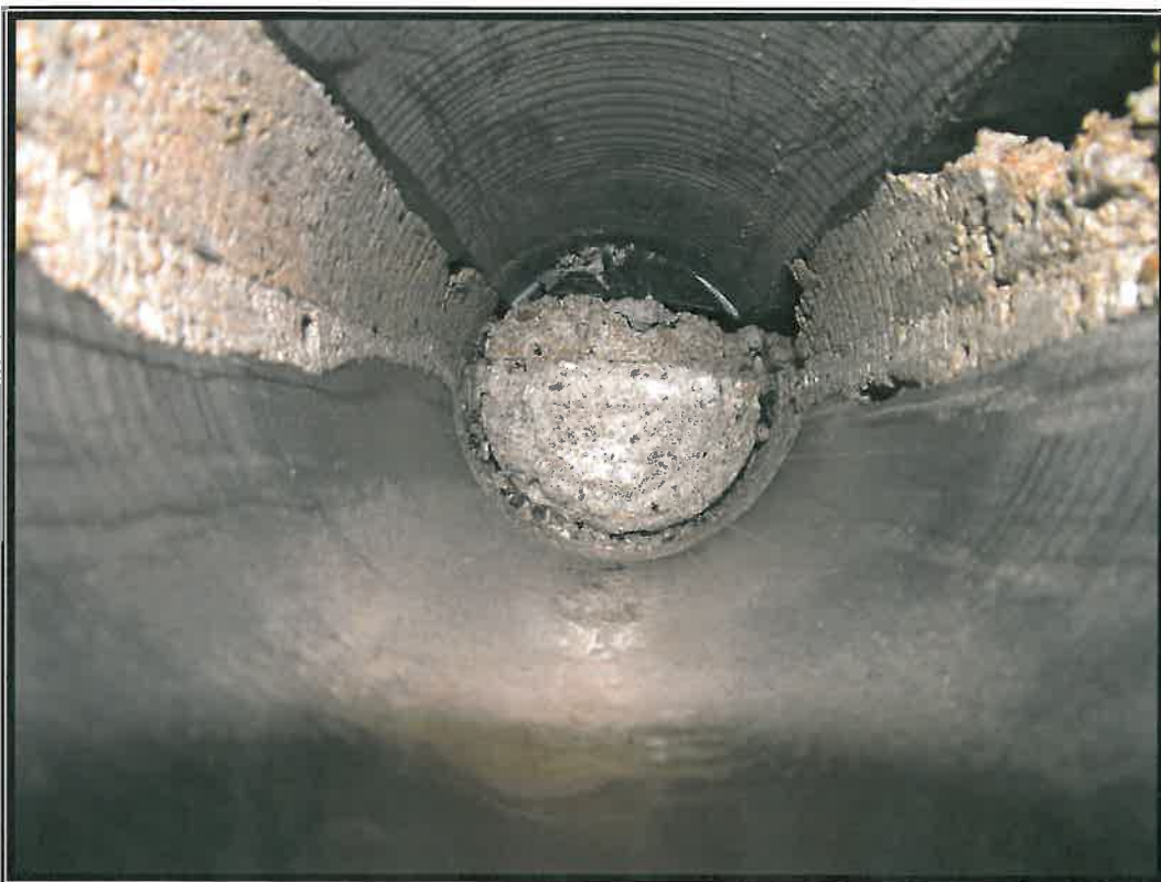
Picture 6 : Inside view of the core through the right wall of the east building (2013-06-06)
