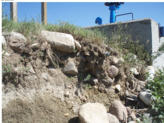
Highfield Dam - Dam Upstream Erosion at the West Low Level Outlet Photo No. 2 Looking towards the structure
