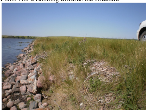
Highfield Dam - Dam Upstream Erosion and Debris Photo No. 3 Looking west along the dam upstream slope
