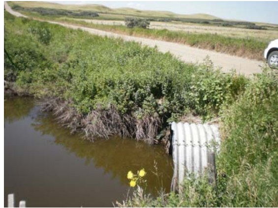
A Local Road Culvert Crossing – 18.9 km Downstream of the Highfield Dam Photo No. 4 Upstream end of the culvert crossing
