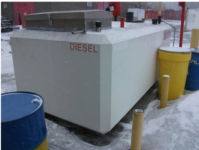
Photograph 23: Helicopter Hangar Building – Diesel Fuel Storage Tank
