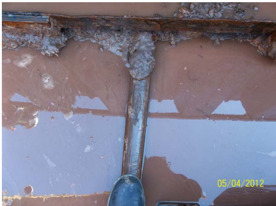
Photo 44 - TP 1 - Exposed tie-rod.
