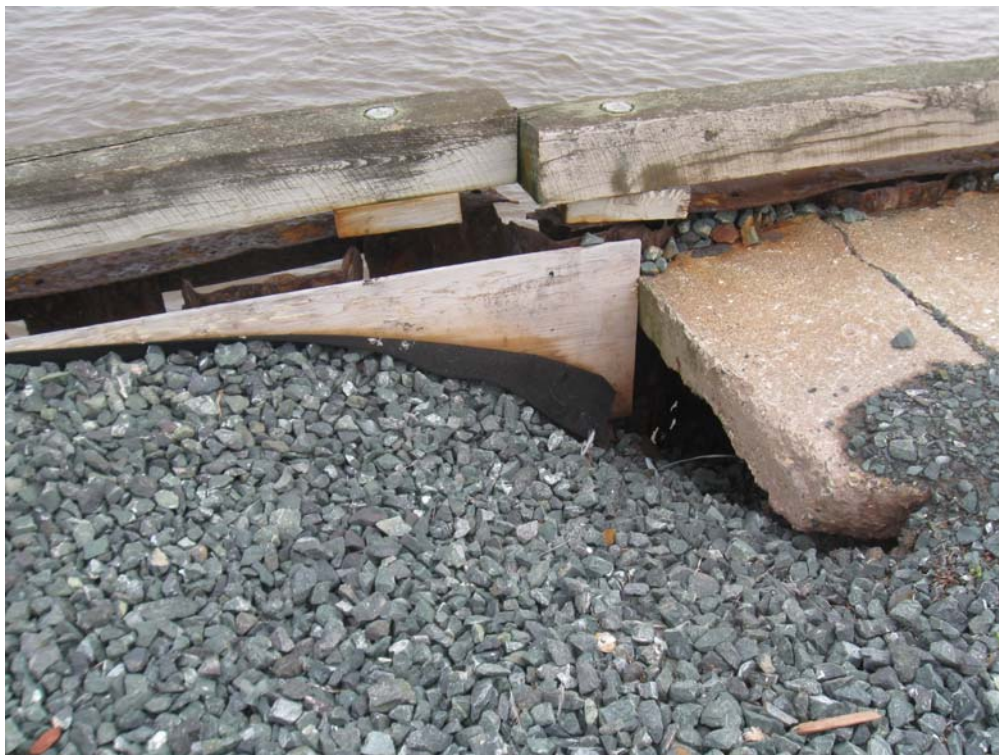
Photo No. 17: Loss of Material at Joint Between 1966 and 1968 Sections of Structure 302. (2011-11-29)
