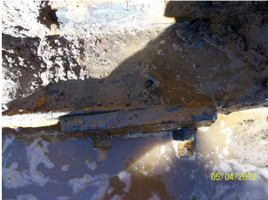
Photo 55 - TP 4 – Exposed back plate.
