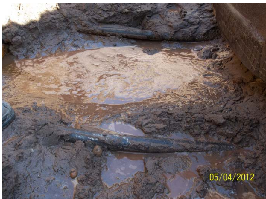
Photo 49 - TP 2 – Tie-rod spacing exposed.
