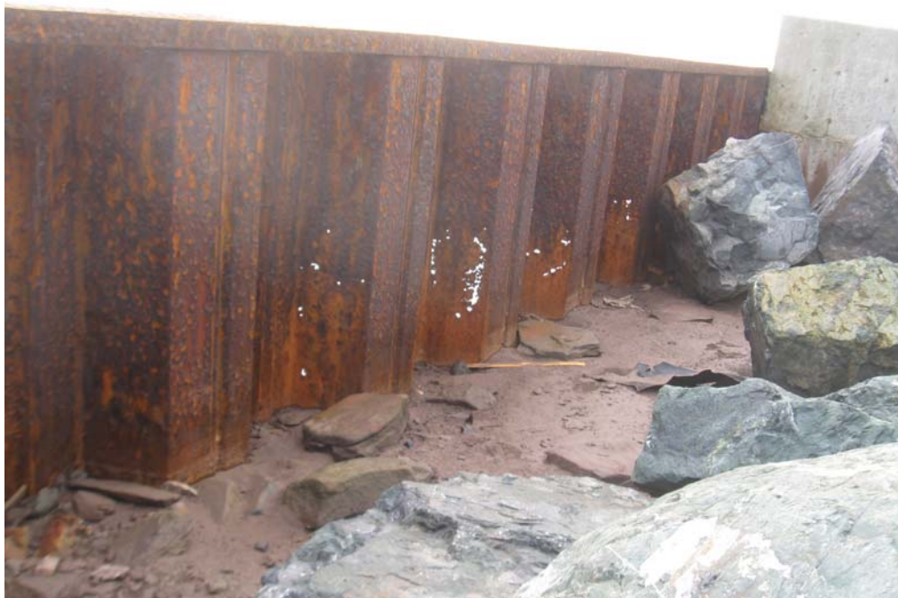
Photo No. 24: Perforations at South End of East Face – Structure 304. (2011-11-29)
