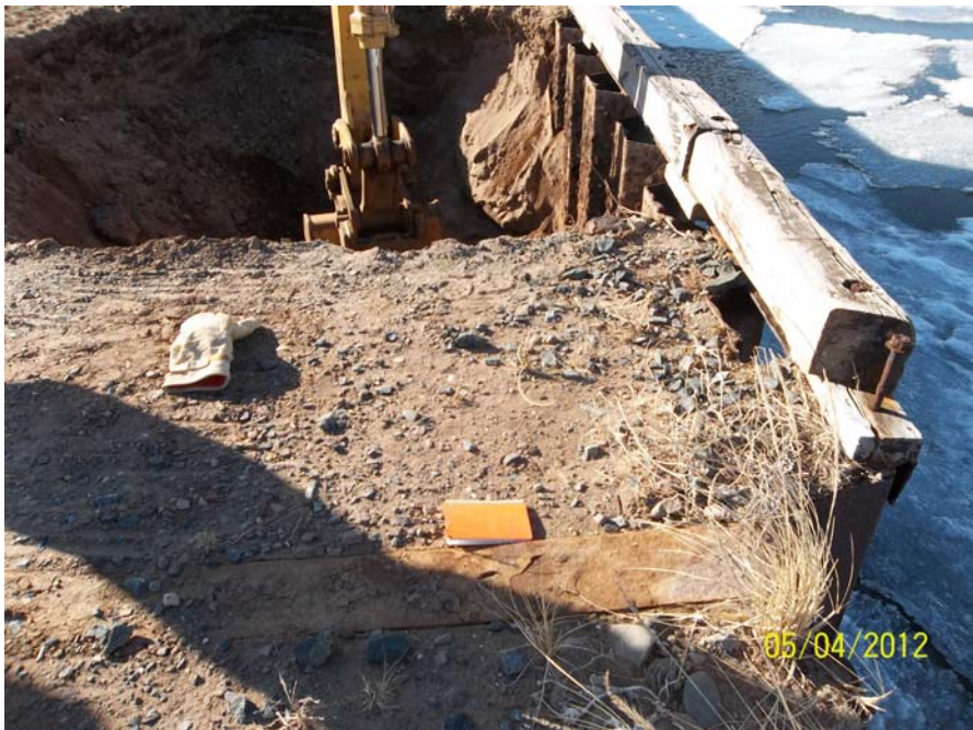
Photo 48 - TP 2 – Exposed Beach Sand Fill
