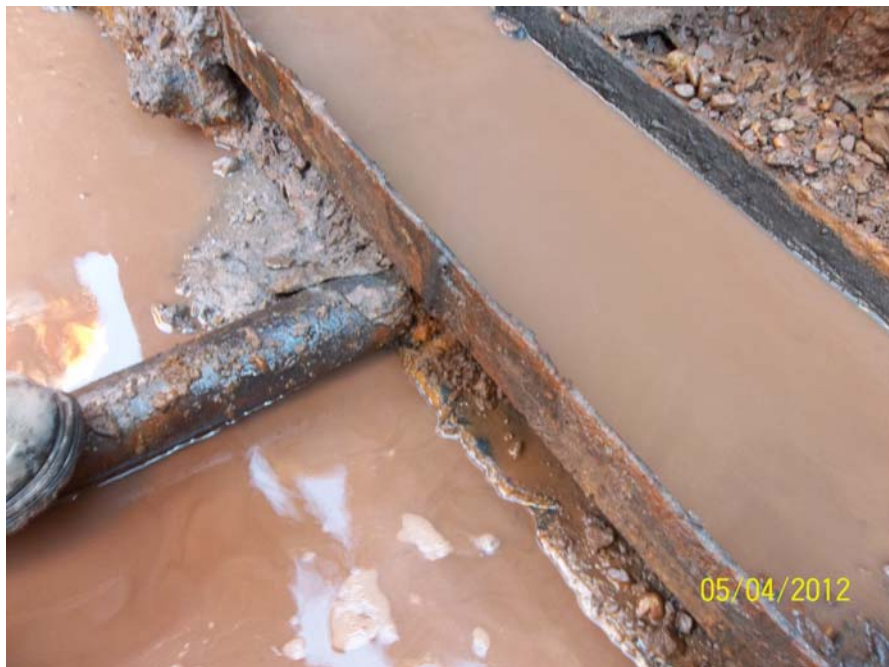
Photo 46 - TP 1 – Upper and lower channel of waler.
