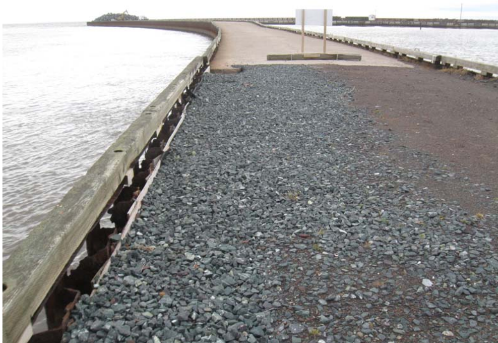
Photo No. 4: Gravel Fill where Material Loss Occurred Through SSP Face at South End of 1966 Section of Structure 302. (2011-11-29)
