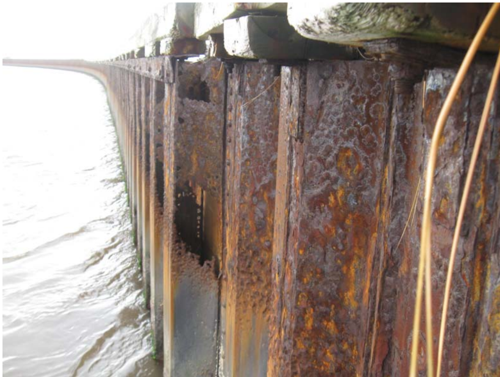
Photo No. 12: Perforations at Top of SSP Along Channel Face of Structure 302. (2011-11-29)
