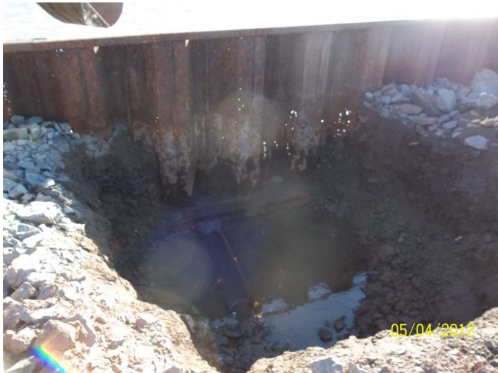
Photo 42 - TP 1 – Tie-Rods exposed and perforations in upper portion of SSP visible.
