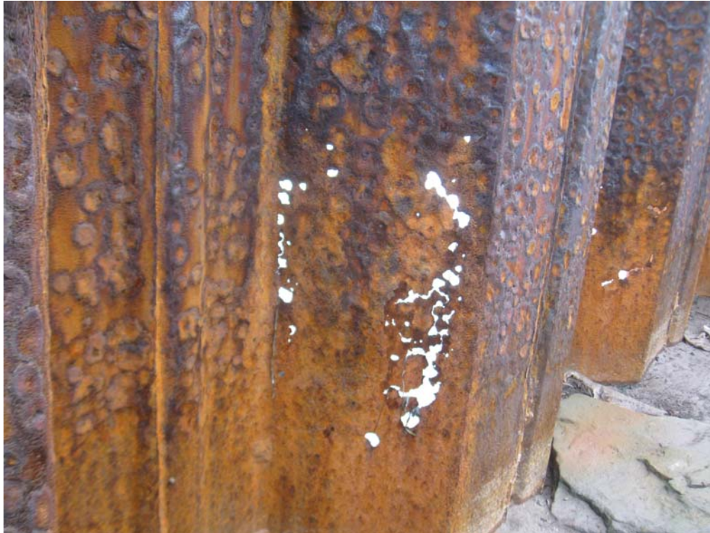
Photo No. 25: Severe Pitting and Perforations in Back Side of SSP East Wall - Structure 304. (2011-11-29)
