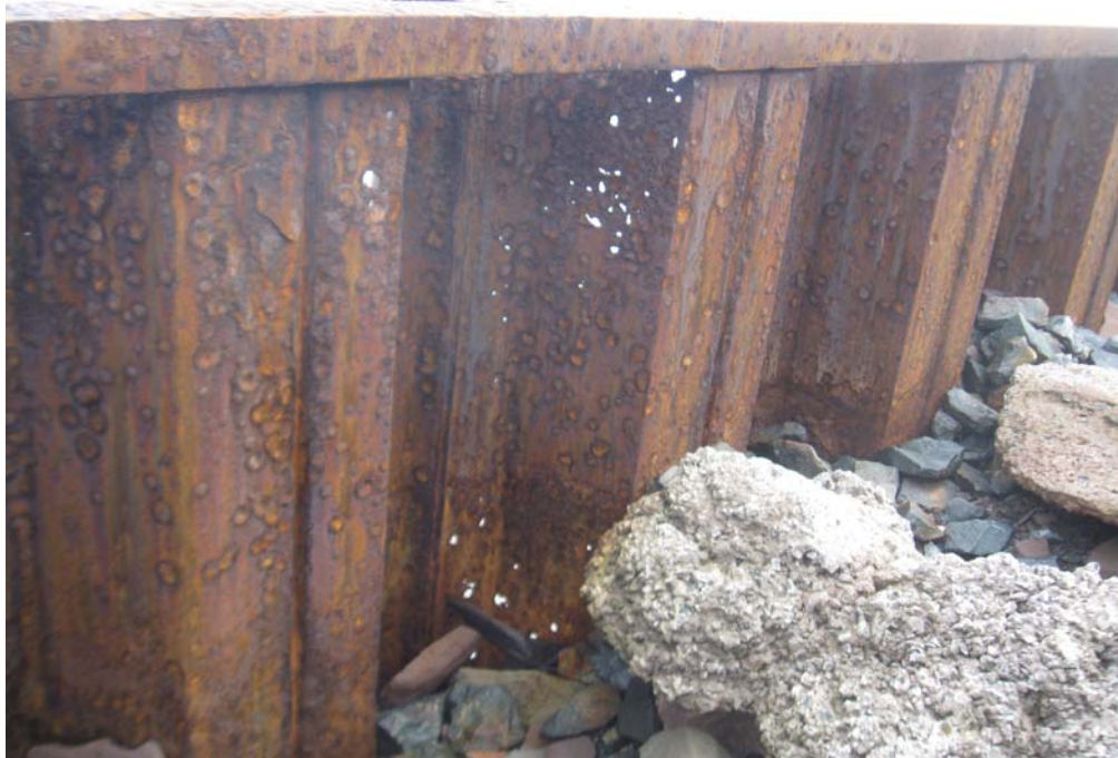
Photo No. 23: Severe Pitting on Back Face of SSP – East Wall of Structure 304. (2011-11-29)
