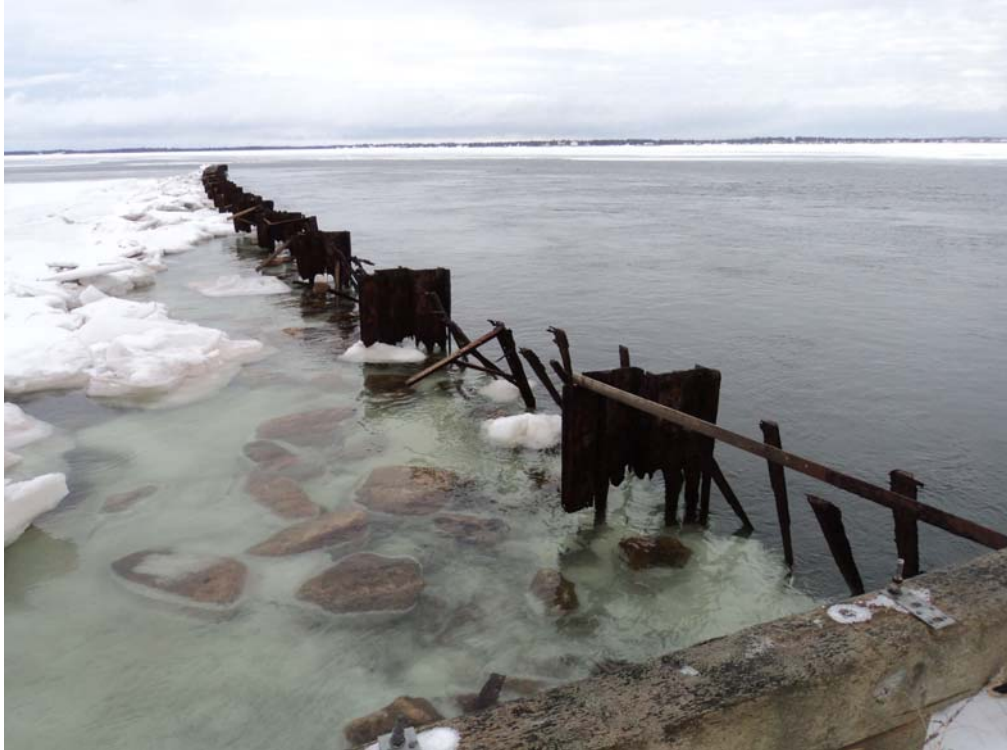
Photo No. 41: North of Structure 302. Remains of SSP Wall. (2012-02-08)
