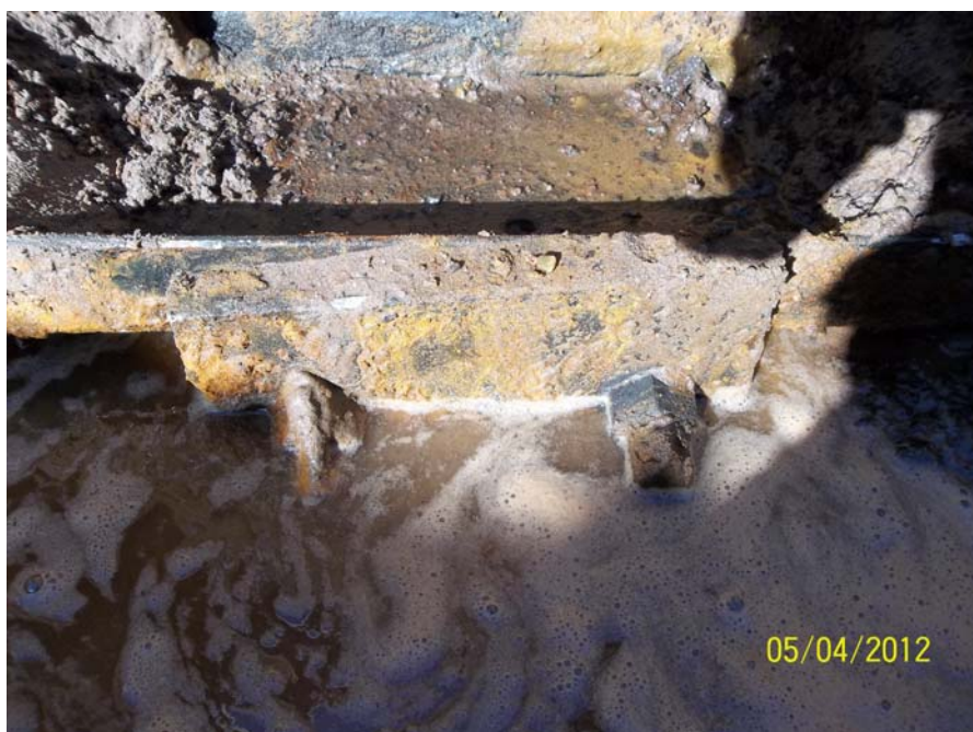
Photo 50 - TP 2 – Back plate and waler in good condition.
