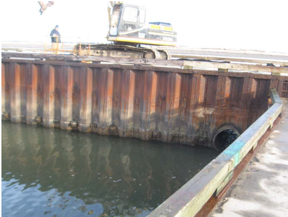
Photo No. 11: SSP Face – Harbour Side of 1968 Section of Structure 302. (2011-11-29)
