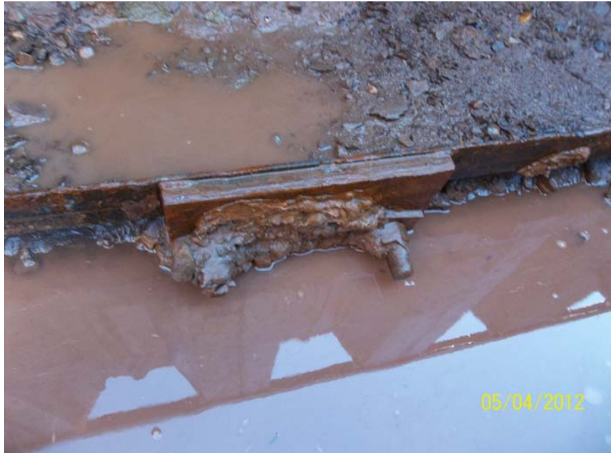
Photo 43 - TP 1 – Exposed waler and back plate.
