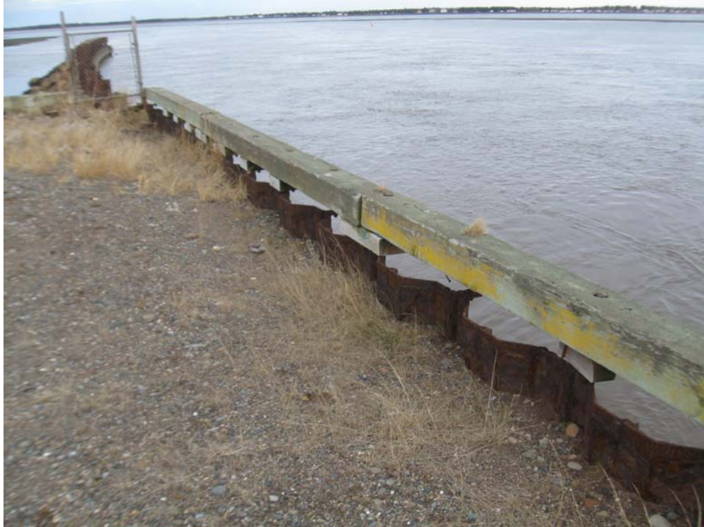
Photo No. 7: Overhanging Guard Along East Face of 1966 Section of Structure 302. (2011-11-29)
