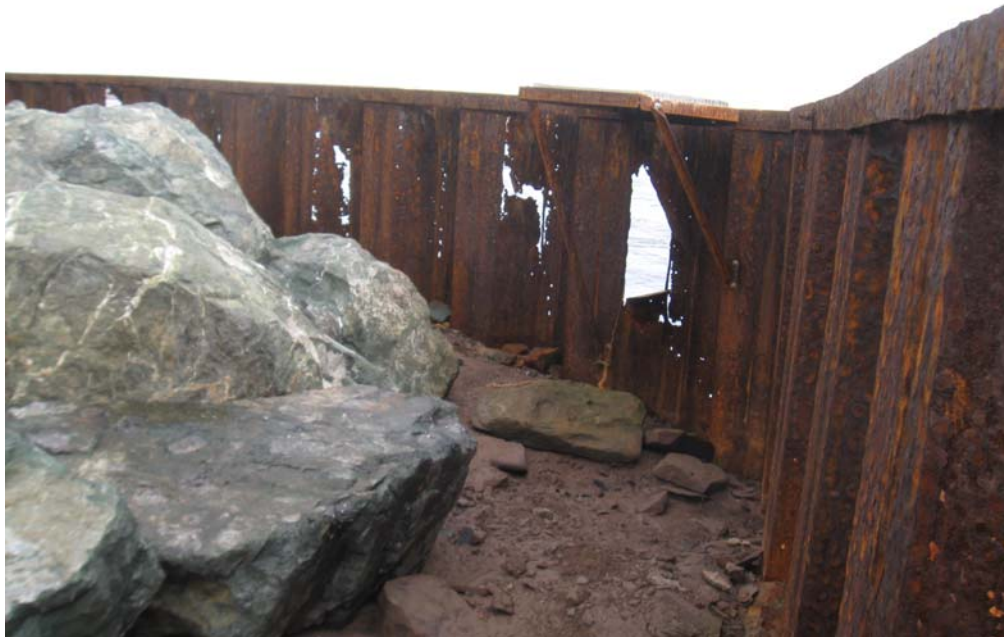
Photo No. 27: Back Face of Perforated SSP at South-East Corner of Structure 304. (2011-11-29)
