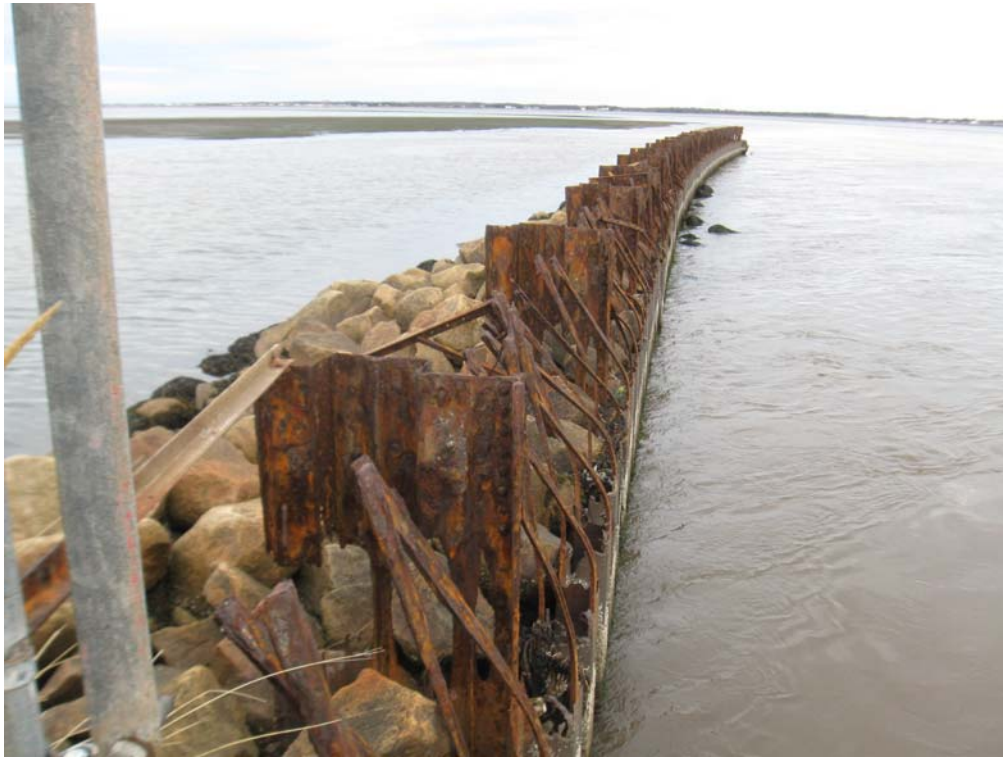
Photo No. 9: Deteriorated SSP Wall to North of Structure 302. (2011-11-29)
