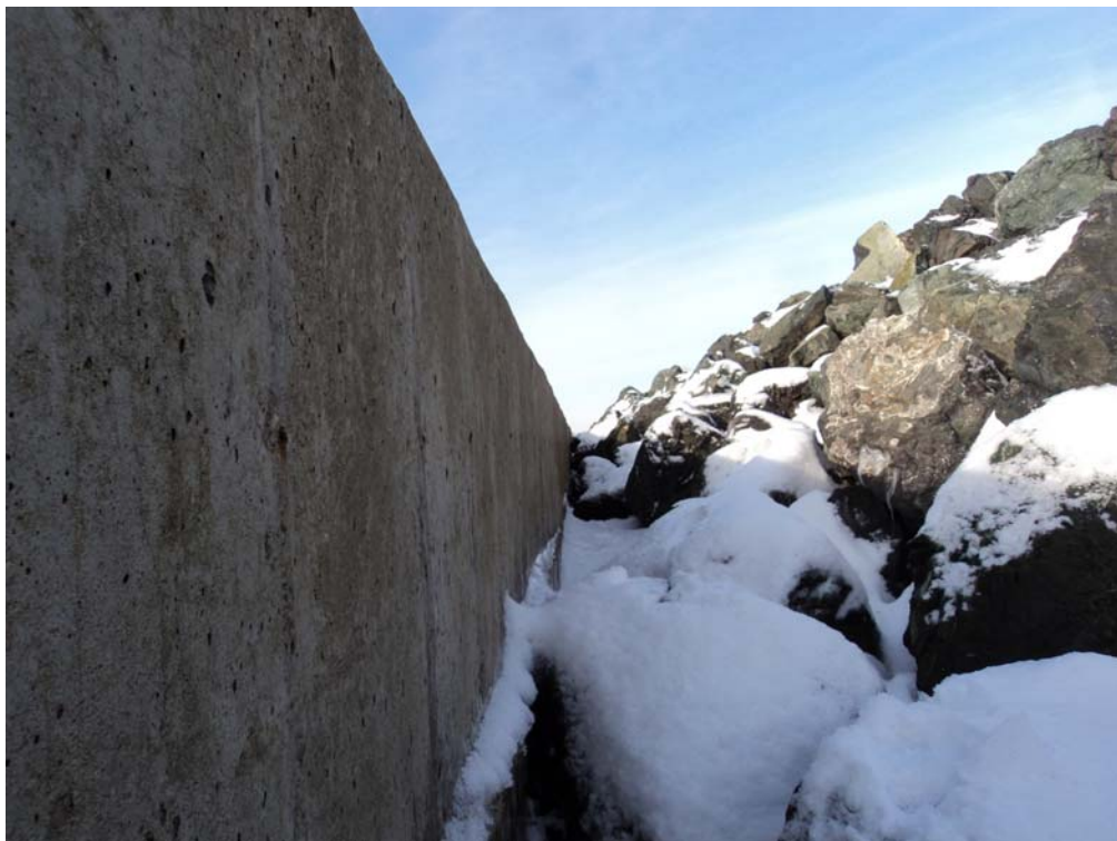
Photo No. 28: Concrete Cope Wall Along Top of South-west Face of Structure 304. (2012-02-08)
