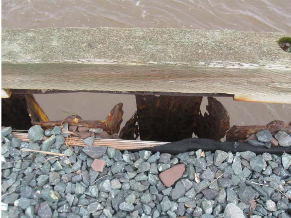
Photo No. 19: Deterioration at Top of SSP Channel Face at 1966 Section of Structure 302. (2011-11-29)
