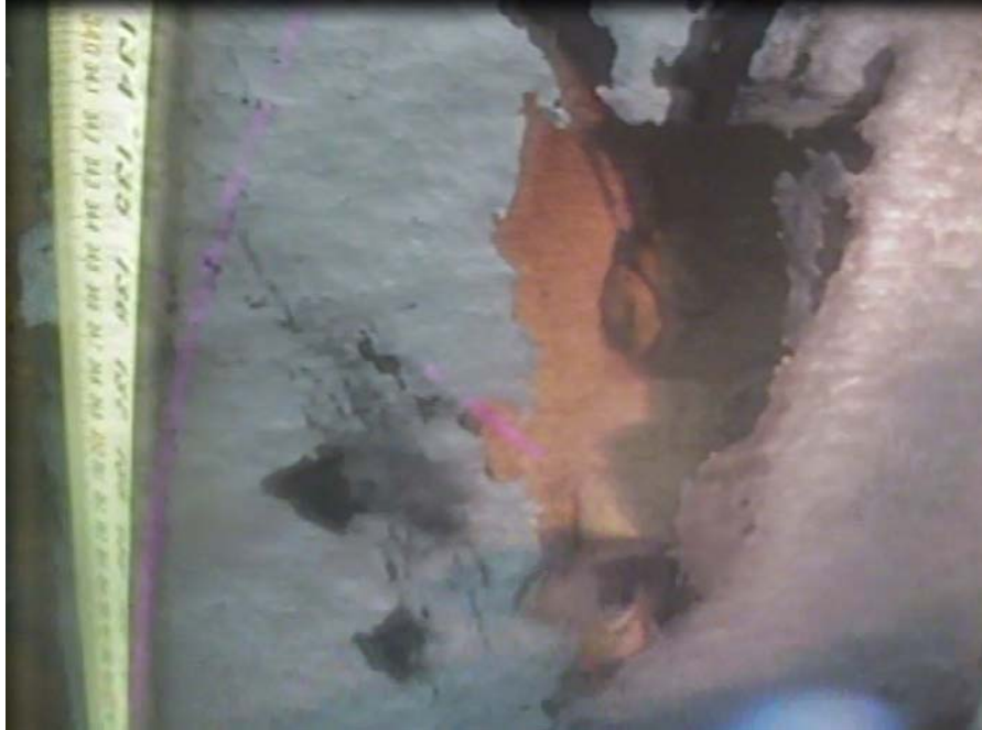
Photo 59 – Perforation in SSP within tidal zone.
