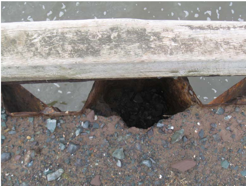
Photo No. 16: Voids In Fill at SSP Face at South End of Structure 302. (2011-11-29)
