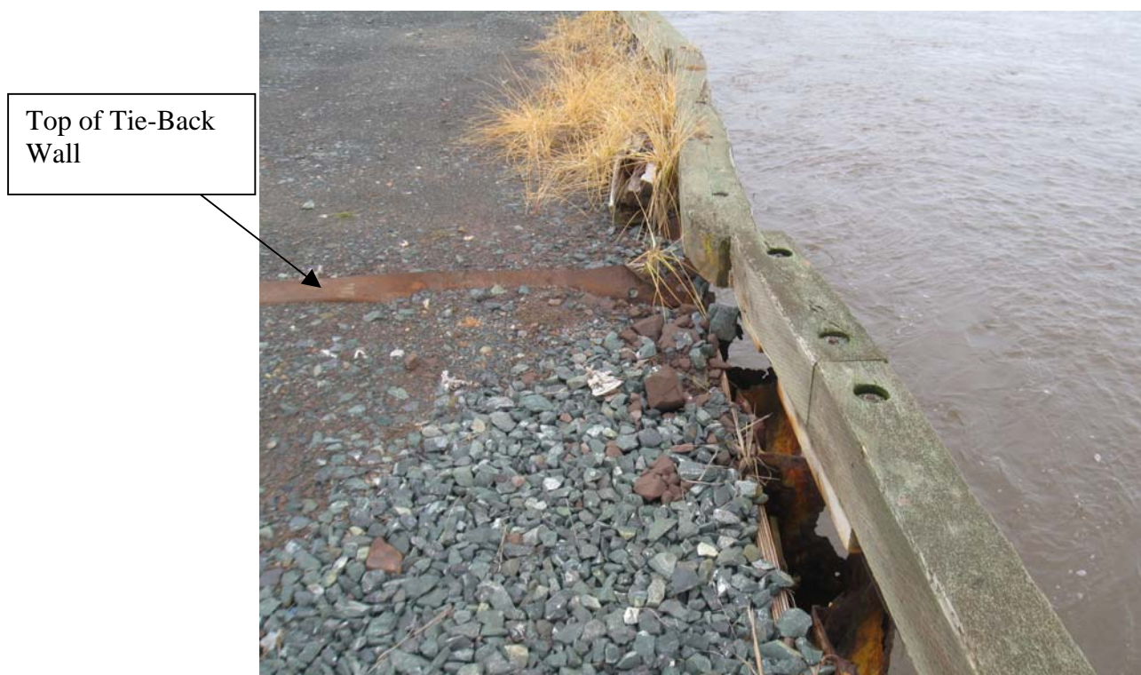
Photo No. 18 Top of Buried Tie-Back Wall at South End of 1966 Section of Structure 302. (2011-11-29)
