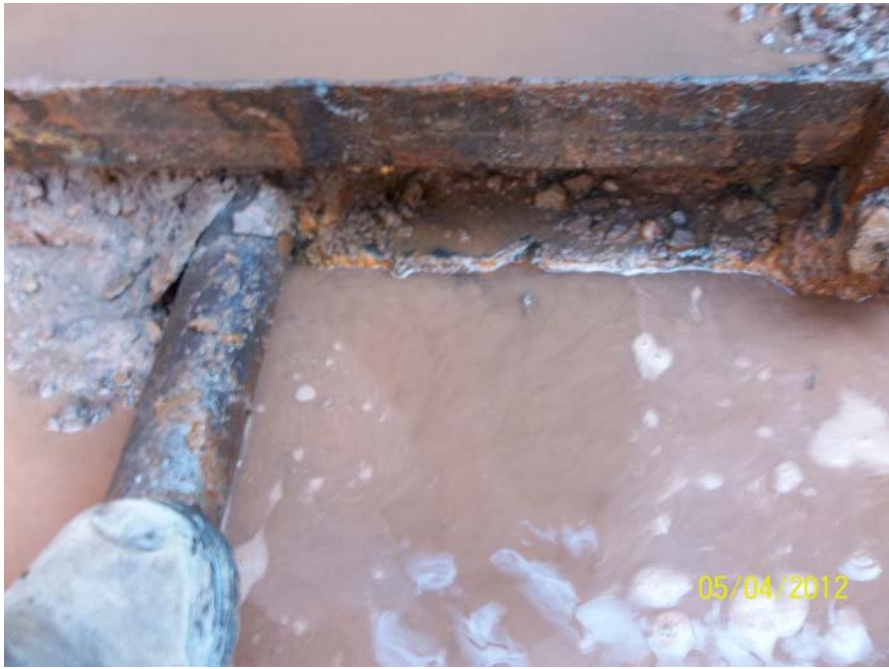
Photo 47 - TP 1 – Exposed Tie-Rod
