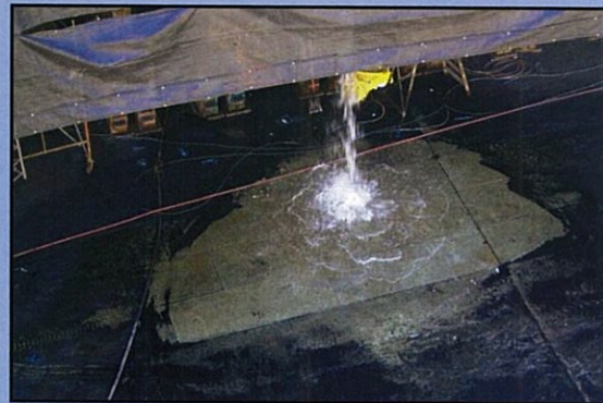
Sweep waste grit under the vessel to prevent it from being washed down the drain.
