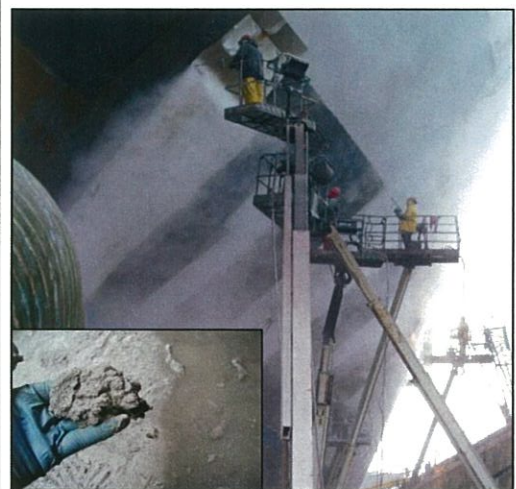
The hull of a cruise ship being ultra high pressure washed. Inset: sludge produced during ultra high pressure washing.
