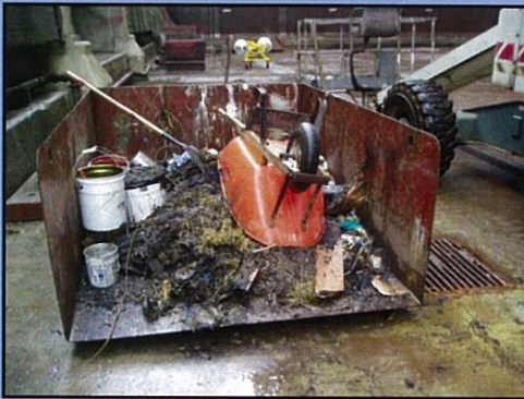
Store all waste grit away from drains, to prevent contaminated water migrating into the marine environment.
