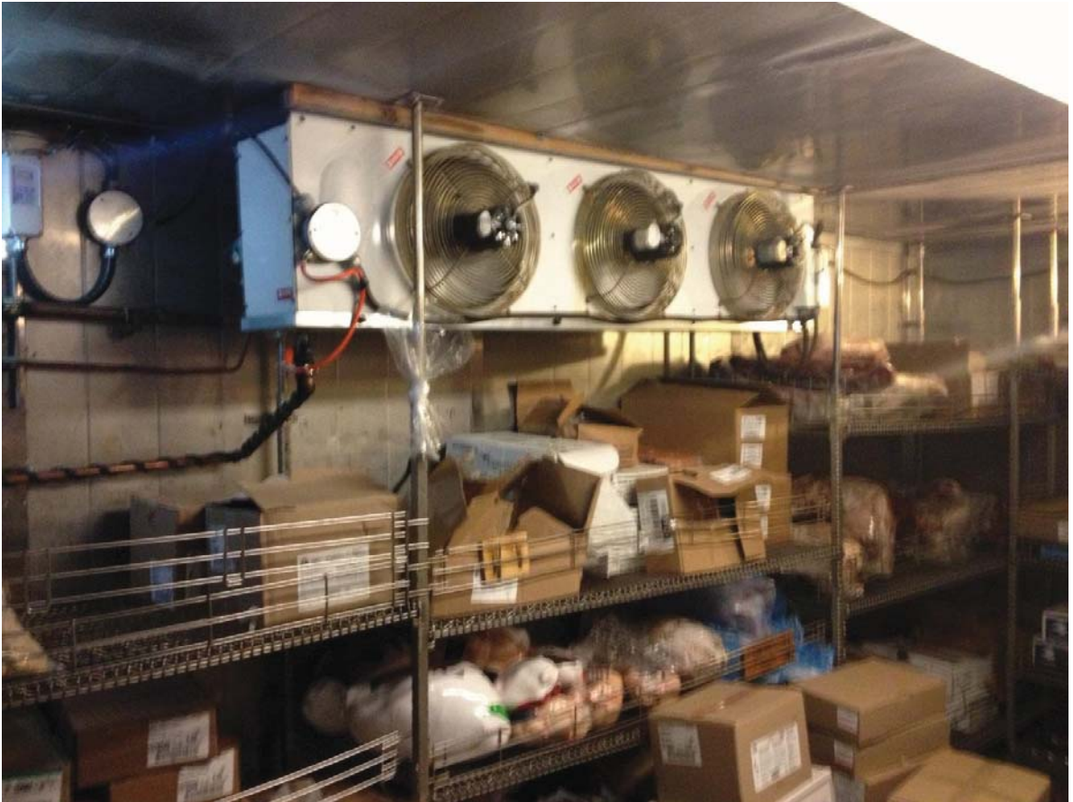
Freezer Room Evaporator Coil (To Remain)
