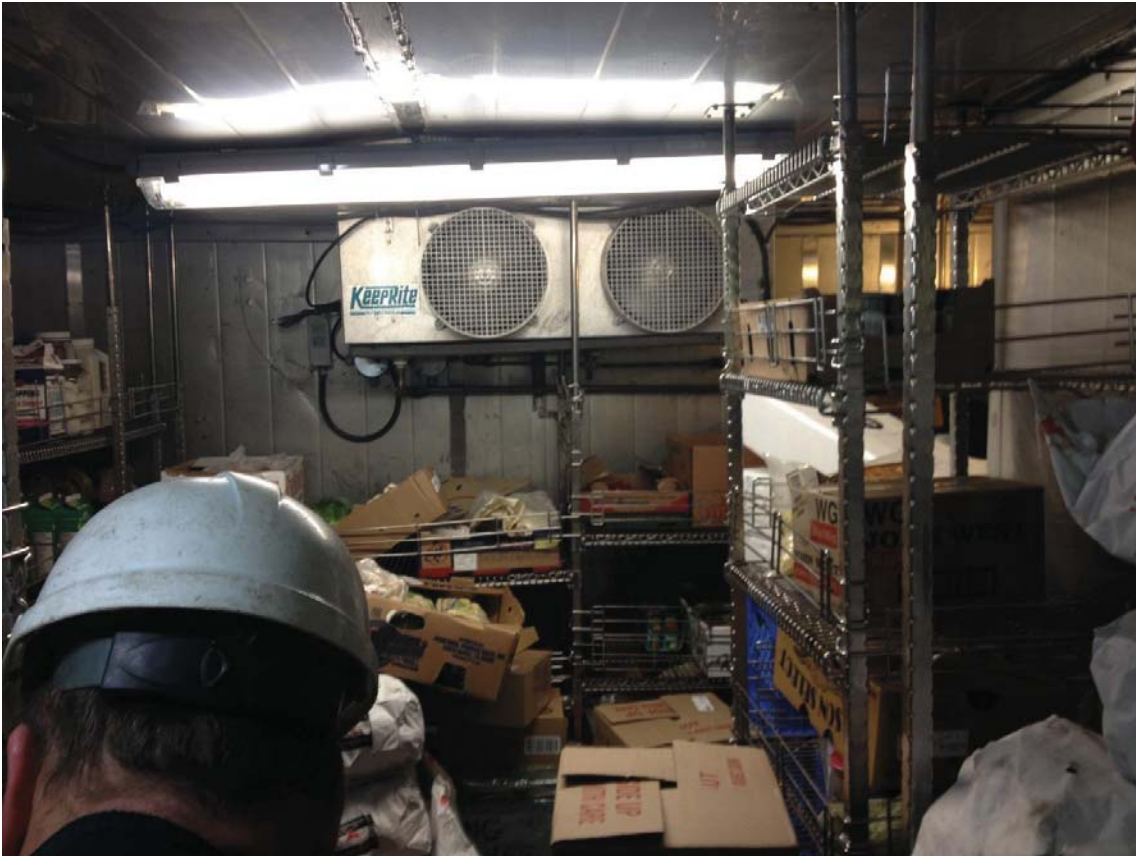
Cooler Room Evaporator Coil (To Remain)
