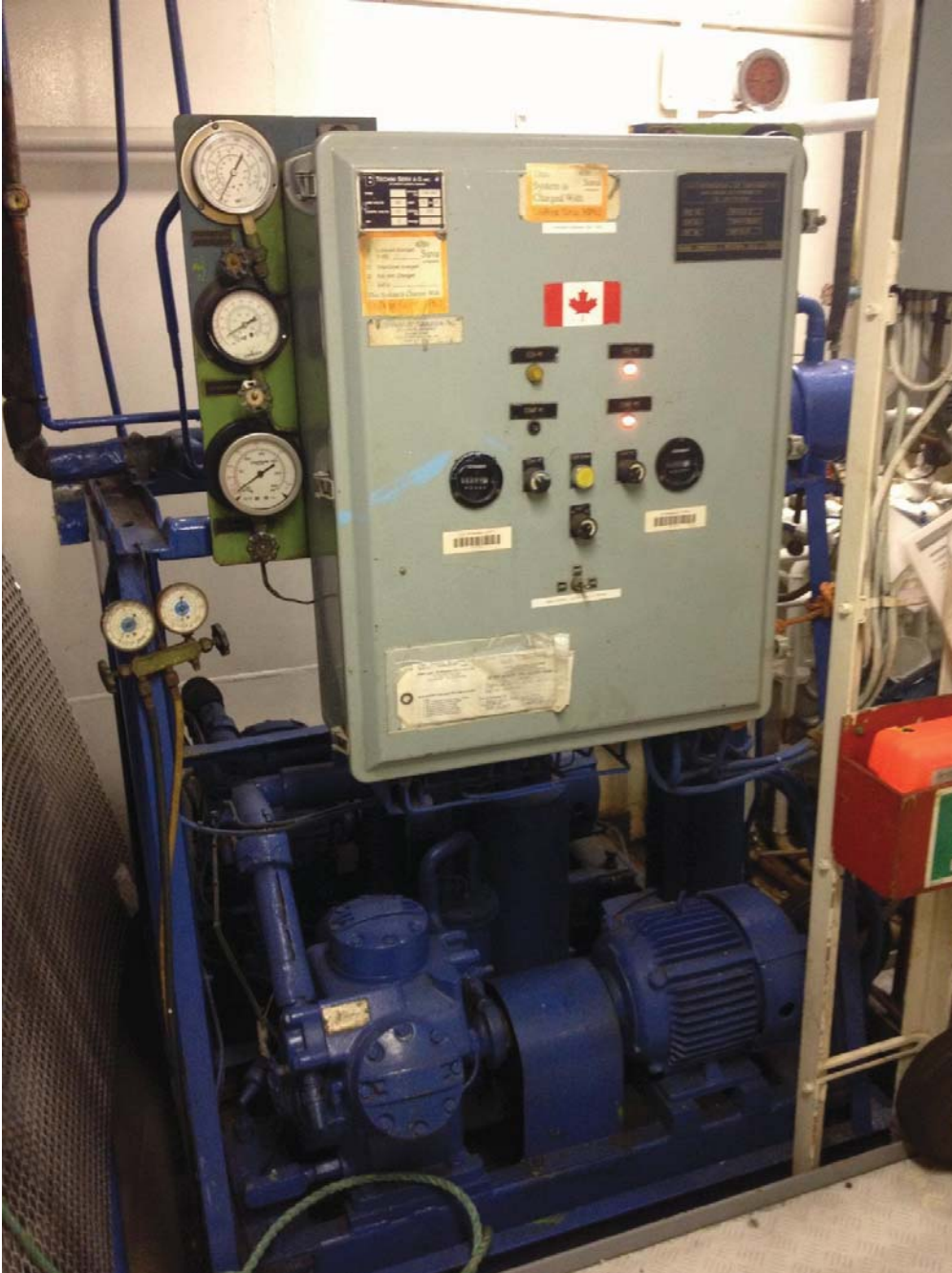
Refrigeration Package (FWD Compressor and motor to be replaced as seen in picture)
