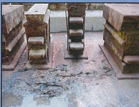
Sediment from the harbour often settles on dock bottom after dewatering. This may become contaminated with paint, etc. and must be disposed of.
