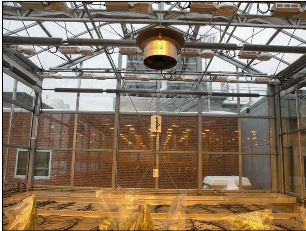
Bay 2 - North Elevation / Baie 2 - Façade Nord
