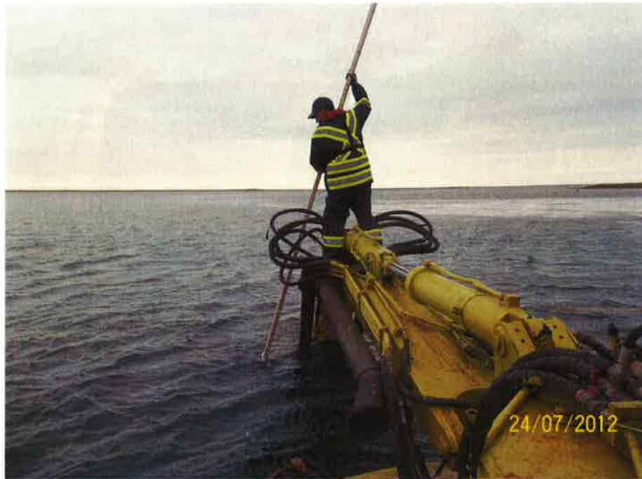
Photo 3 - Manual sounding undertaken at test pit locations.
