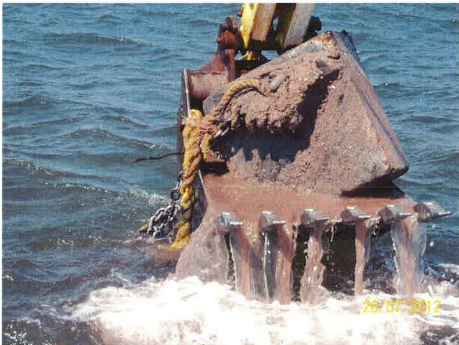
Photo 10- Concrete block with chain encountered at TP 6 - Pigeon Hill (Approximate elevation -0.61 CD). The location was marked with a buoy.
