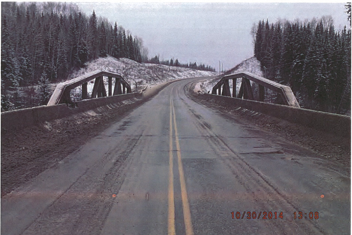
P52 - Overall Bridge - Looking South - Collision Damage to East Concrete Bridge Barrier
