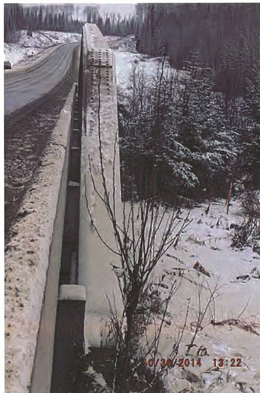
P44 - East Truss - Looking North - Straight and Plumb
