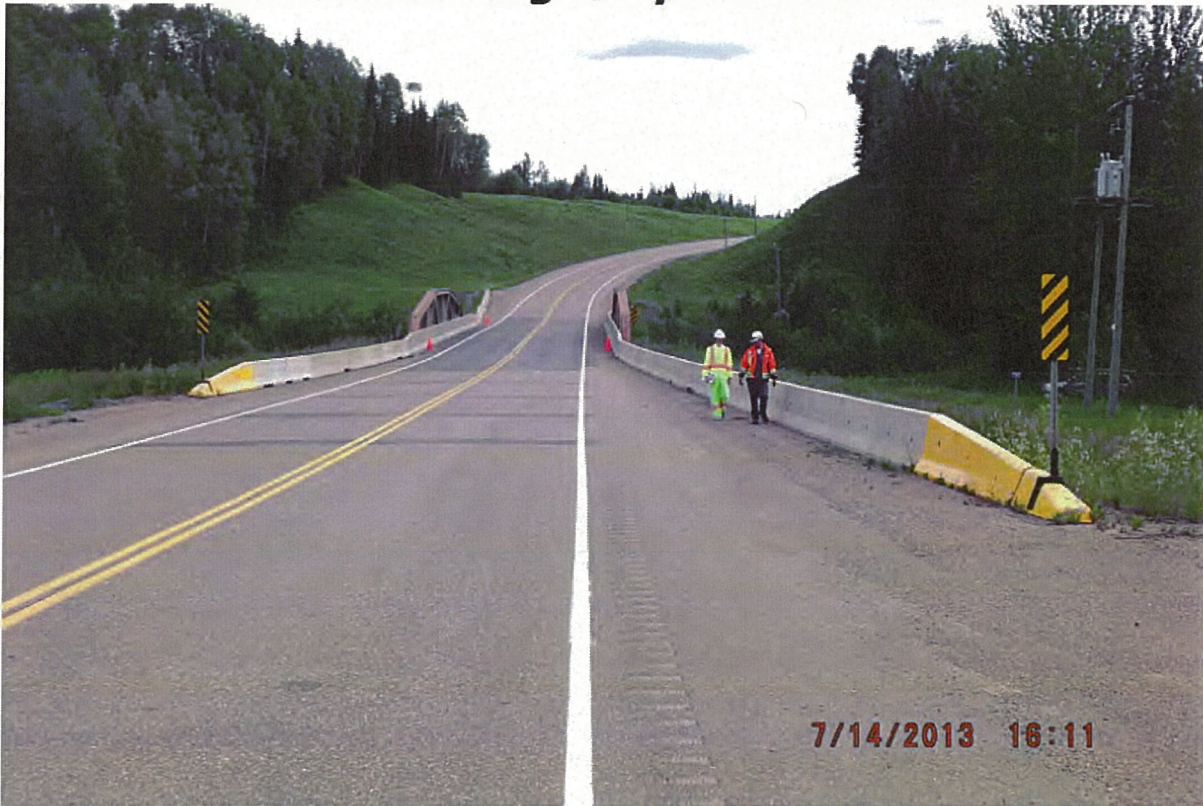
P17 - Previous July 2013 Inspection - North Approach - Both Approach Barriers Properly Aligned
