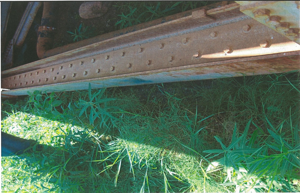
Bottom Chord of Truss
