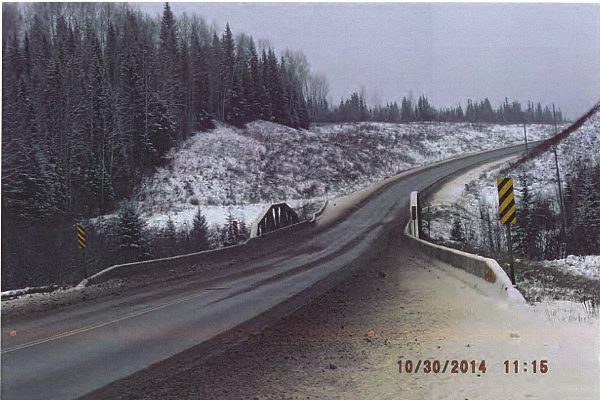
P14 - North Approach - Looking South
