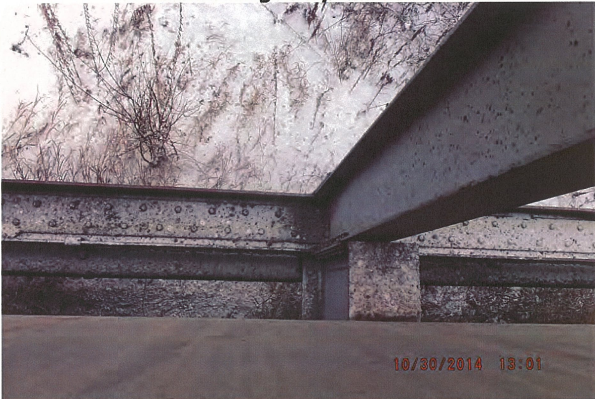
P43 - West Truss - Vertical 1 and Bottom Chord - No Collision Damage
