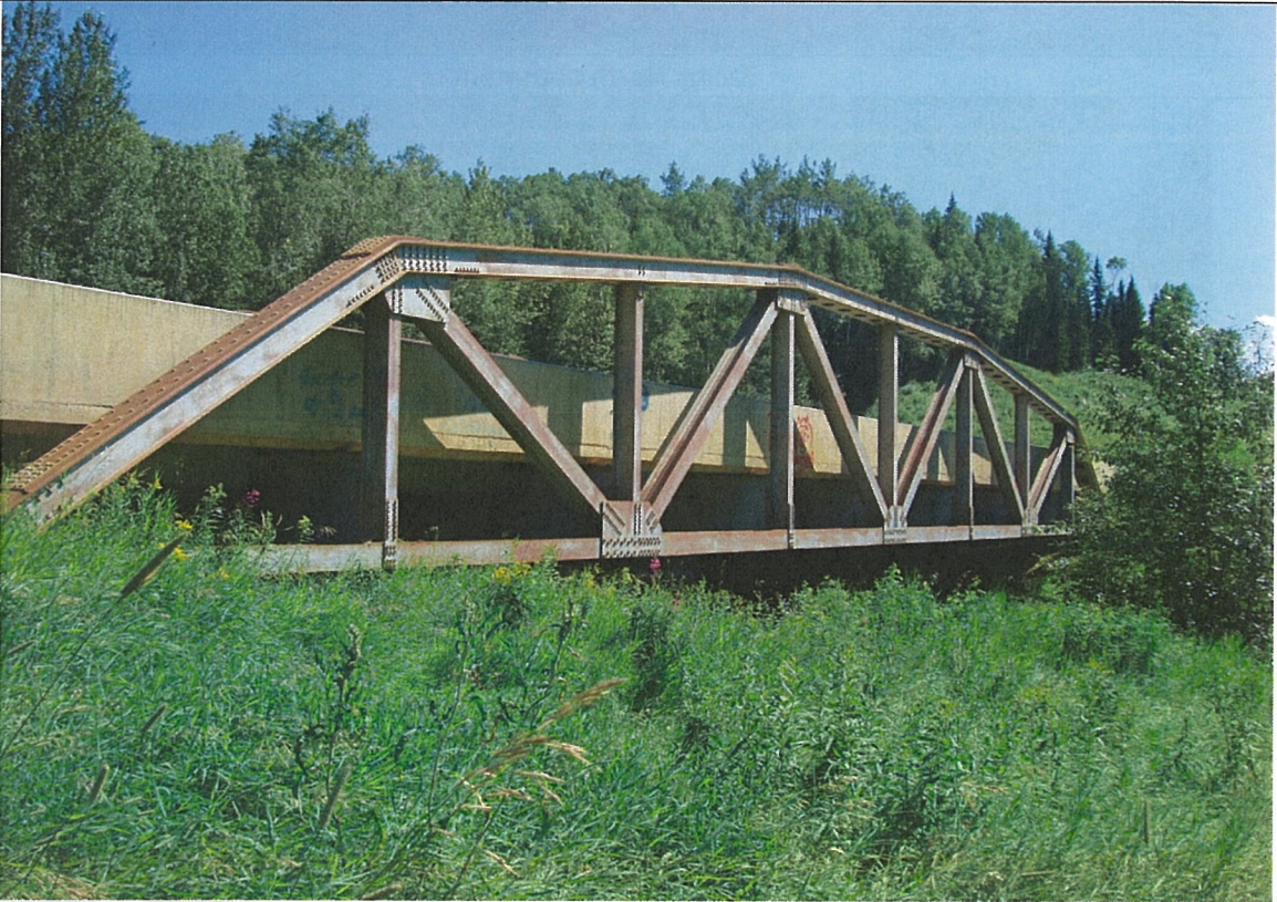
(NW) West Truss
