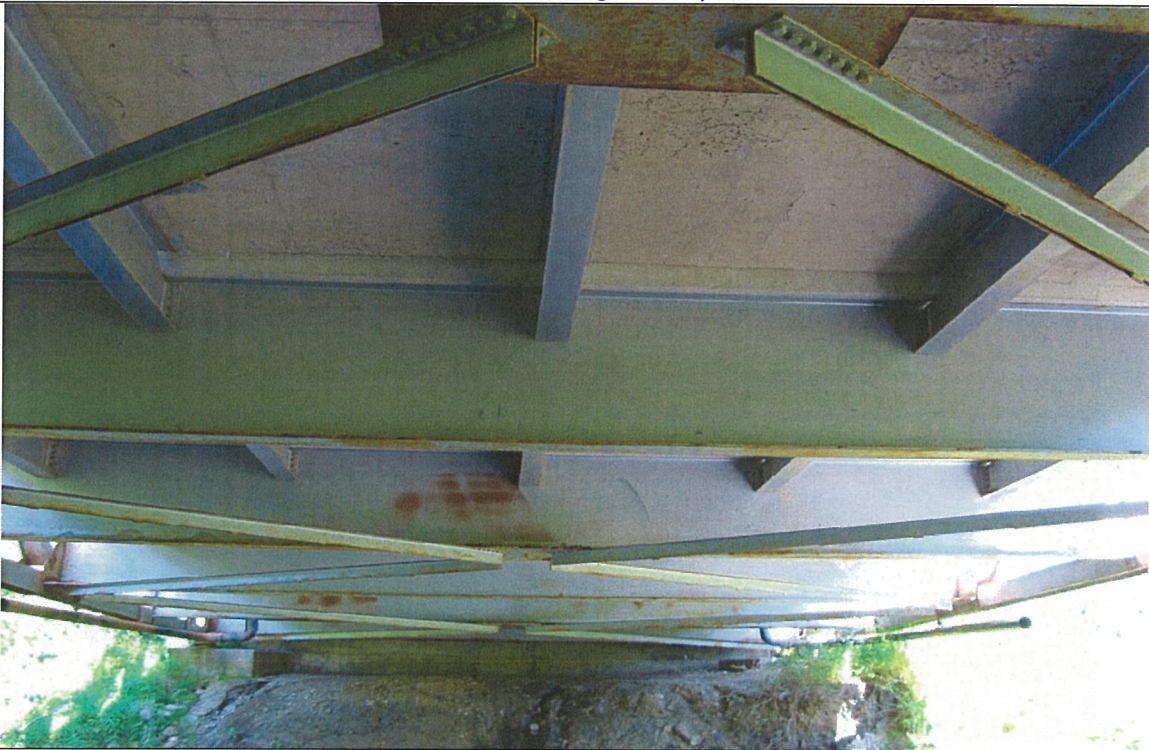
Floor Beam System (Facing north abutment)
