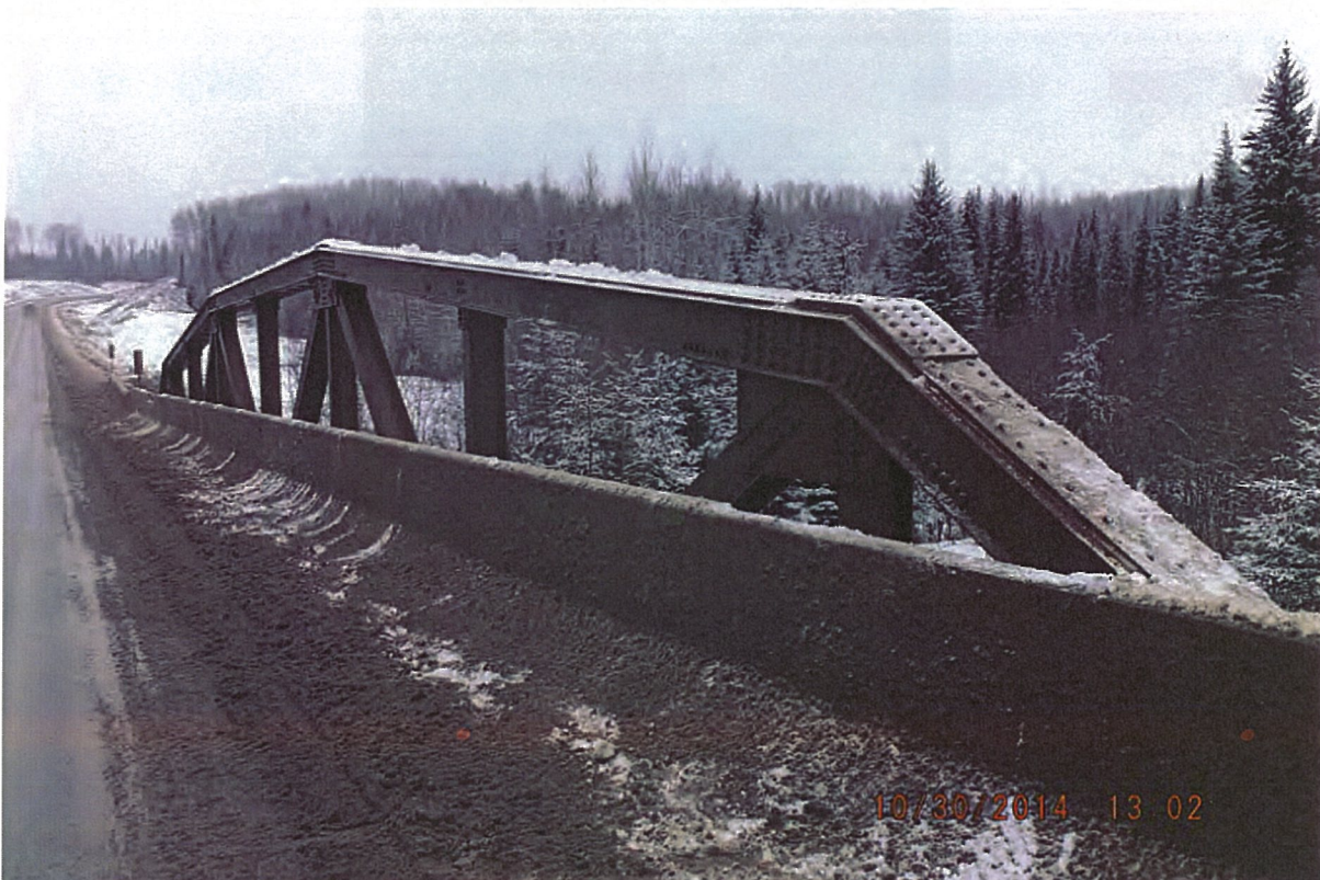
P42 - East Truss - Looking North - Straight and Plumb
