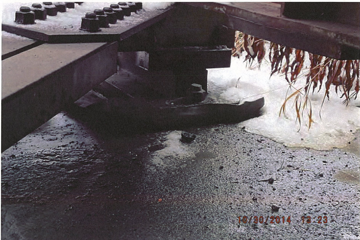
P50 - NW Bearing - Anchor Bolts in Place and Straight
