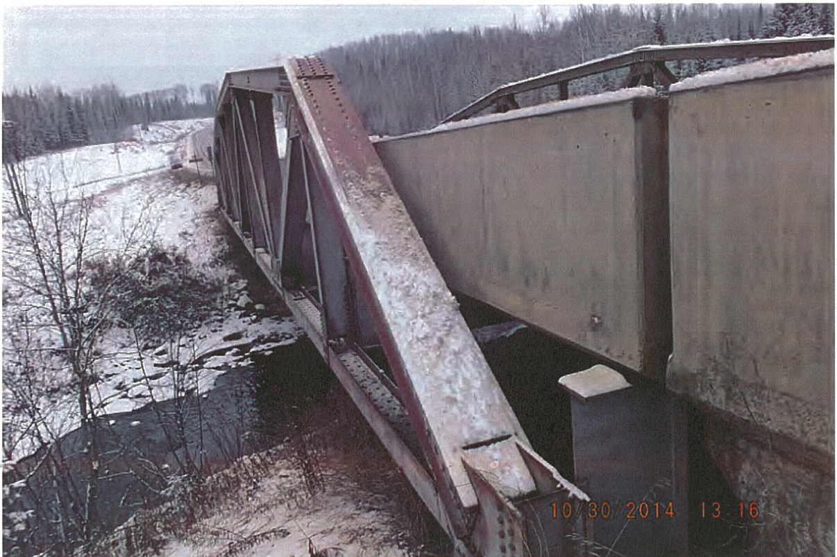
P24 - West Truss - Straight and Plumb
