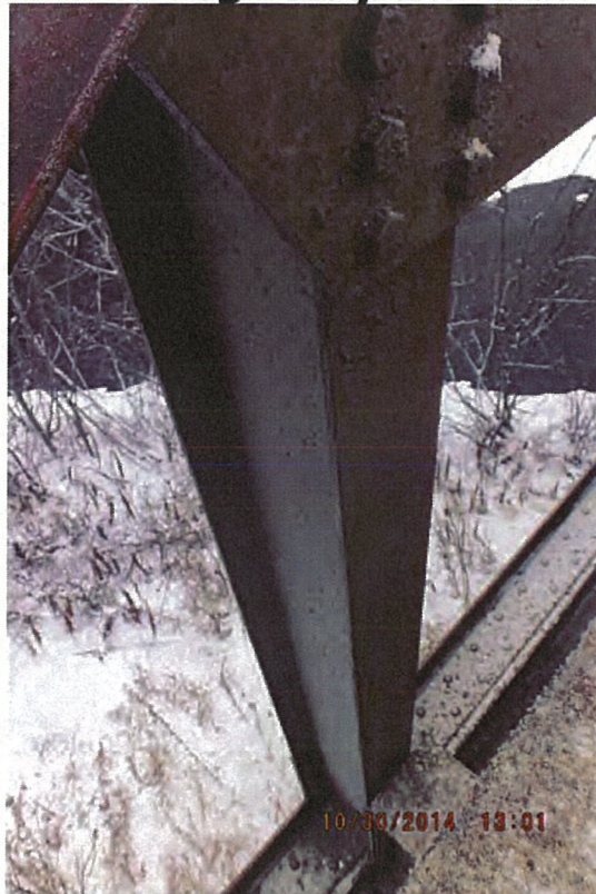
P41 - West Truss - Vertical 1 - No Collision Damage
