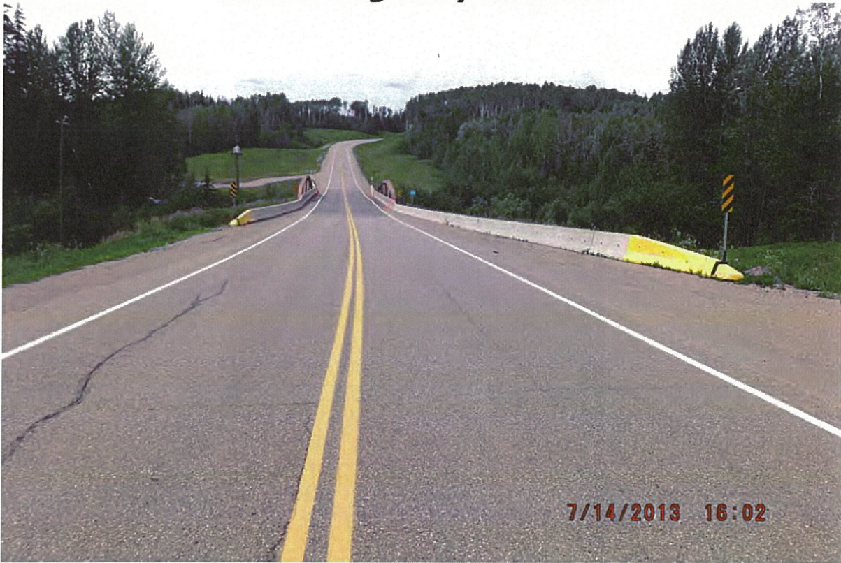
P13 - Previous July 2013 Inspection - South Approach - Both Approach Barriers Properly Aligned
