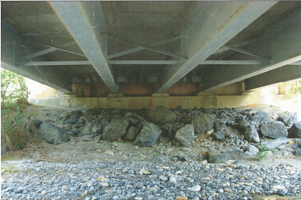
Girders (South abutment)
