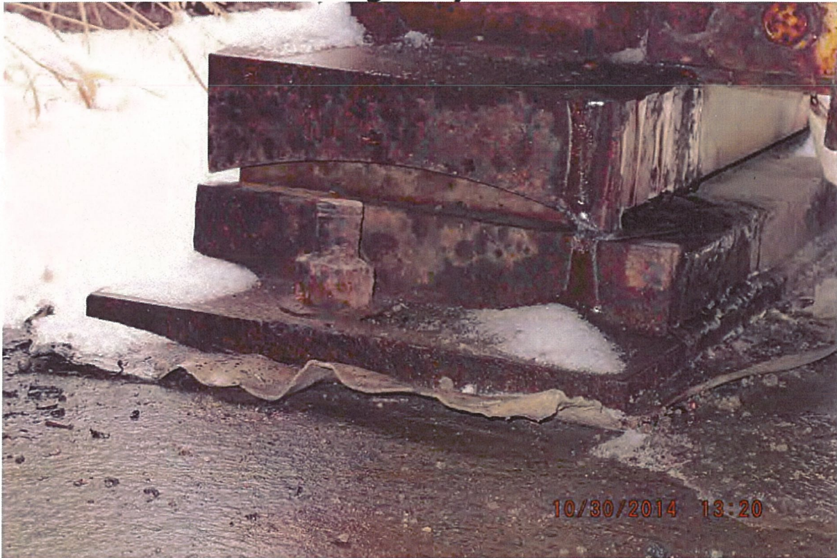
P49 - SW Bearing - Anchor Bolts in Place and Straight
