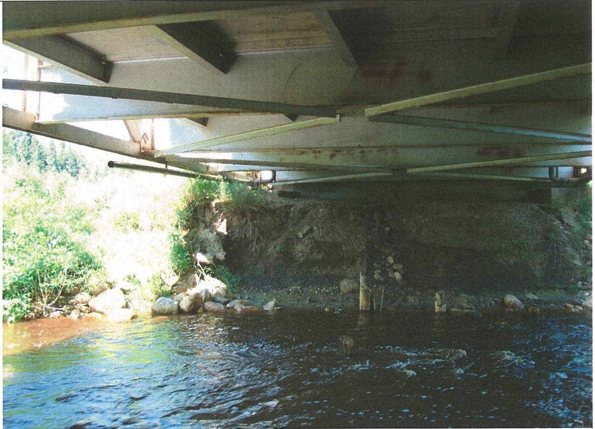
Facing North abutment
