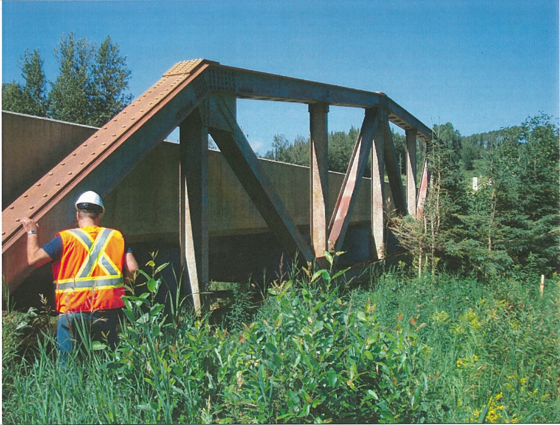
(SE Elevation) East Truss
