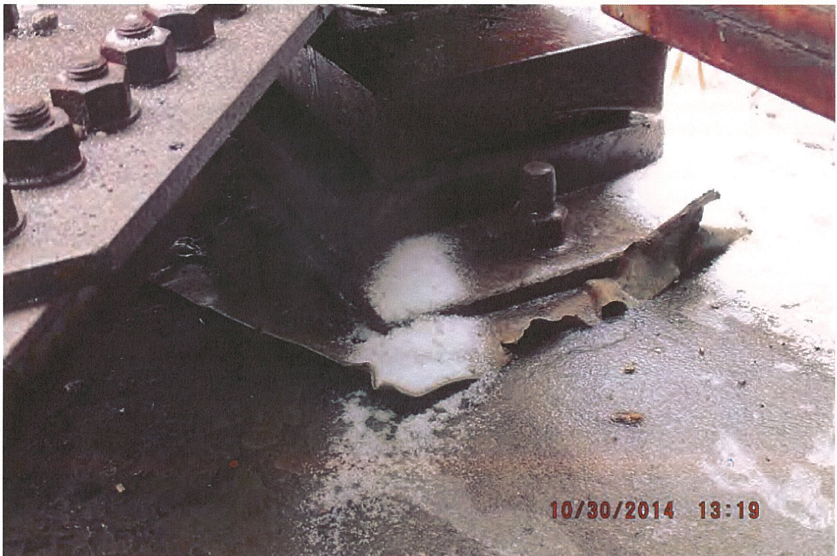
P48 - SE Bearing - Anchor Bolts in Place and Straight
