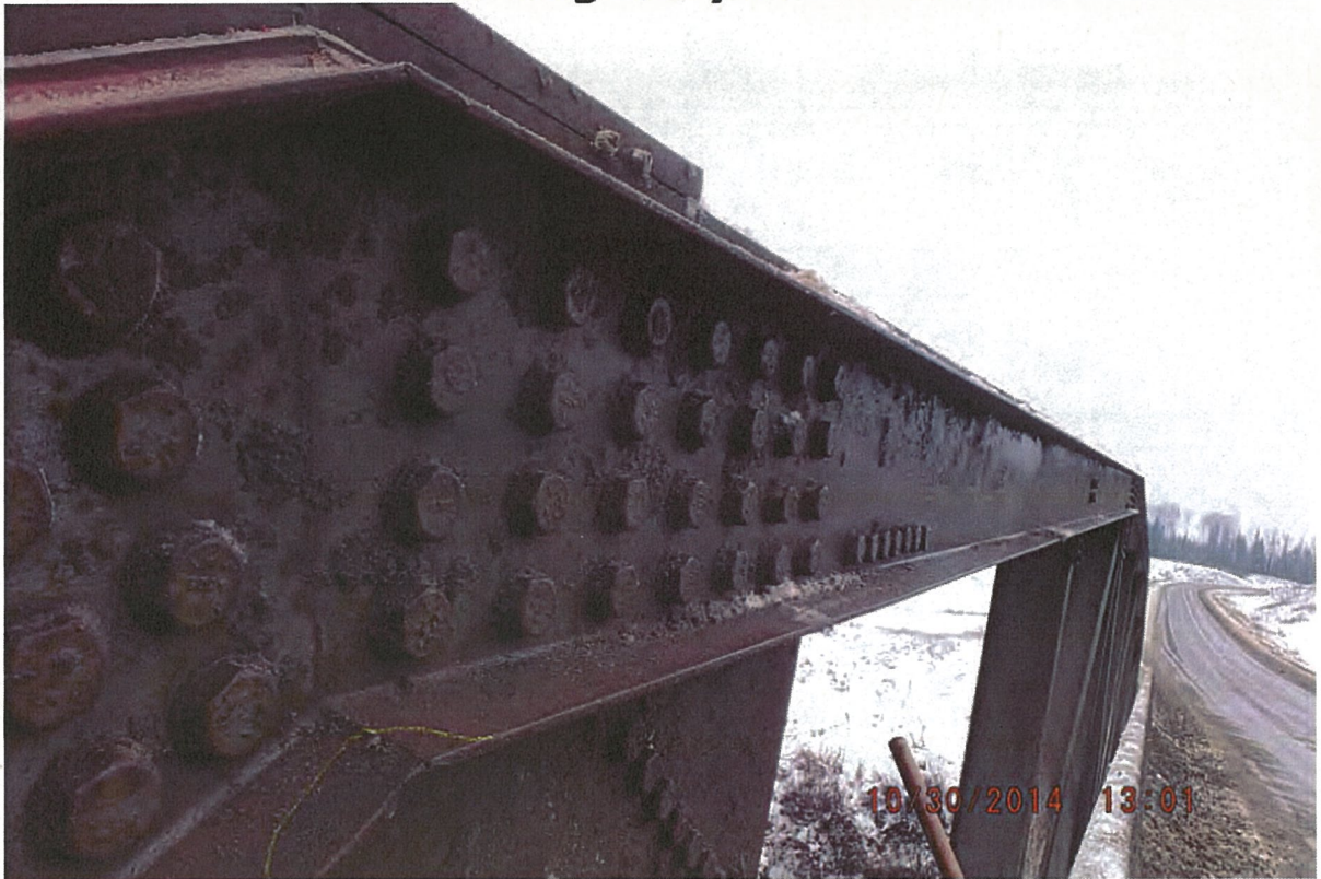
P39 - West Truss - Top Chord U1-U3 Straight
