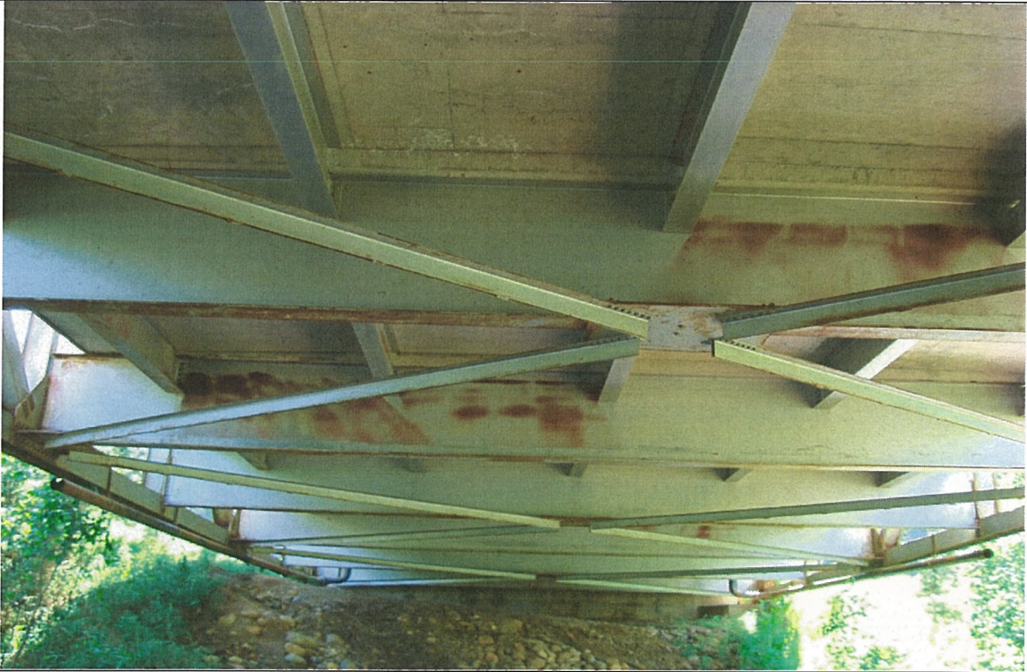
Floor Beam System Facing South Abutment
