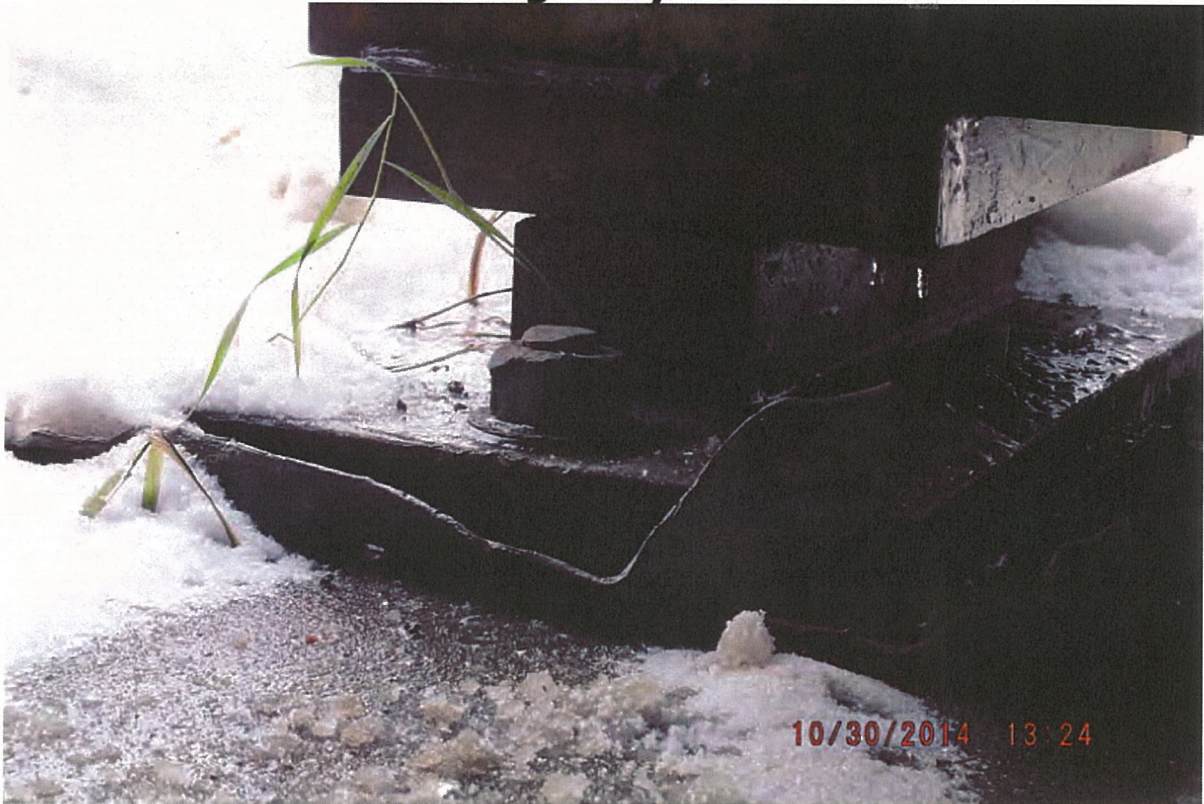
P51 - NE Bearing - Anchor Bolts in Place and Straight
