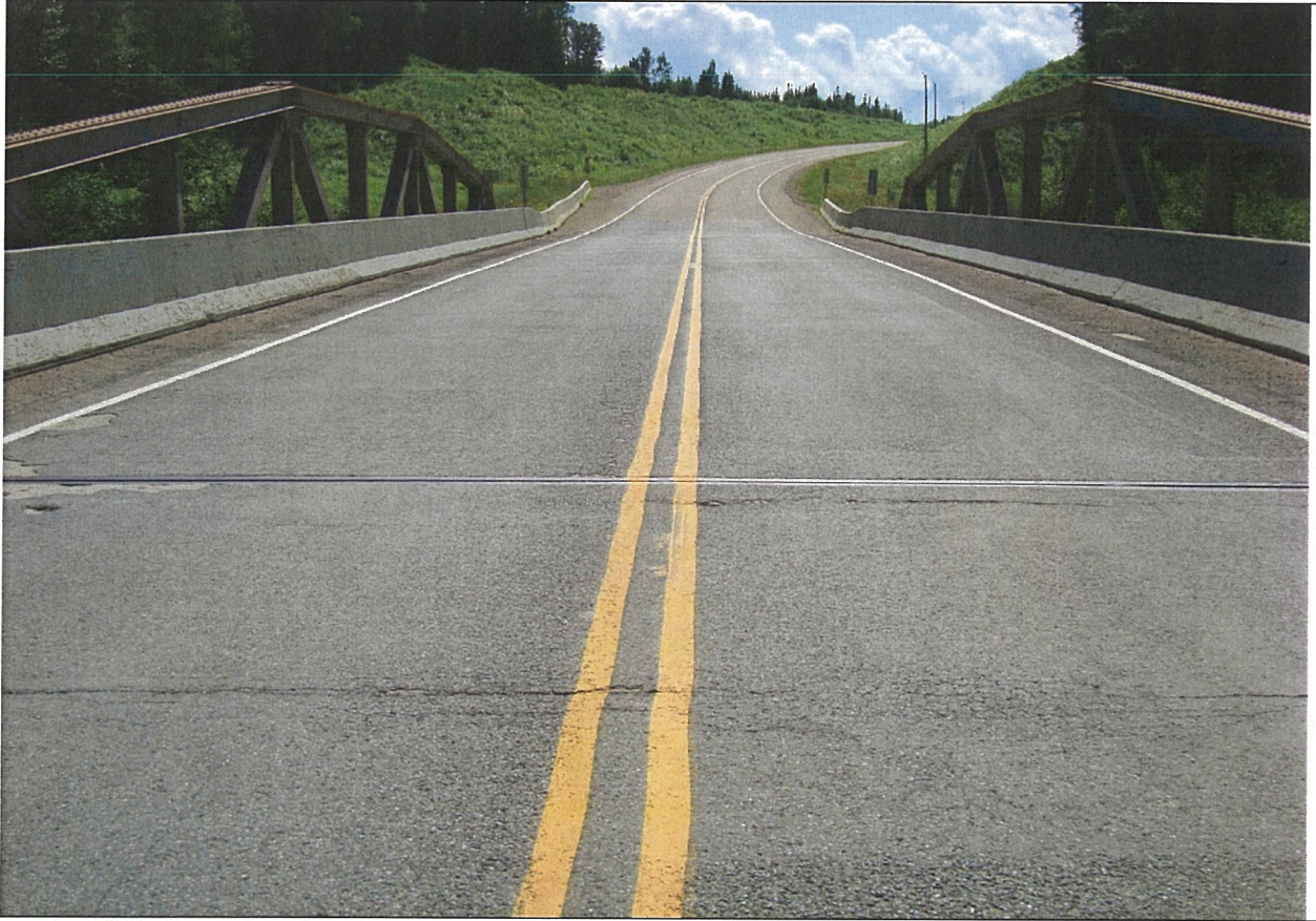
Jackfish Creek Bridge – Pony Truss
