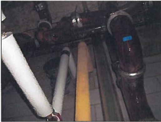
Asbestos-containing parging cement on pipe fitting, steam line, Service Core adjacent to Lab L761
