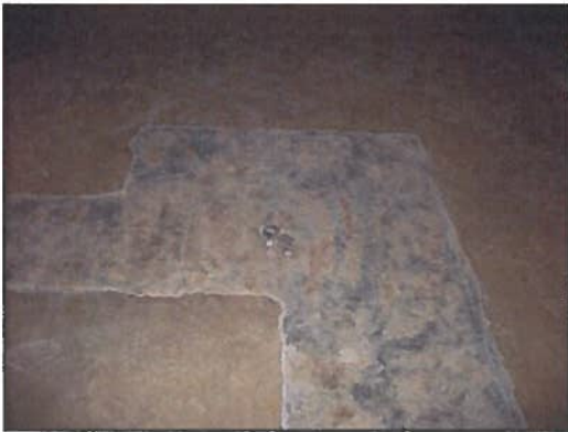
Non-asbestos vinyl floor tile mastic and poured flooring, Lab L760
