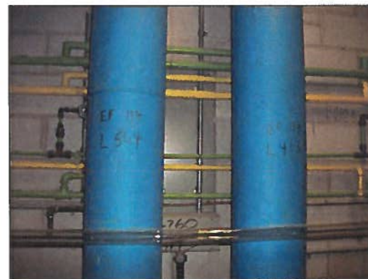
Transite exhaust ductwork, 7 th Floor Service Core
