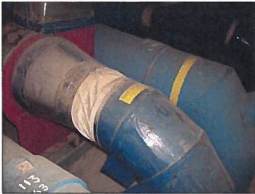
Non-asbestos black coating on metal exhaust ductwork, Mechanical Penthouse
