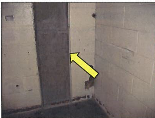
Asbestos-containing white caulking at concrete column, Lab L760
