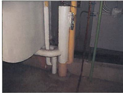
Asbestos-containing parging cement on pipe fitting, steam line at riser, across from Elevator Mechanical Room in Mechanical Penthouse
