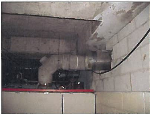
Mercury may be present in south-east metal exhaust ducting, Lab L760
