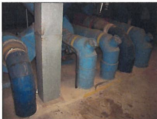
Transite exhaust ductwork, Renovation Area of Penthouse
