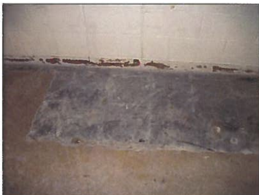
Non-asbestos baseboard mastic on wall, Lab L760
