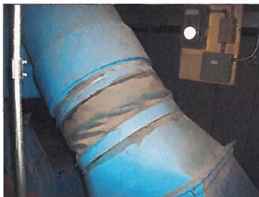
Non-asbestos rubber vibration damper, Mechanical Penthouse
