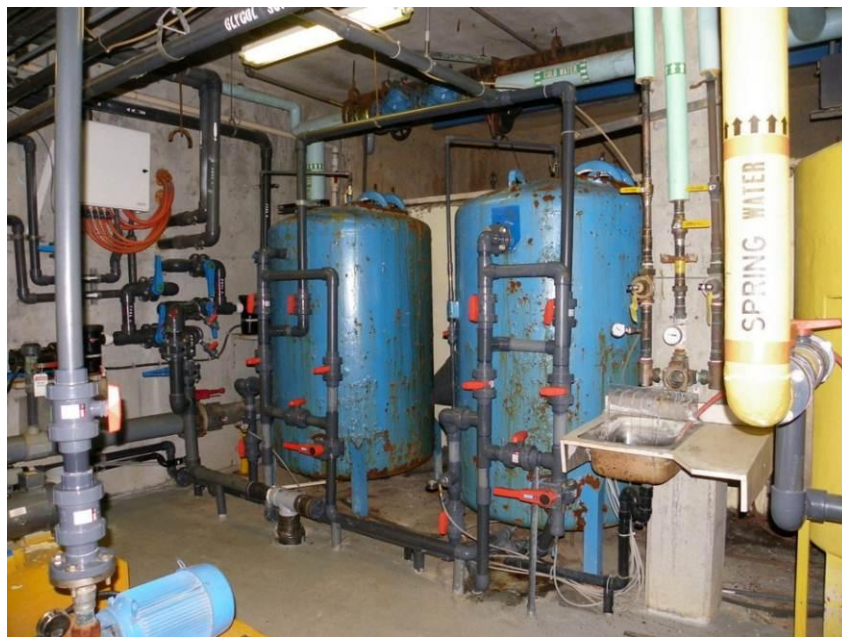
Image showing existing rapid sand filter system.
