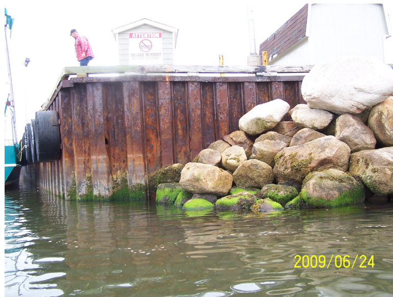
Photo 9 - Steel Sheet Pile Wall (Station 29.5)
