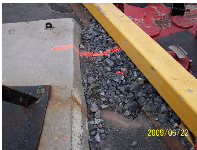
Photo 20 - Wharf 404 Loss of Fill Materials (Station 12.5)
