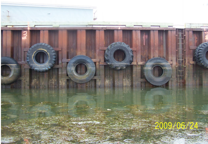
Photo 15 - Steel Sheet Pile Wall Wharf 403 (Stations 2 to 3)
