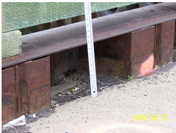
Photo 13 - Wharf Deck Subsidence (Station 8)
