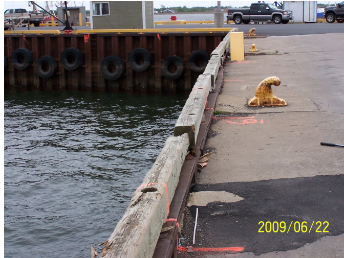
Photo 14 - Outward Bowing SSP Wall (Stations 6.5 to 7.5)
