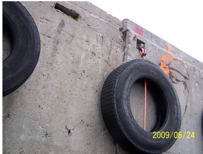
Photo 24 - Wharf 402 Cope Wall Misalignment (Station 6.1)
