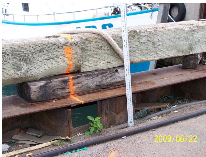
Photo 1 - Wharf Deck Subsidence (Station 1)
