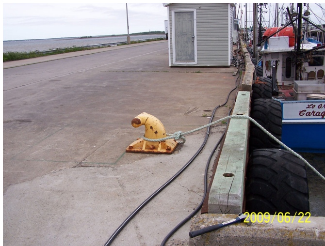
Photo 3 - Outward Bowing SSP Wall (Station 1)
