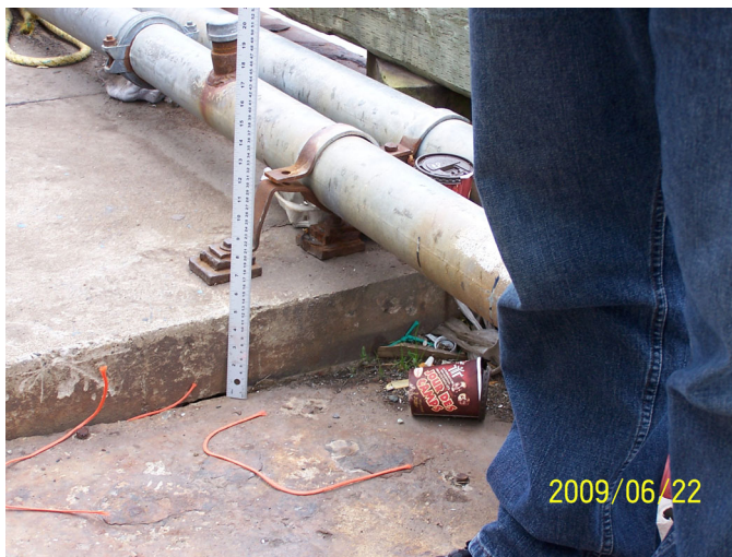
Photo 2 - Wharf Deck Subsidence (Station 5.5)
