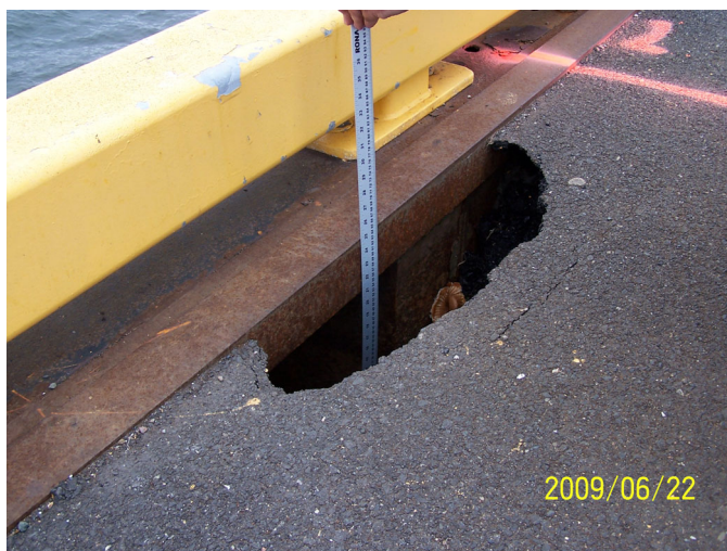
Photo 19 - Wharf 404 Loss of Fill Materials (Station 9.5)
