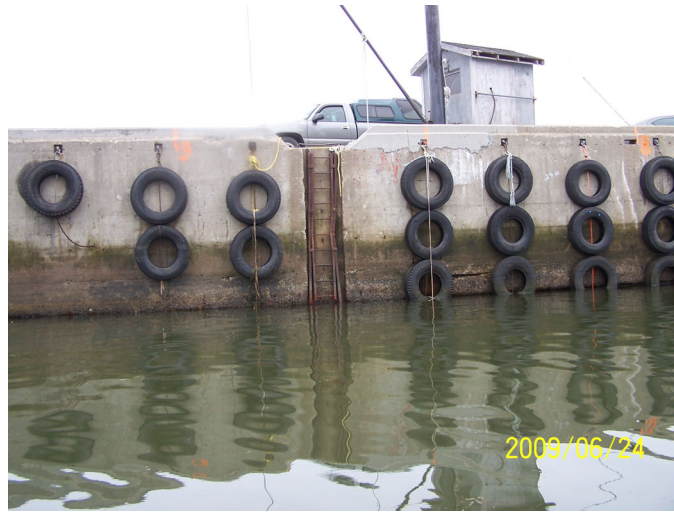
Photo 23 - Wharf 402 Concrete Deterioration at "Cold Joint" (Station 8.5)
