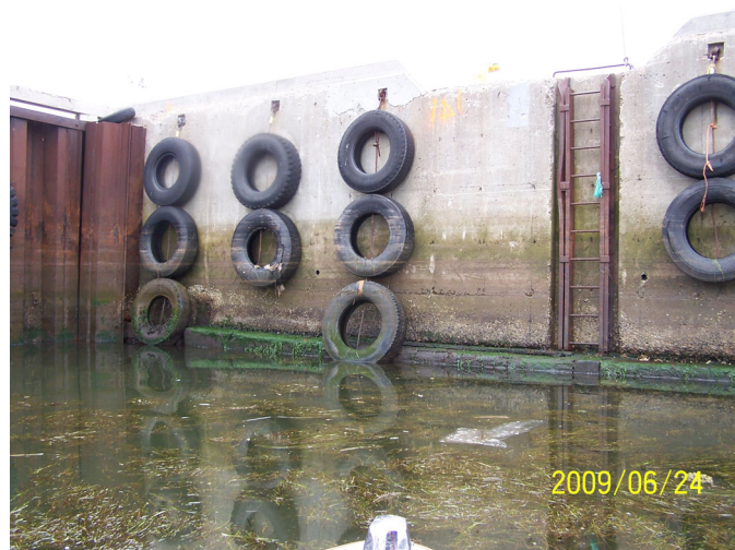
Photo 25 - Wharf 402 Projection of Cribwork Beyond Cope Wall (Station 14)
