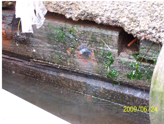
Photo 26 - Wharf 402 Timber Cribwork (Station 3.5)
