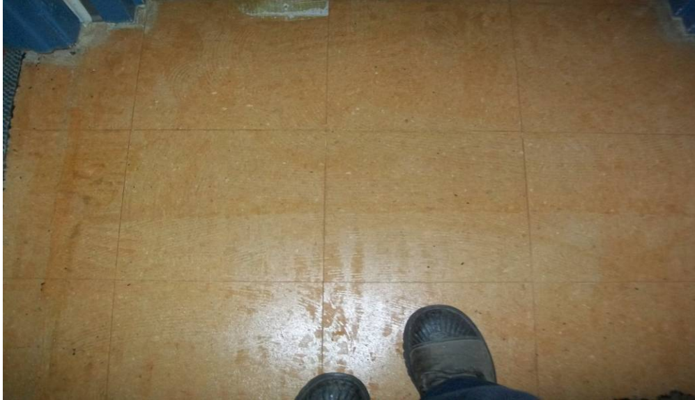
Photograph 11: View of typical assumed asbestos-containing vinyl floor tiles (“VFTs”) under carpeting along floor of west wing of building.
