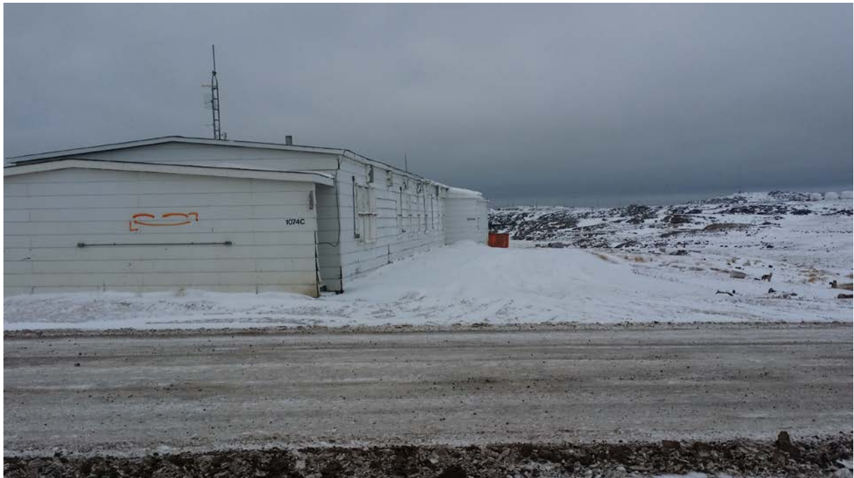
Photograph No. 4: View south along the west wing. Lead-containing paint (white) applied to the wall paneling, window frames, fascia and soffits.
