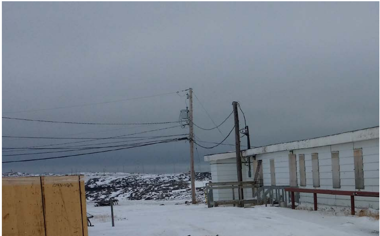
Photograph No. 2: View of the hydro-pole near the south east corner of the building. Note the pole mounted transformer.
