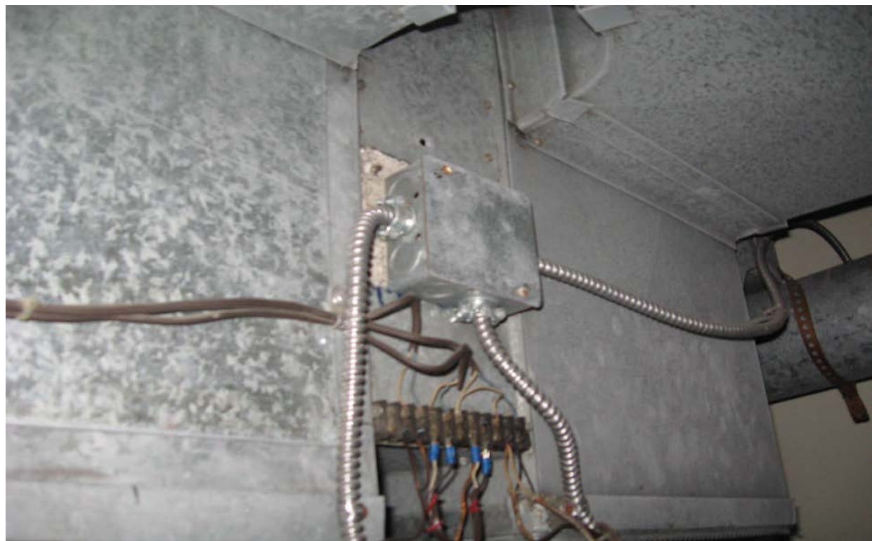
Photograph No. 6: Asbestos-containing gasket on forced-air furnace electrical junction box.
