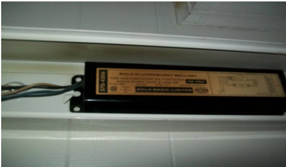
Photograph 10: View of assumed PCB-containing fluorescent lamp ballast along upper wall of washroom along west wing of building.
