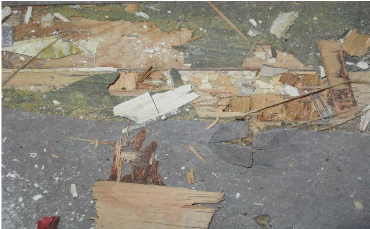
Photograph No. 5: Vinyl sheet floor flooring with asbestos-containing paper backing located under existing non-asbestos sheet flooring and plywood.
