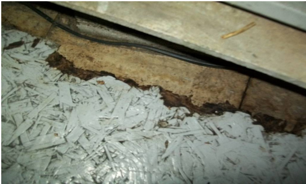
Photograph 12: View of additional typical assumed asbestos-containing VFTs under wood and other flooring material of building.
