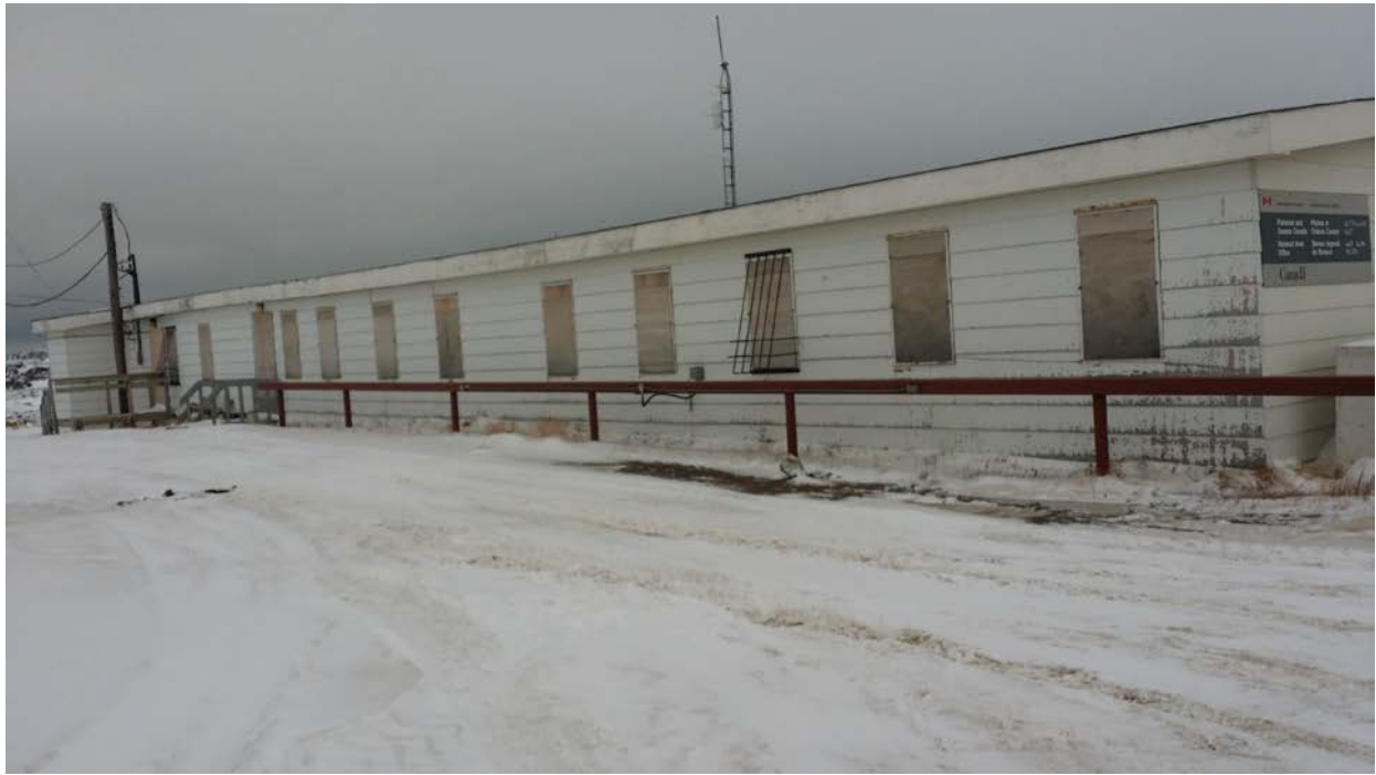
Photograph No. 1: View south along the east wing. Lead-containing paint (white) applied to the wall paneling, window frames, fascia and soffits.
