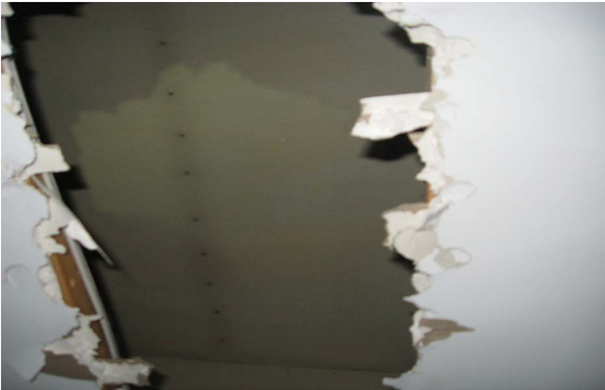
Photograph No. 7: Lead-containing paint (green) applied to underside of the roof sheeting.
