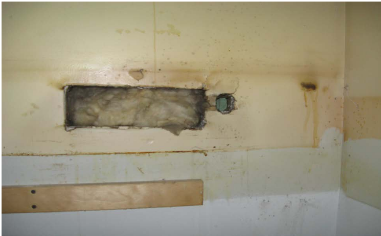
Photograph No. 8: Lead-containing paint (green) applied to the inside face of the exterior wood sheeting.
