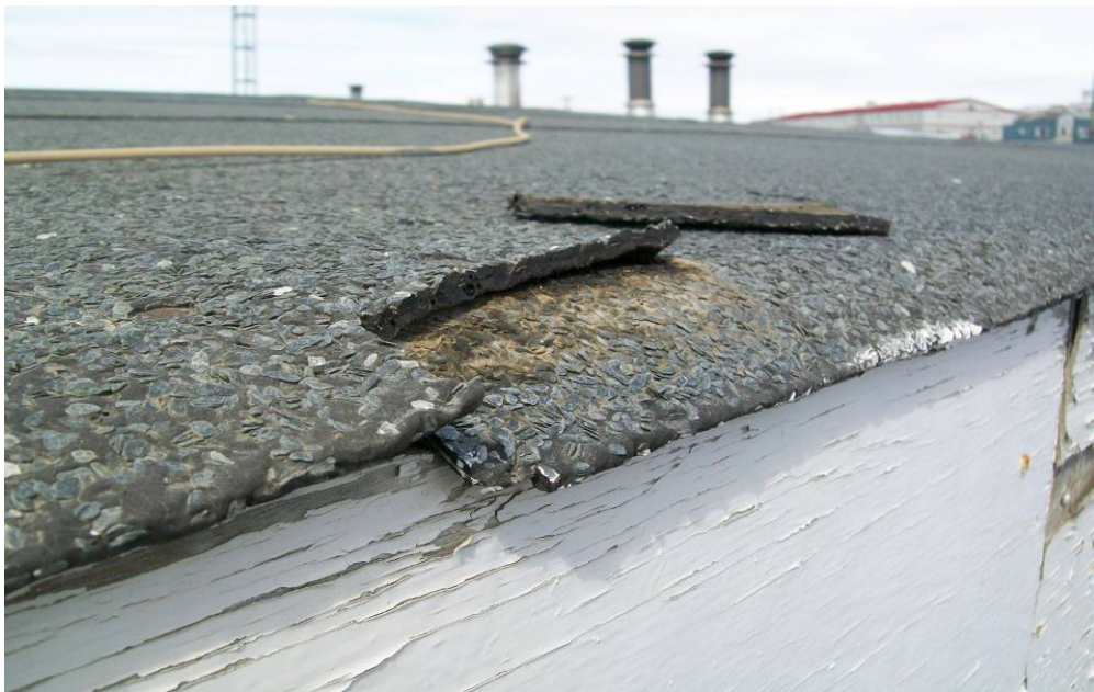
Photograph 2: View of asbestos-containing asphalt roof shingles on building. Sample (RF-01c) contained 3% Chrysotile asbestos.
