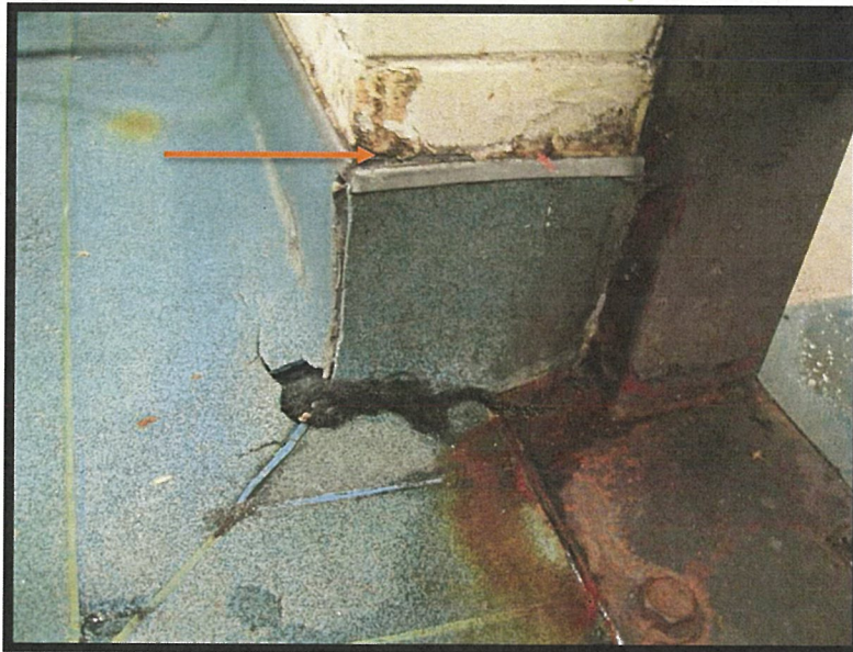
Photo #4 – Illustration of suspect visible mould identified on cinder block walls.
