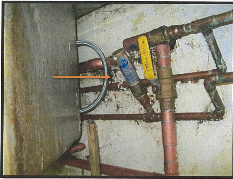
Photo #3 – Illustration of suspect visible mould identified on cinder block walls.
