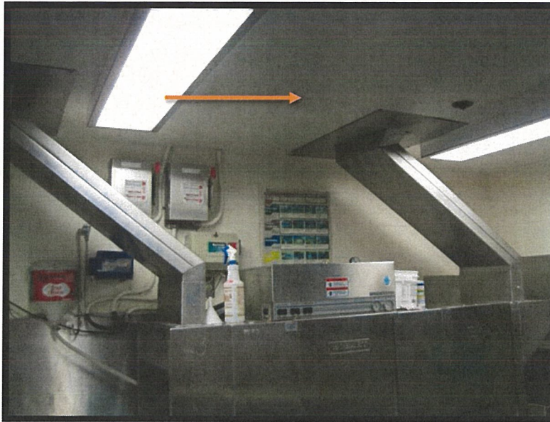
Photo #1 – Illustration of identified asbestos-containing drywall joint compound ceiling.
