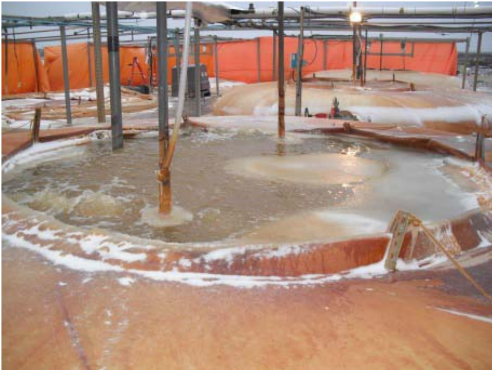
Figure 12: Plant Winterizing Phase – Tanks Freezing
