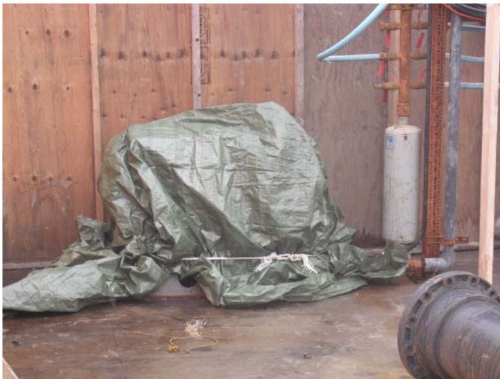
Figure 18: Chemical Makeup Blower Storage (Platform)
