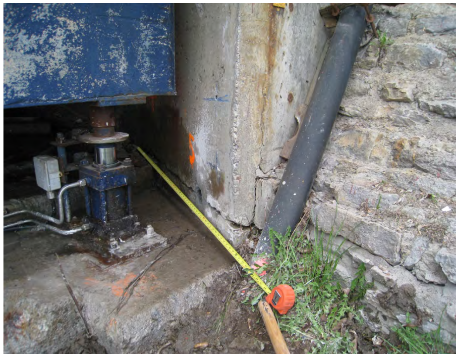
No.24: The northeast of the swing bridge; note the nearly-straight-line crack from the edge of the wing wall extending west to a distance of about 1.5 m.
