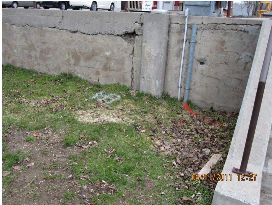
No.25: The retaining wall on the northwest side of the swing bridge; note the upper portion of the concrete was poured in different years and cracks between the different pours; note the deterioration of lower portion concrete.
