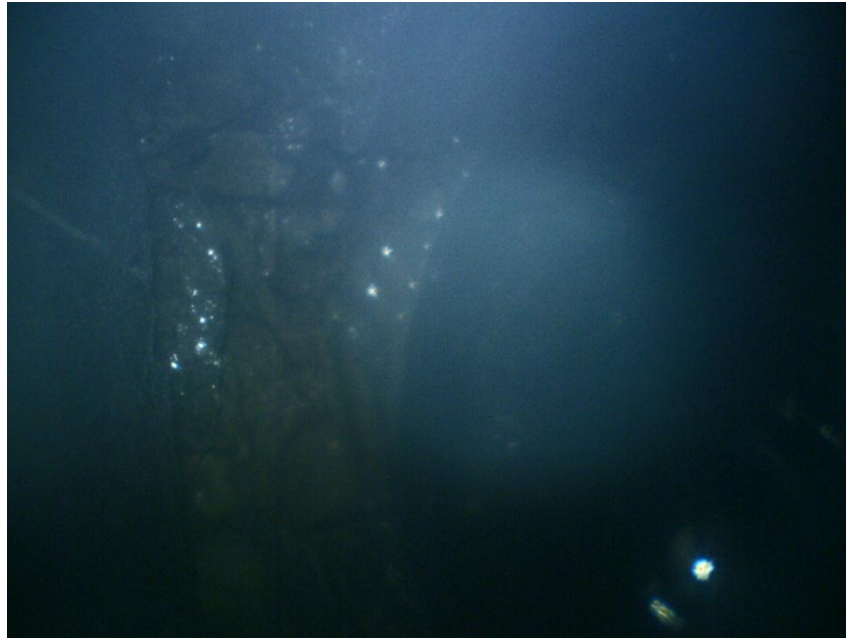
Photograph 3: highly weathered rock between pier concrete and bedrock
