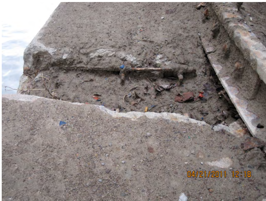
No.20: The north canal concrete wall; note the deterioration of concrete on the wall surface and exposed and eroded steel rebar and the void underneath the steel track on top of the central pier.
