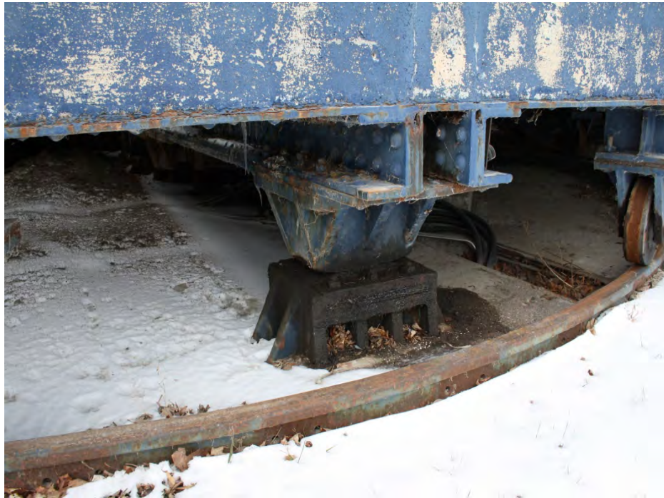
No.19: The central concrete pier; note the circular steel track on top of the concrete pier, the balance wheel on the track and steel pillow block rest to support the transverse beam of the swing bridge.
