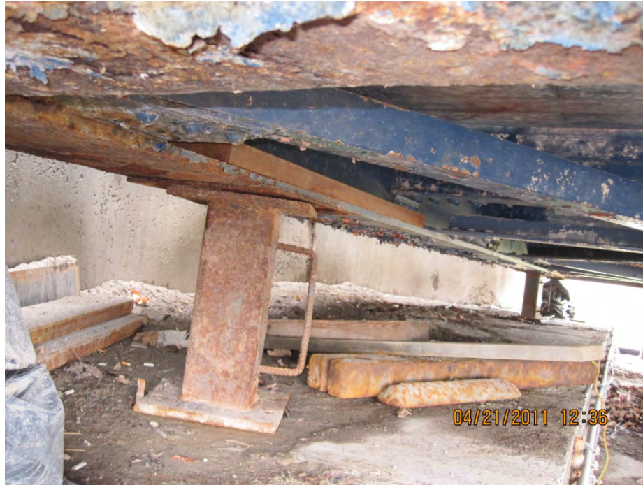
No.15: The north abutment underneath the bridge deck, looking east; note two steel posts used to support the bridge during the non-operational seasons.
