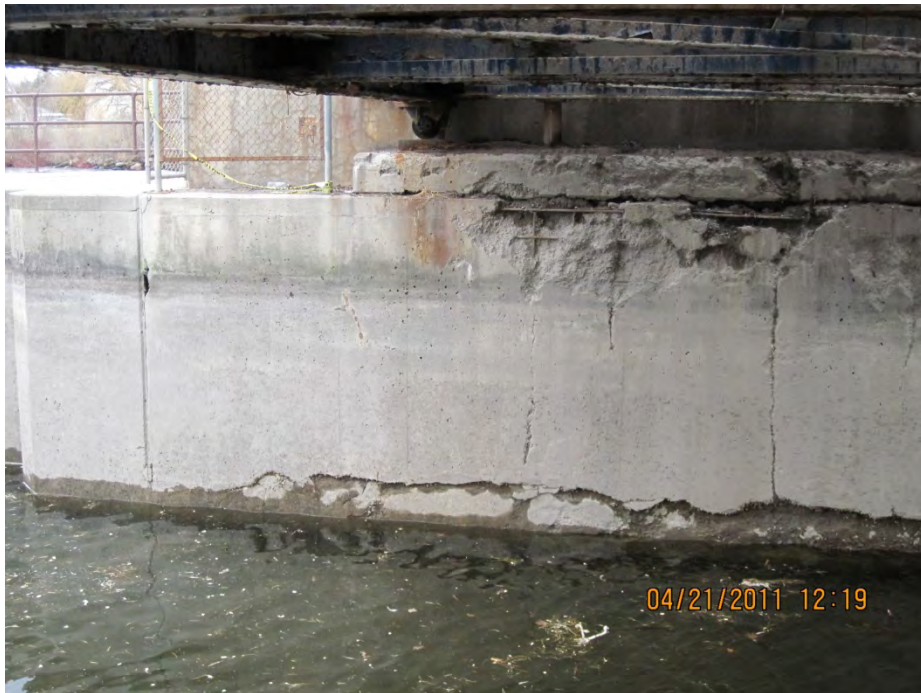
No.12: The south abutment underneath the bridge deck, looking south; note the deterioration of the concrete, exposed steel rebar at or immediate below the abutment slab; also note the nearly horizontal deterioration of the concrete at lower portion of the south canal wall.
