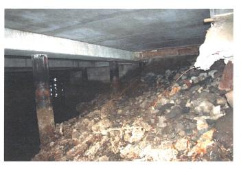
PHOTO C17-05 FORESHORE FILL MOUND UNDER STEEL PILED CRANE PAD - LOOKING NORTHWEST TOWARDS TIMBER CRIB
