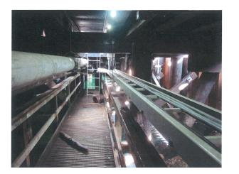
PHOTO C16-02 SOUTH JETTY CATWALK WITH MECHANICAL AND ELECTRICAL SERVICES
