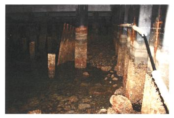
PHOTO C14-06 PAINTED SHEET PILE BULKHEAD - NOTE CATHODIC PROTECTION AND REMNANTS OF LOWER SHEET PILING (TIDE APPROX. EL+1.0M)
