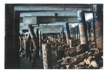
PHOTO C14-04 STEEL PILED CONCRETE DECK LOOKING WEST - NOTE CATHODIC PROTECTION CABLES AT SLAB SOFFIT
