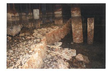
PHOTO C14-07 REMNANTS OF LOWER SHEET PILING -NOTE SHEET PILED BULKHEAD IN BACKGROUND
