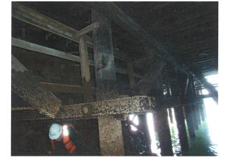
PHOTO C15-05 TIMBER PILED JETTY - VIEW AT EAST END FIRE STOP WALL AND CATWALK (BEFORE SHEET PILE PERIMETER WALL WAS INSTALLED)
