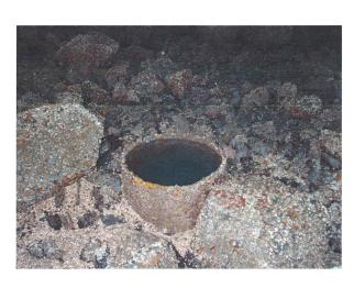
PHOTO C14–09 OPEN STEEL PIPE PILE UNDER STEEL PILED CONCRETE DECK – NOTE SAFETY RISK
