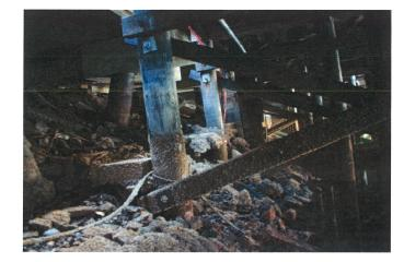
PHOTO C15-06 TIMBER PILED JETTY AT INTERFACE WITH STEEL PILED DECK- NOTE RIPRAP ON FORESHORE AND MISCELLANEOUS CONCRETE FOOTINGS
