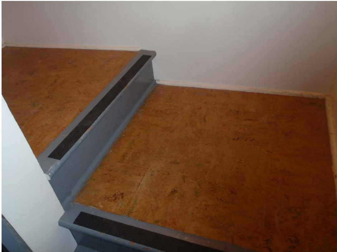
House #9 - 18 - Non-asbestos orange vinyl floor tiles throughout house.
