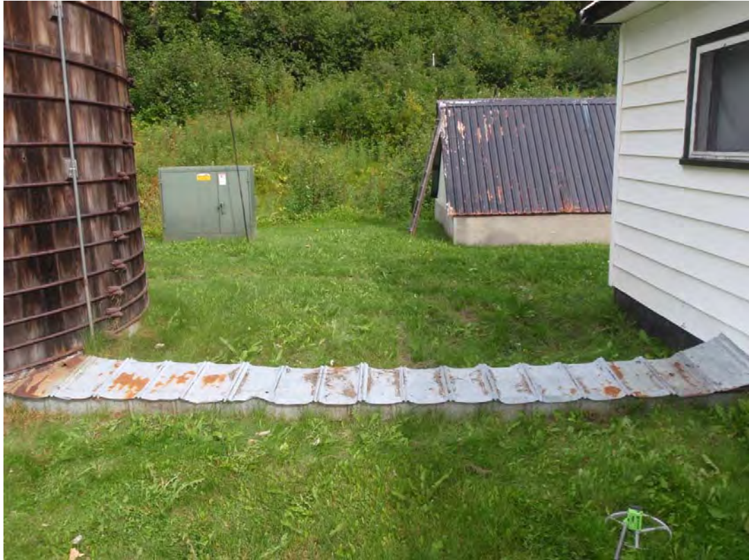
Water Storage Tank - 2 - Metal cladding over ground piping between Water Storage Tank and Generator Building.
