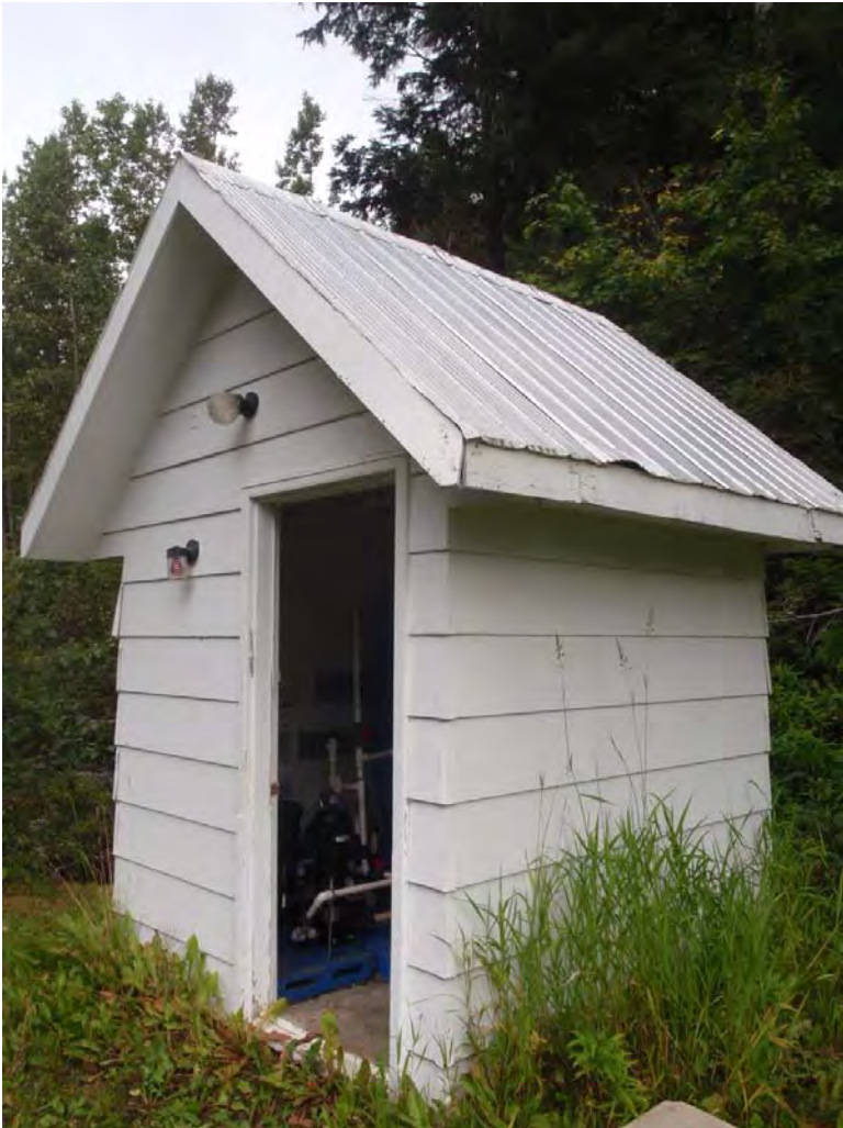
Pump House - 1 - Facing northwest.
