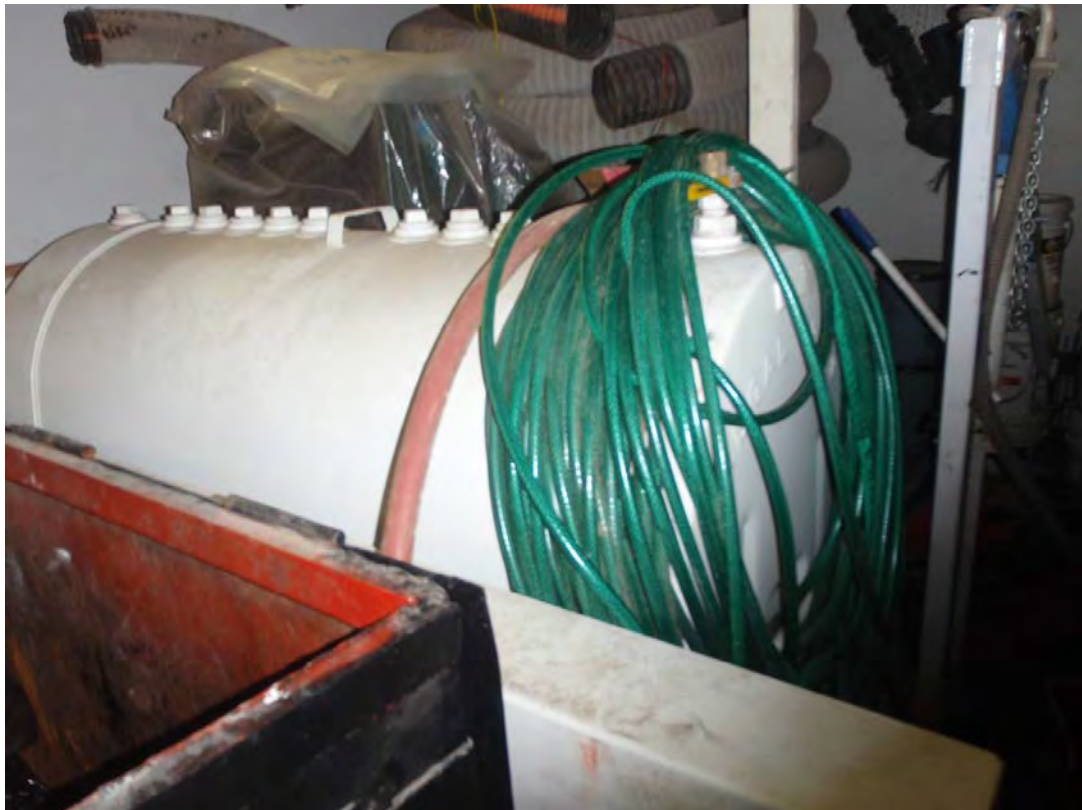
Secondary Examination Shelter - 8 - Unused AST.
