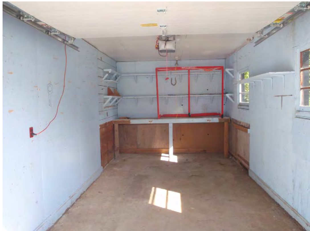
Garage - 2 - East bay of garage.
