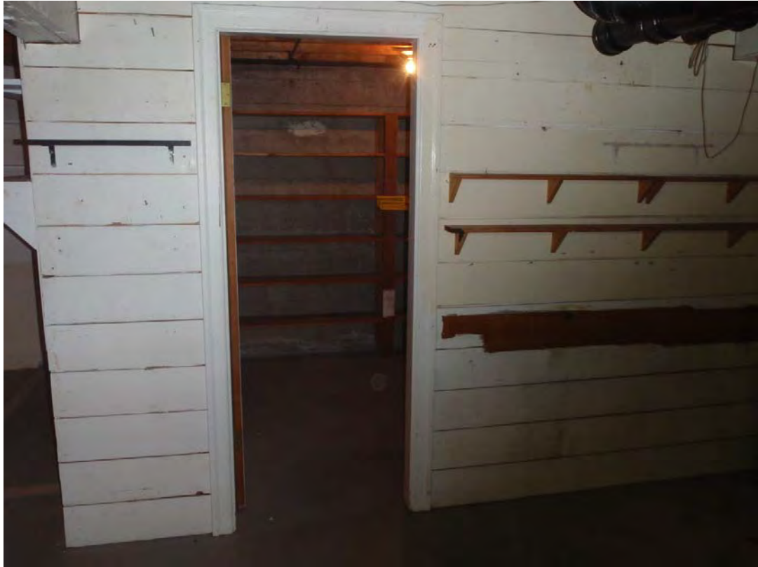
House #9 - 8 - Cold room in basement.
