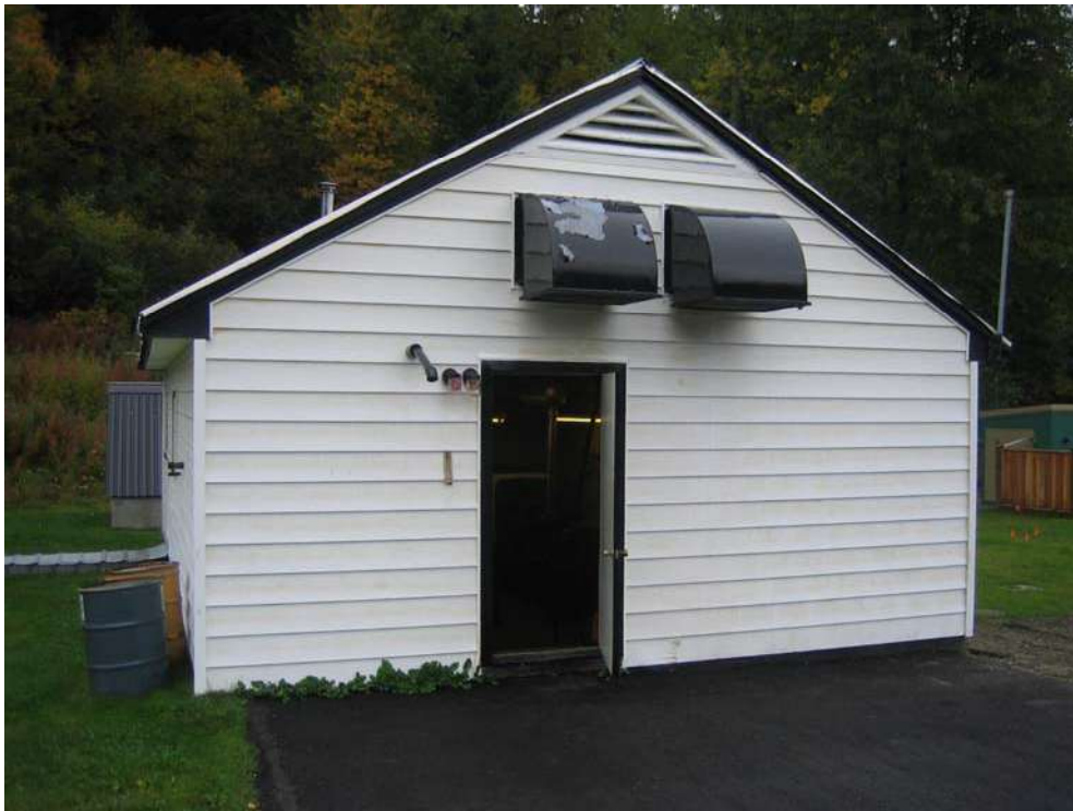
Maintenance Building, looking south east.
