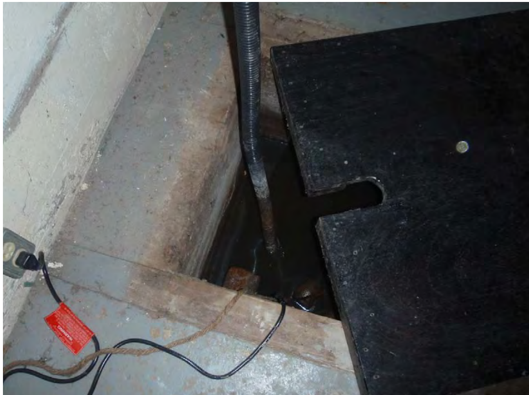
House #9 - 9 - Floor sump in basement.
