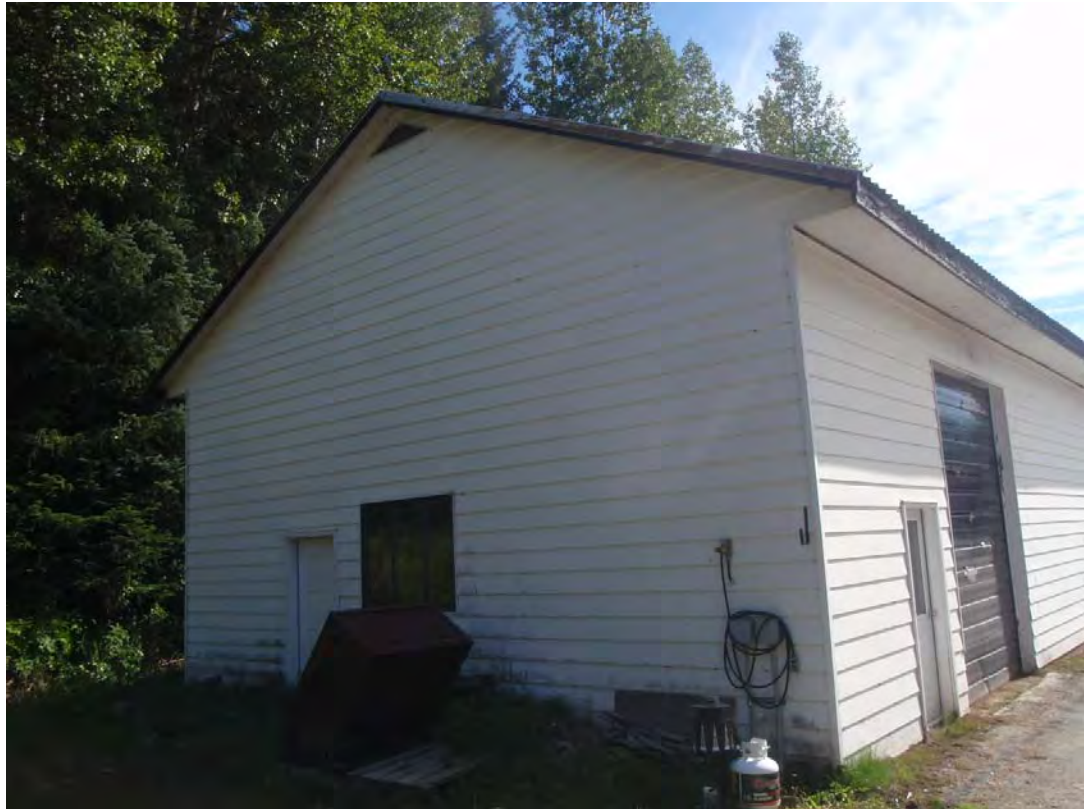
Secondary Examination Shelter - 1 - Facing northeast.
