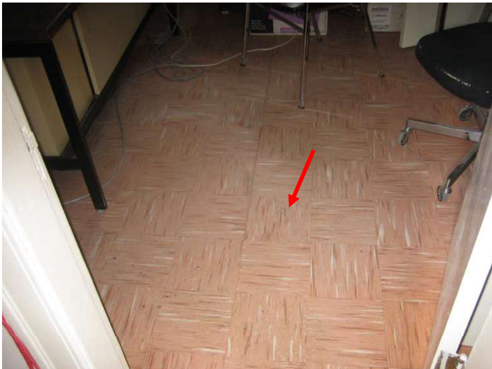
Diesel Storage Building, looking north east.
