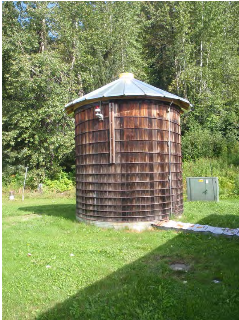
Water Storage Tank - 1 - Facing north.
