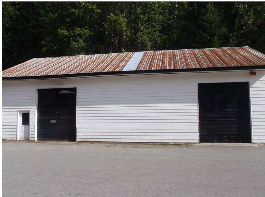
Secondary Examination Shelter - 2 - Facing north.
