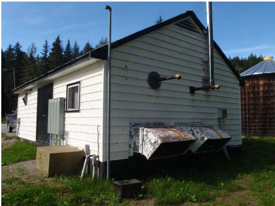
Generator Building - 2 - Facing southwest.
