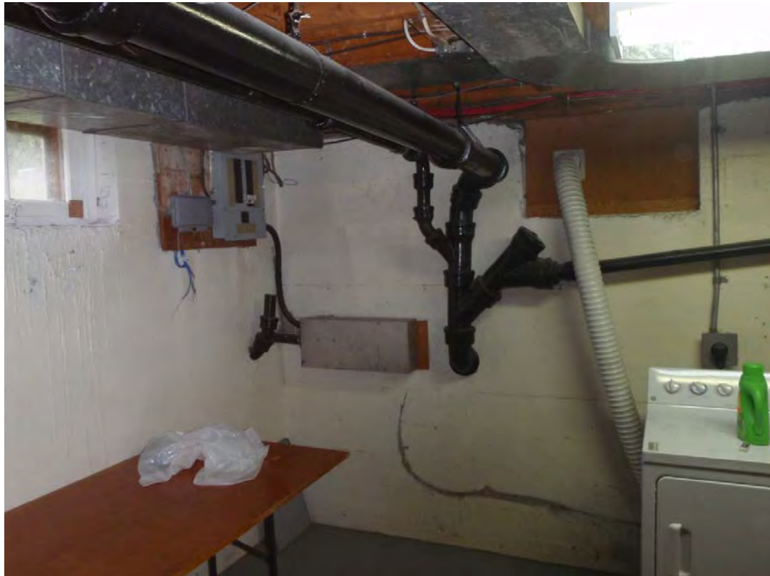
House #9 - 10 - Cast iron piping in basement.
