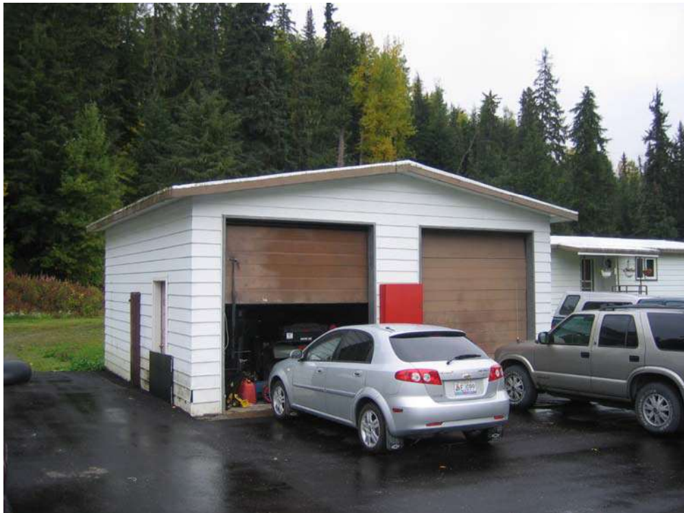
House #5, looking north east.
