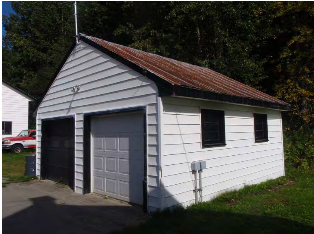
Garage - 1 - Facing northwest.
