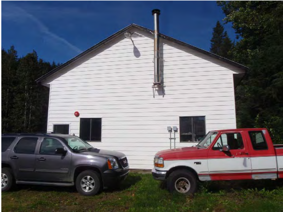
Secondary Examination Shelter - 3 - Facing northwest.
