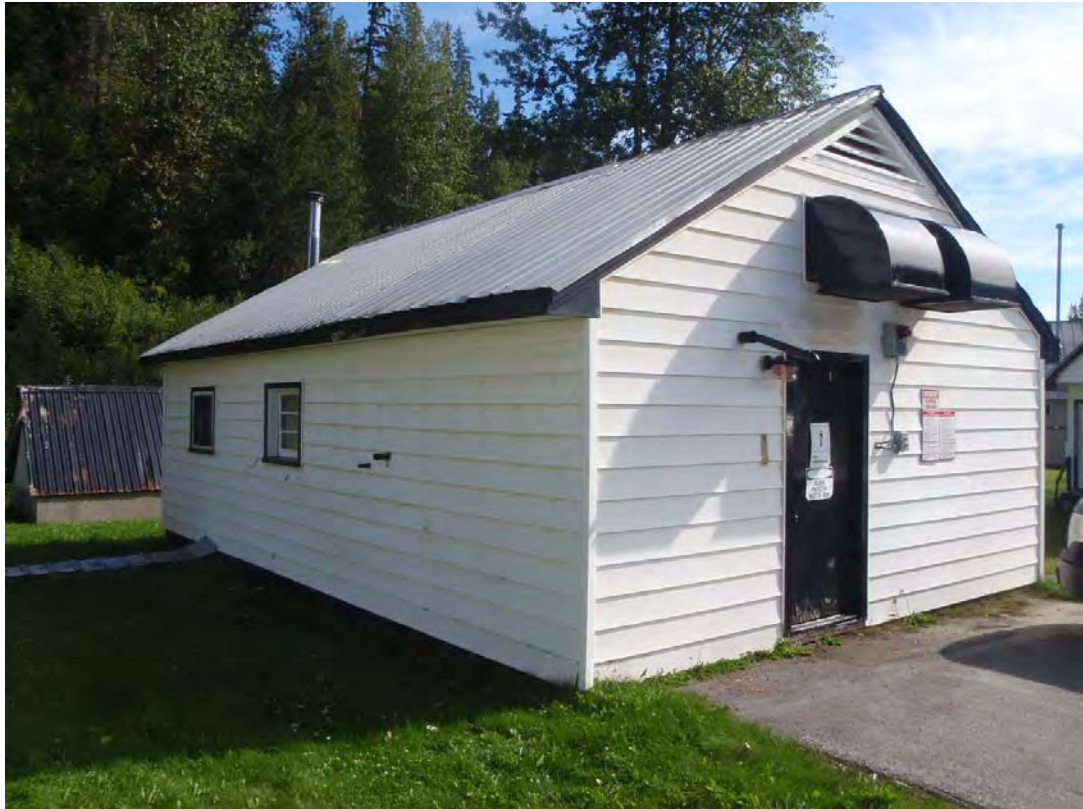
Generator Building - 1 - Facing northeast.
