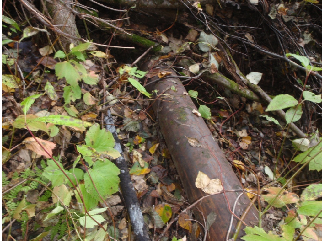
Photograph 5: Abandoned section of pipeline identified within the right-of-way.
