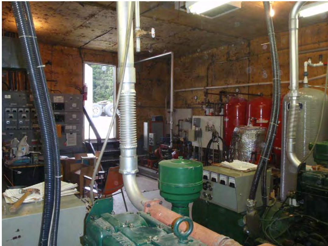
Generator Building - 4 - Facing southwest at newer area.
