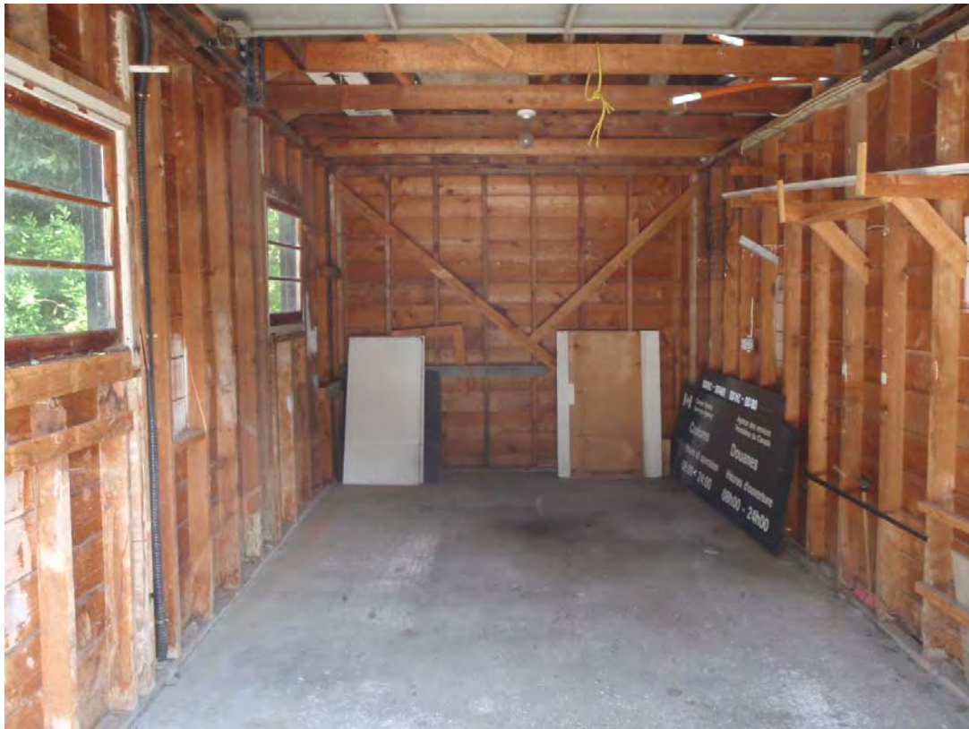
Garage - 3 - West bay of garage.
