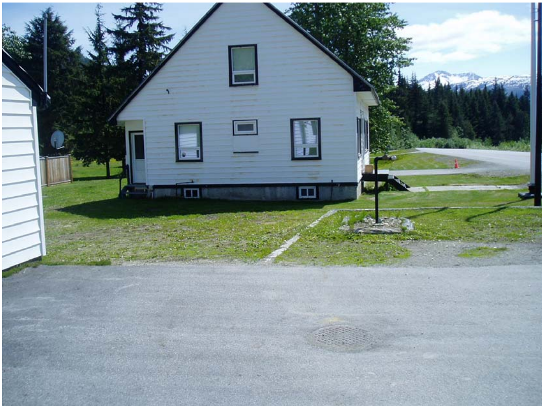
Photograph 6: View looking east at House #5. The fuel fill pipe and fuel transfer area is visible in the foreground.
