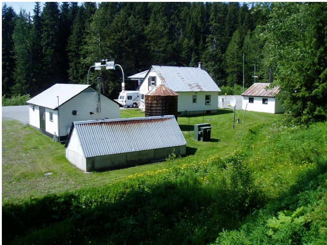
Photograph 2: Border crossing facility, facing west, with generator building, water tank and fuel tank in foreground (June, 2008).
