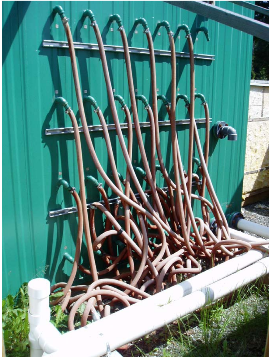
Photograph 23: Air sparge and SVE header connections.
