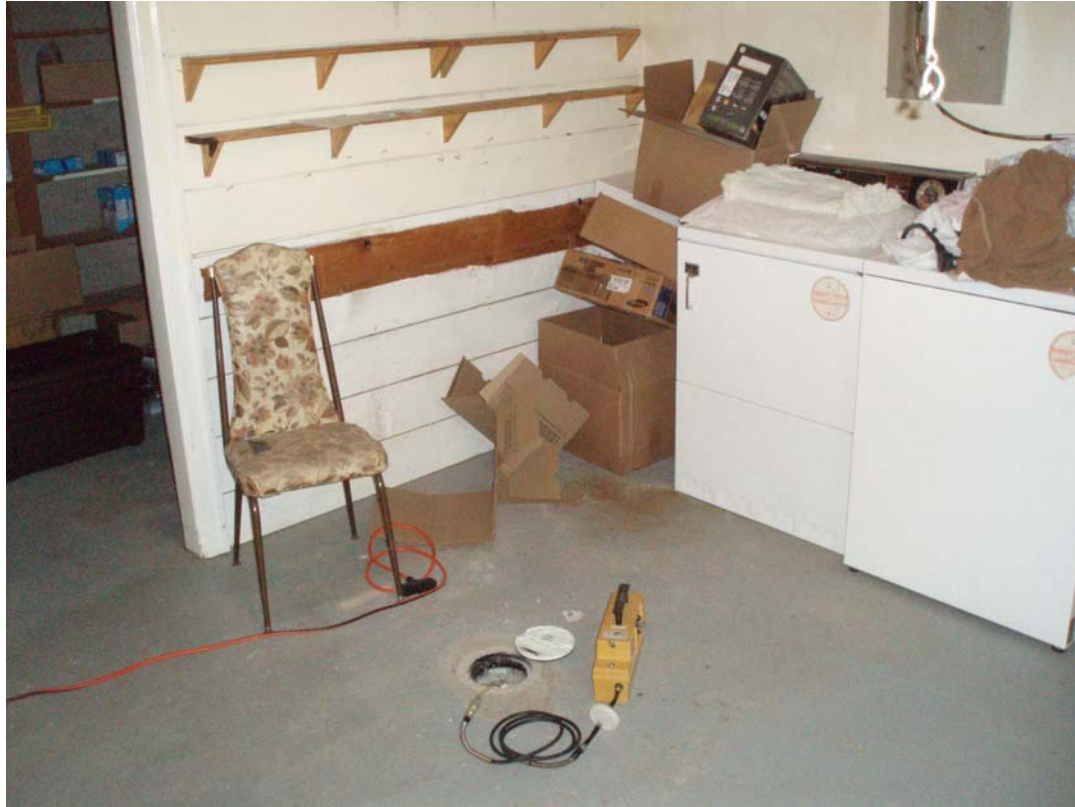
Photograph 17: Sub-slab soil vapour well SVW09-1 installed in the basement of House #5.
