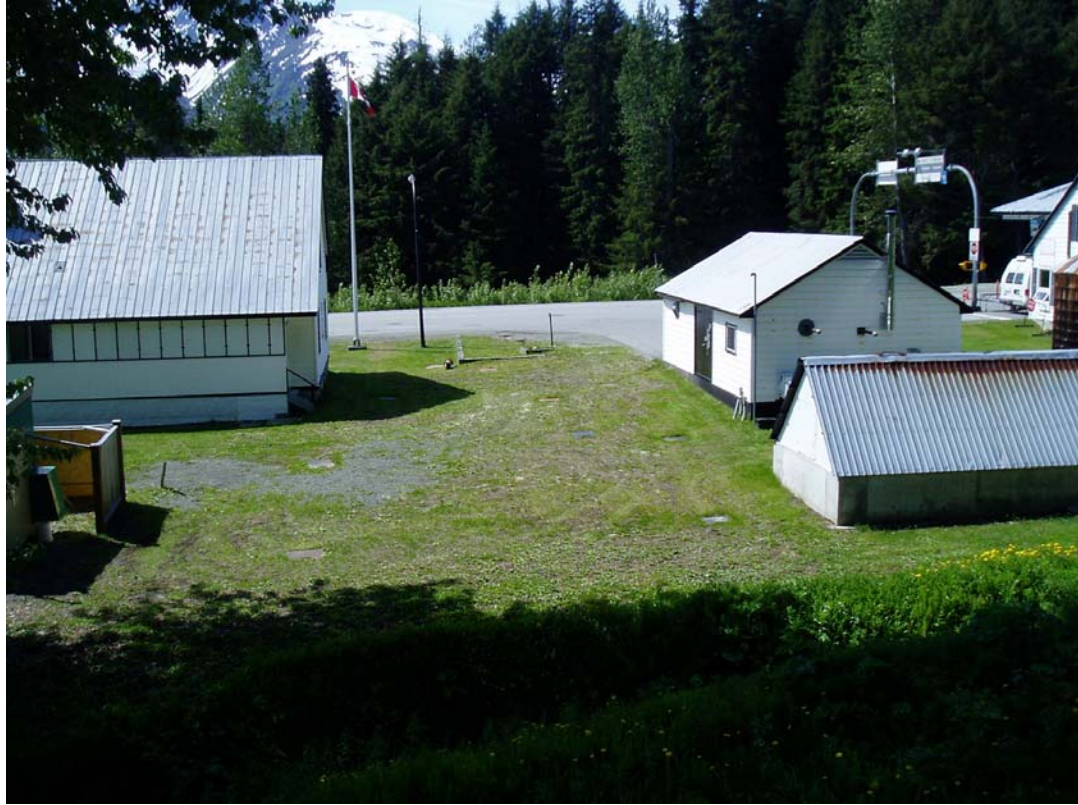
Photograph 7: View looking southwest between House #5 and the Generator Building.
