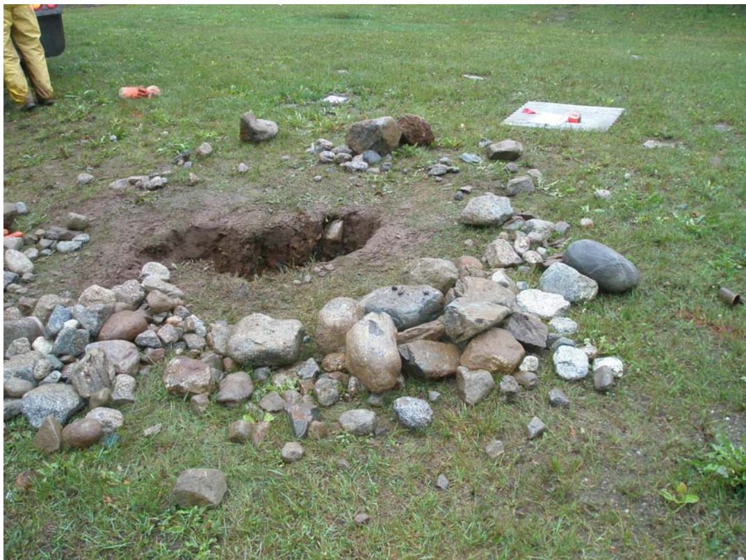
Photograph 12: Boulders and cobbles removed by the hydrovacuum rig from BH09-11.
