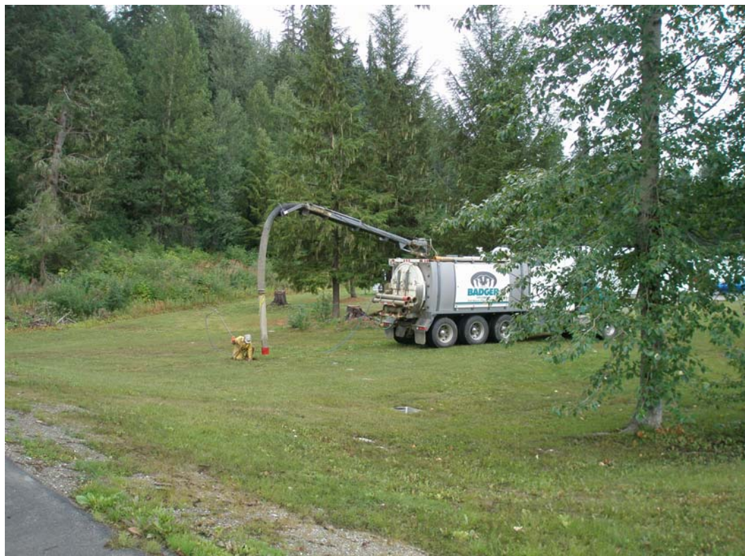
Photograph 10: Hydrovacuum rig working at BH09-11 adjacent to the underground fuel line.
