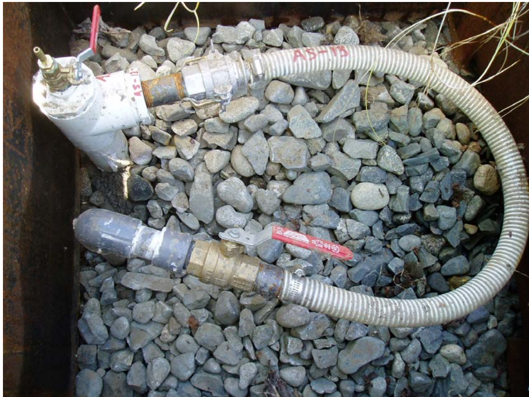
Photograph 27: Typical air sparge well.
