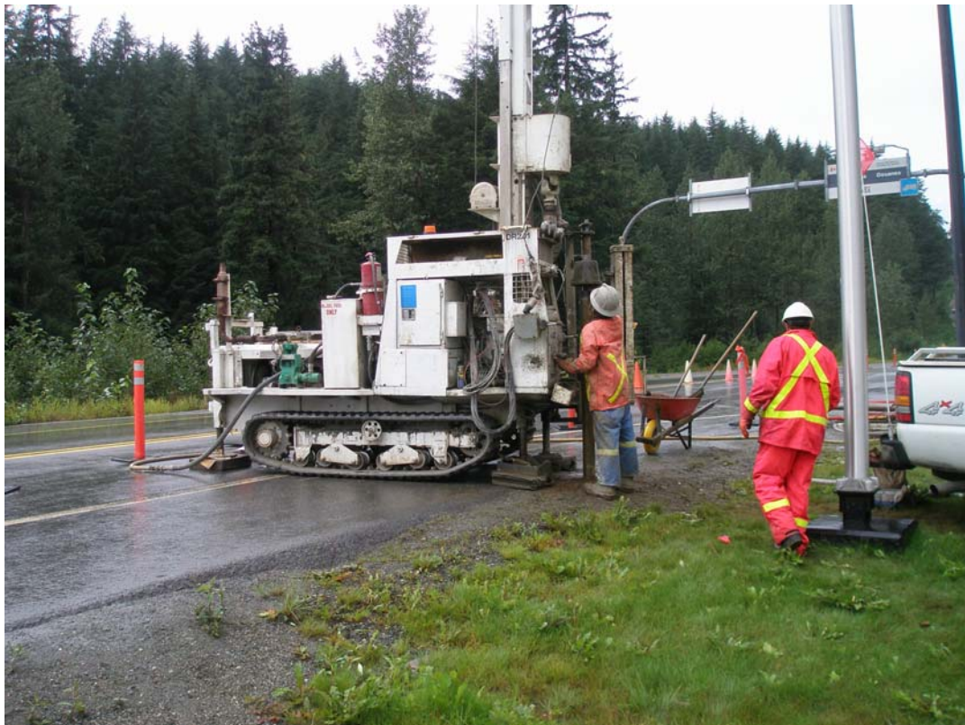
Photograph 14: Drilling at BH09-17 on Haines Hwy. August 2009.
