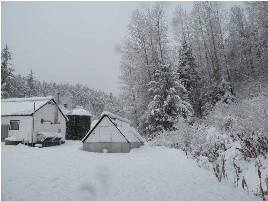
Photograph 8: View of fuel tank, generator building and water tank, with ditch to right and Grove 2 in background, facing west (October 2012).
