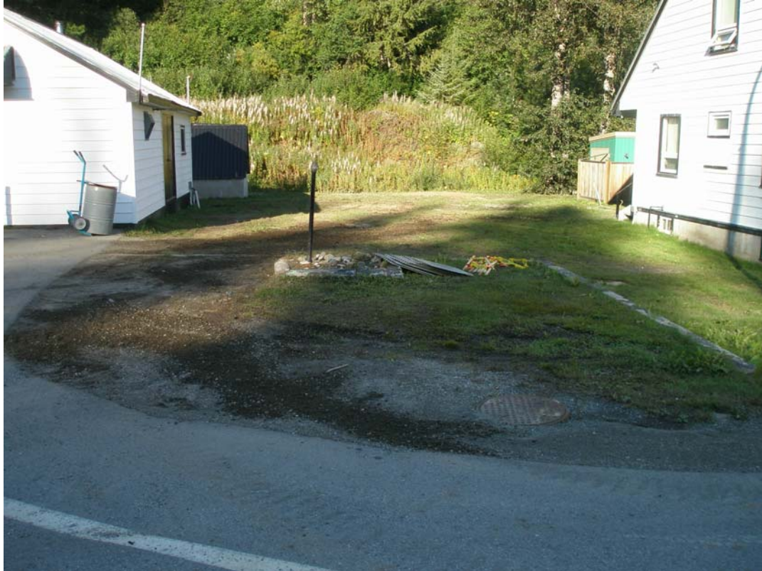
Photograph 5: View looking north between the Generator Building and House #5. The fuel transfer area and fill pipe is visible in the foreground.
