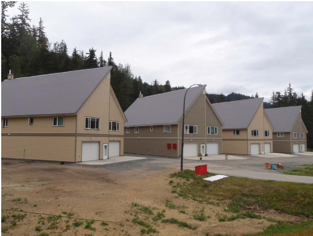
Photograph 5: View of new residential units (#1 to 8 from right), facing east (October 2011).
