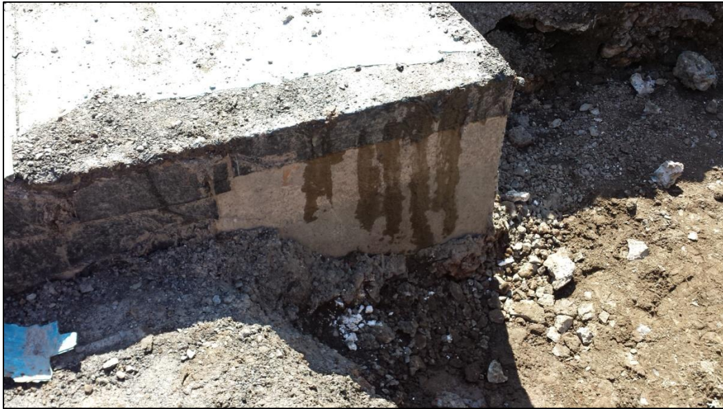
Photo 5 - Exposed corner of existing tunnel within east portion of TP 12D.
