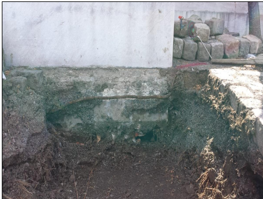
Photo 1 – Silty sand fill at base of test pit along with the existing perimeter wall foundation exposed at TP 1A.
