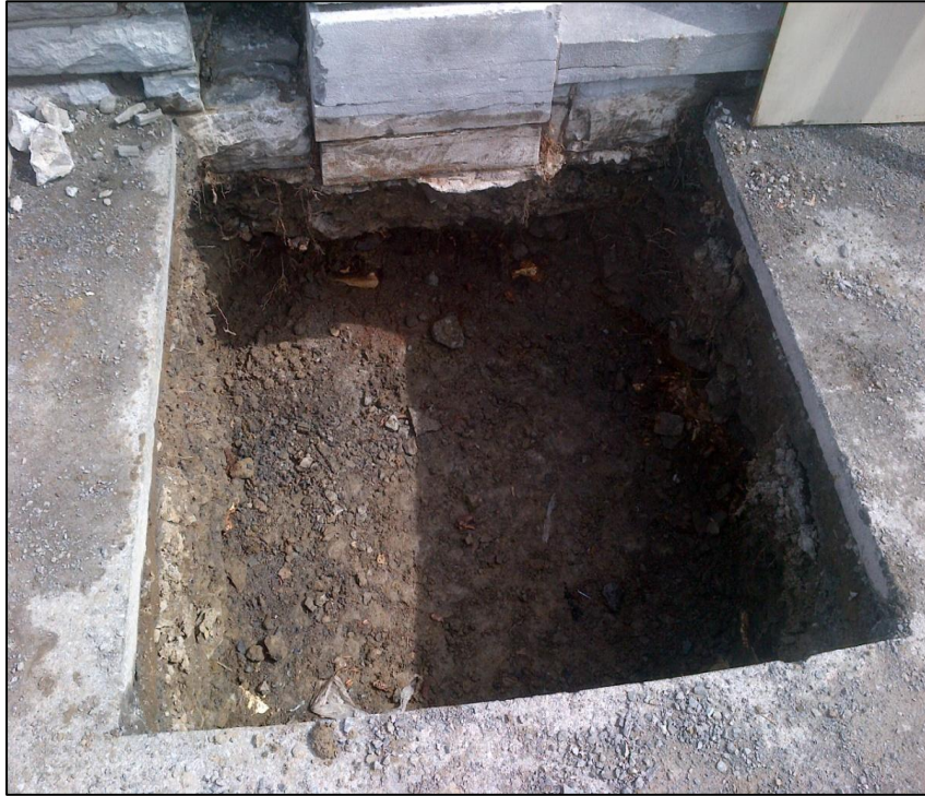
Photo 1 – Silty sand fill at base of test pit along with the existing perimeter wall foundation exposed at TP 1A.
