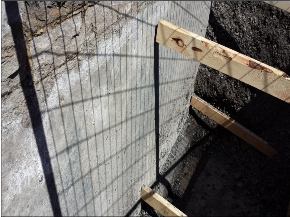
Photo 4 - Exposed foundation wall and top of tunnel at TP 9C.
