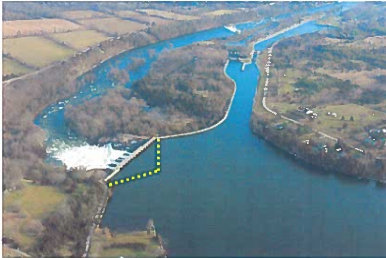
Photo 1 - Aerial Photo looking downstream. Healey Falls Dam seen at left. Lock 17 is seen to right of dam. Approximate proposed boom location shown as yellow dashed line. Intent is to direct watercraft away from dam and towards the lock. An inverted v-shape layout is proposed to promote self rescue.
