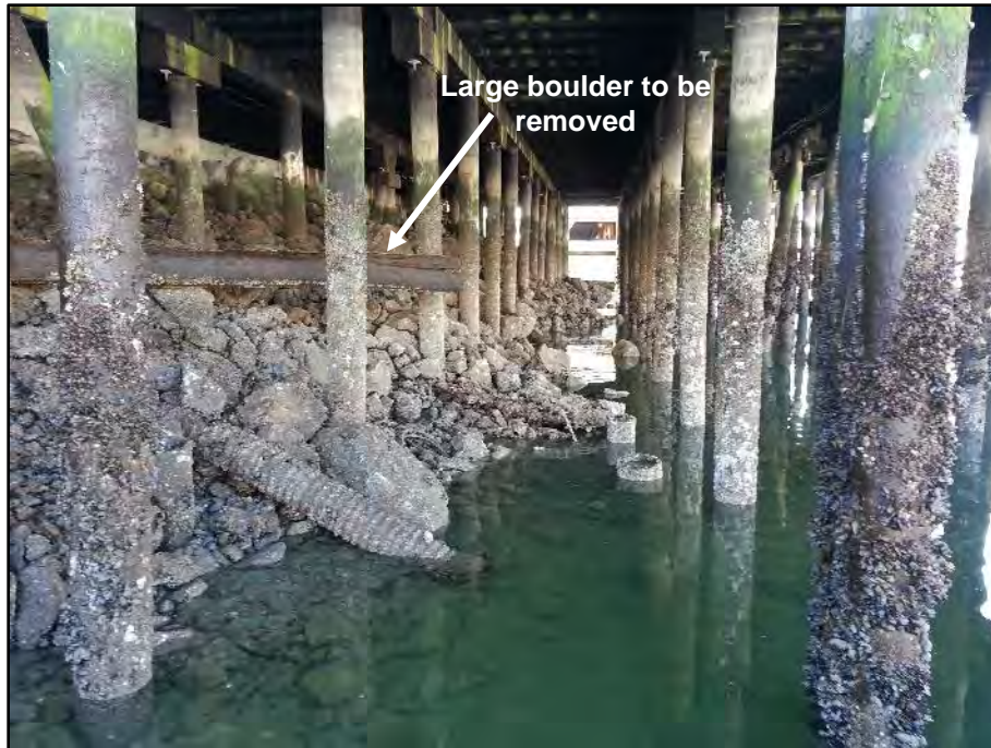
Photo 18 View underneath Bridges Dock Facing Southwest Showing the Concrete Abutment (left) and Piles where Steel Bands will be Installed
