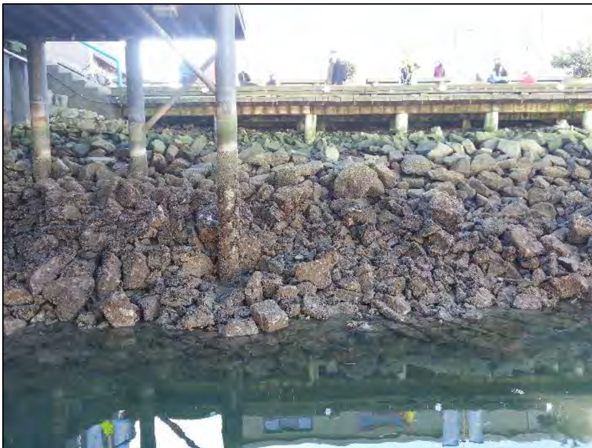
Photo 5 View of the Rip Rap Slope adjacent to the Public Market Boardwalk
