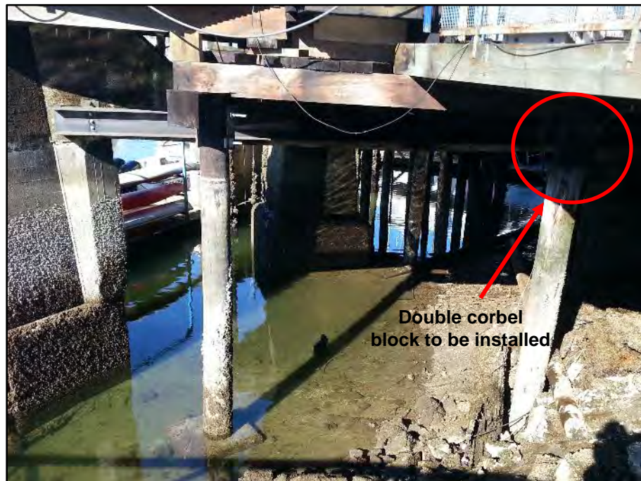
Photo 17 Location of Proposed Installation of Corbel Blocks under Lion's Gate Dock
