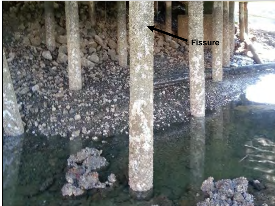
Photo 16 Example of Wooden Piles with Compromised Structural Integrity, under the Lion's Gate Dock
