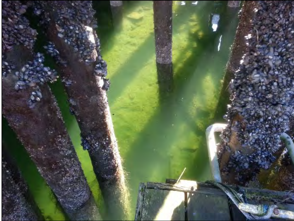
Photo 6 Wooden Piles underneath West Dock
