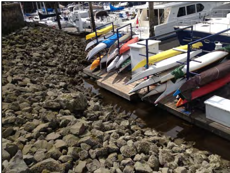
Photo 11 View of a Stranded Floating Dock at Low Tide Adjacent to the Maritime Market Boardwalk (Photo Courtesy of Parsons)
