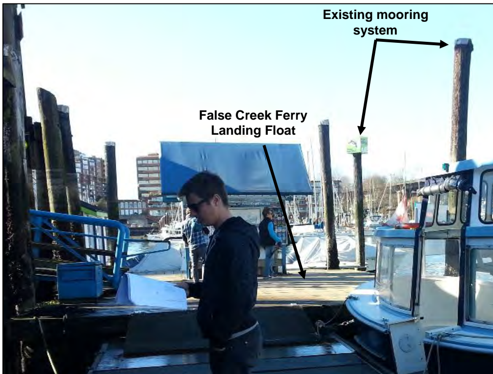
Photo 14 False Creek Ferry Landing Float with Wooden Mooring Piles
