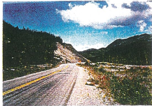
Photo 4: Viewed from 741+200 Facing North
