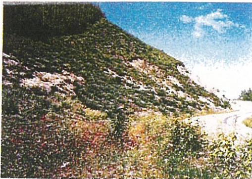
Photo 9: Viewed from 746+125 Facing North
