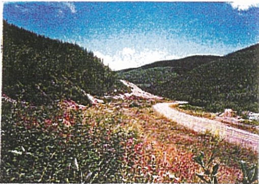
Photo 8: Viewed from 745+150 Facing North
