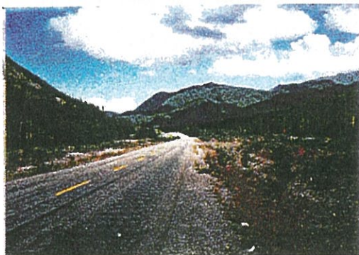
Photo 3: Viewed from 740+200 Facing North
