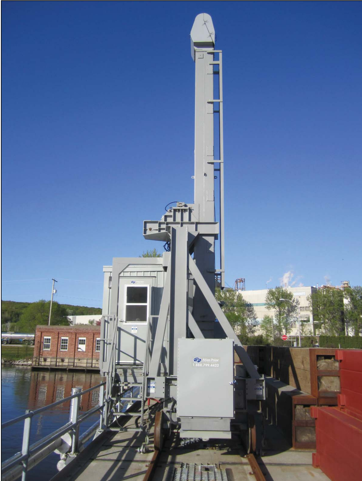
Figure 4 - Right end of Quebec Dam's stoplog lifter.
