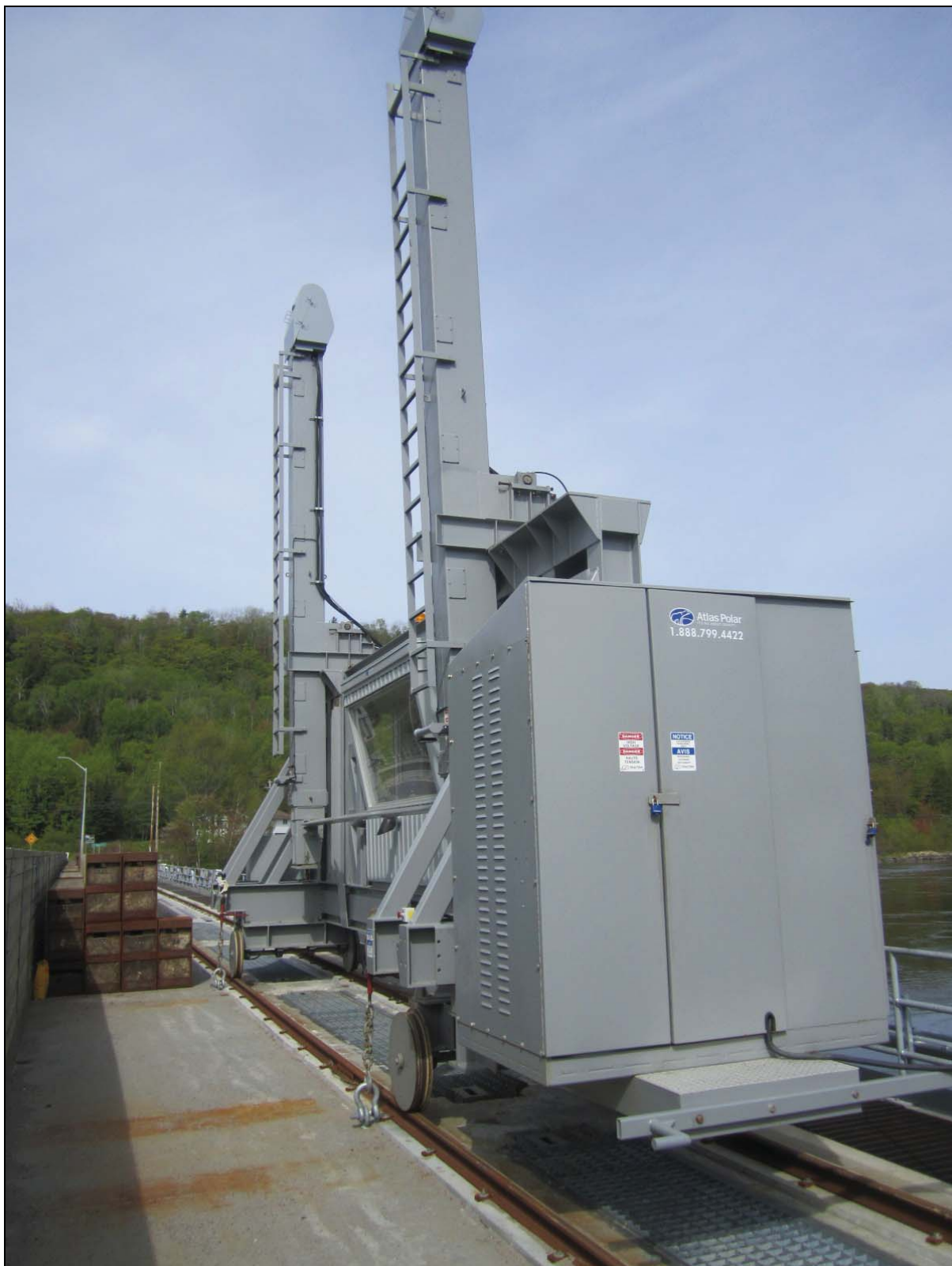
Figure 3 – Ontario dam's stoplog lifter, left end and downstream side.
