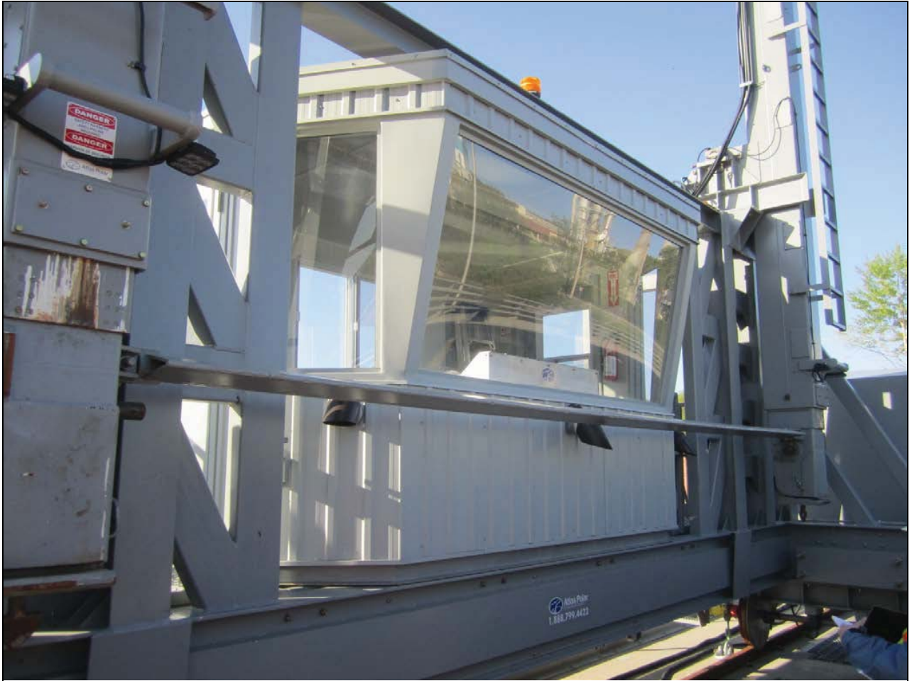
Figure 2 - Stoplog lifter, downstream side, with booms in vertical and raised position. Note lack of overhang protecting the window.
