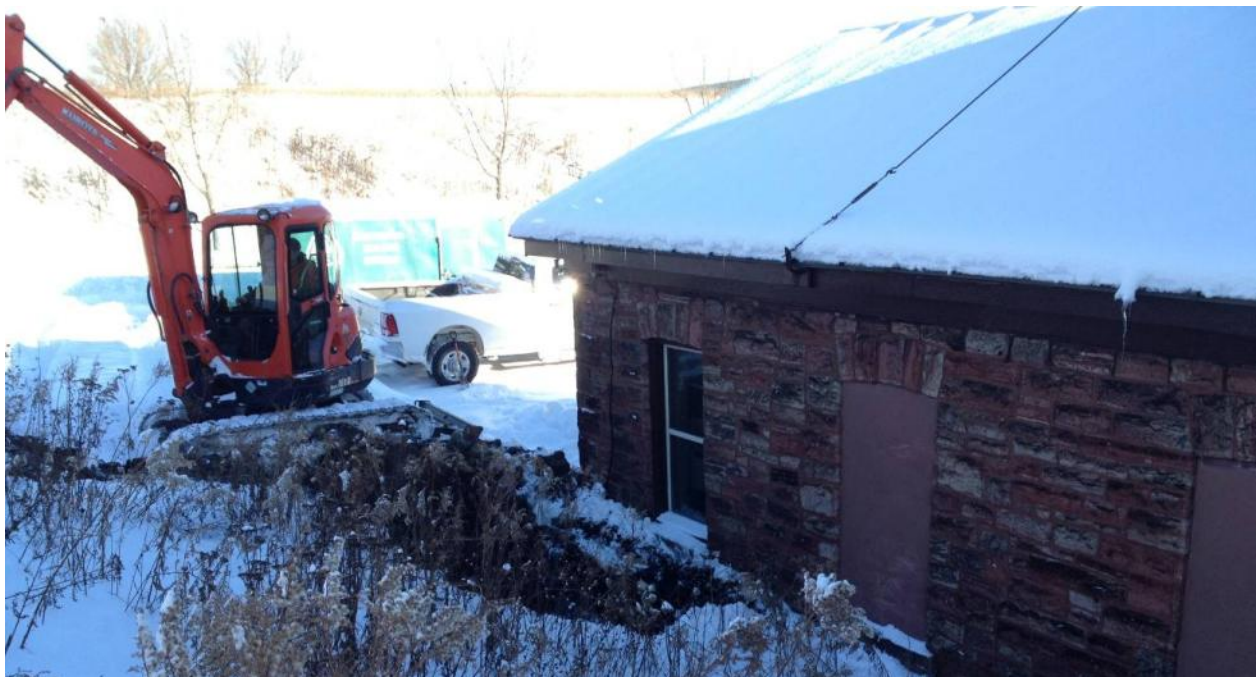
Photo 2: View of TP13-03 excavated at northwest corner of the building. The northern portion of the building does not appear to be moving, so this test pit was for comparative purposes.
