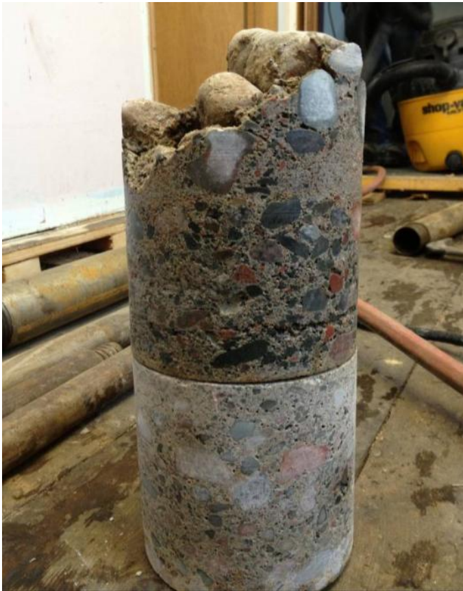
Photo 4: Core of floor slab.
