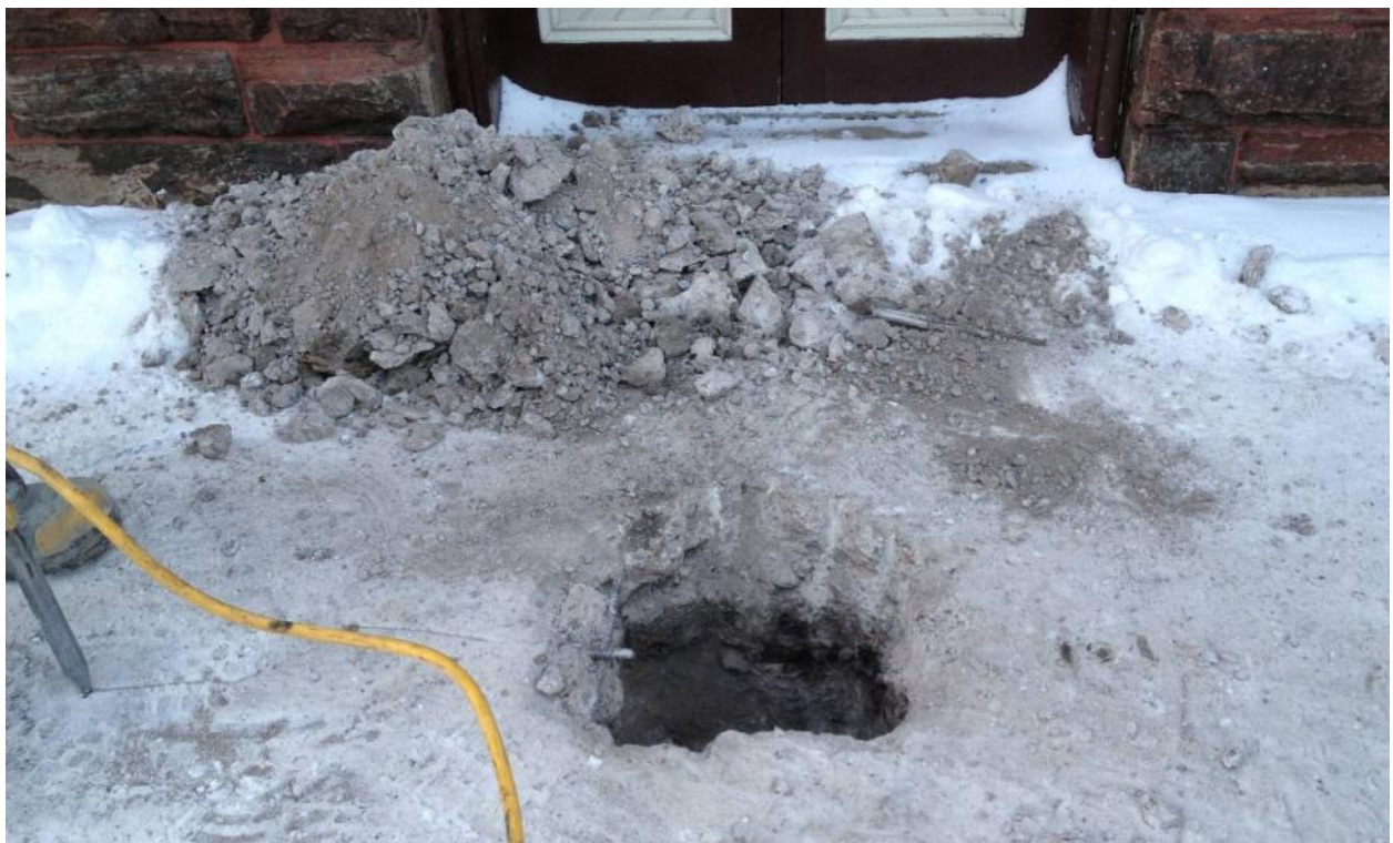
Photo 1: Jack hammered hole for pump well installation.
