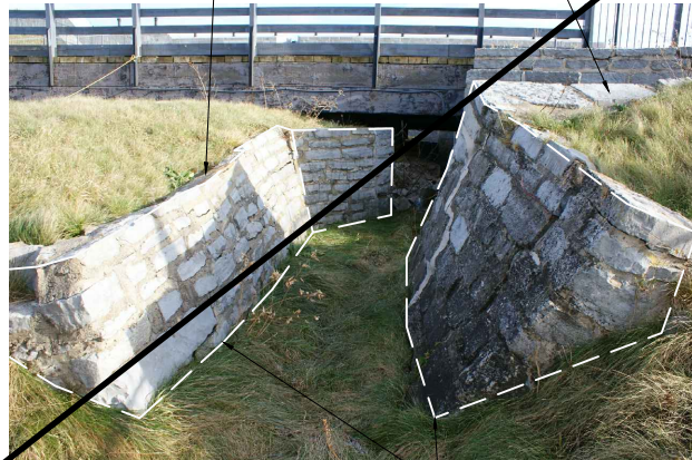
PHOTO 42: MASONRY WALL AT BRIDGE-EAST SIDE-3 N.T.S
