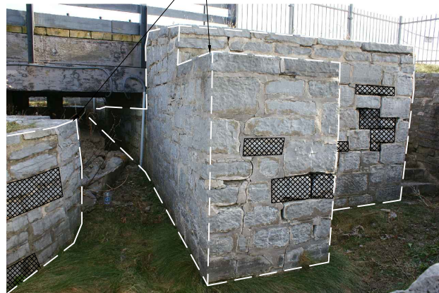
PHOTO 40: MASONRY WALL AT BRIDGE-WEST SIDE-1 N.T.S
