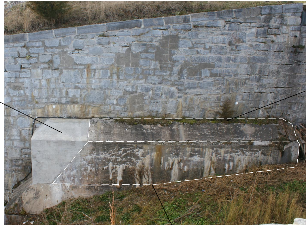
PHOTO 44: EAST BRANCH DITCH BUTTRESS N.T.S.
