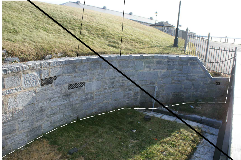
PHOTO 37: MASONRY WALL AT BRIDGE-EAST SIDE N.T.S
