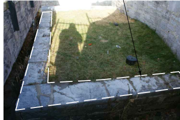
PHOTO 38: WEST BRANCH BRIDGE-CAPSTONE WORK-1 N.T.S
