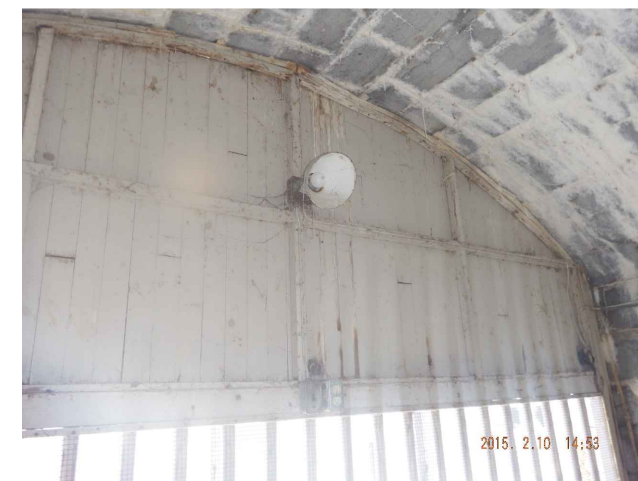
INTERIOR OF D5-01 - RIGHT
