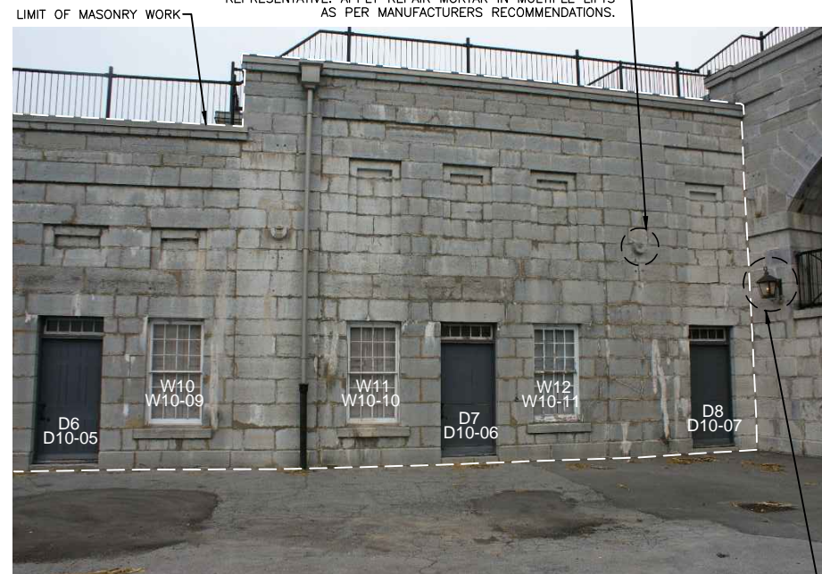
CAREFULLY DISMANTLE, TURN OVER TO OWNER FOR REPAIRS TO BE COMPLETED (BY OTHERS) AND RE-INSTALL AFTER MASONRY REPAIRS ARE COMPLETE
