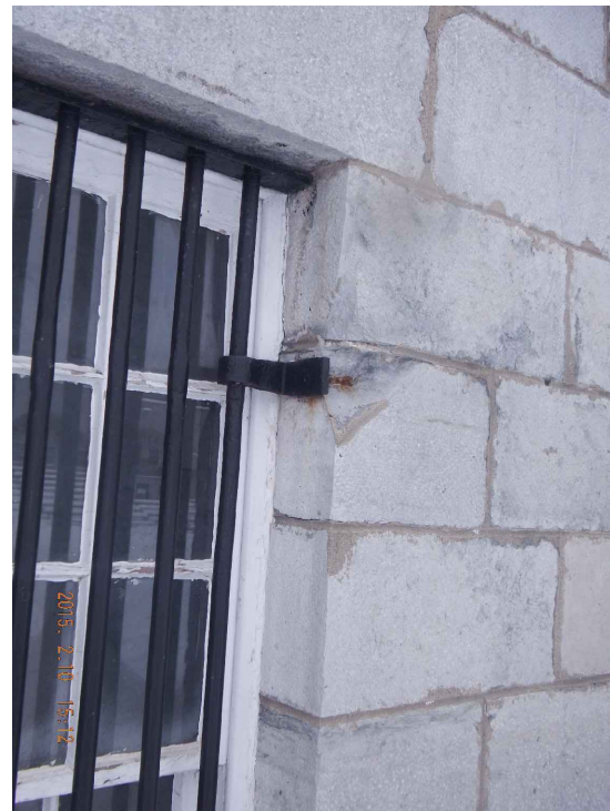
TYPICAL IRON PLUG TO BE REMOVED N.T.S.
