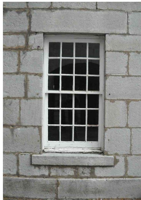
ORIGINAL 1938 UNIT REQUIRING REPAIRS - W10-01
