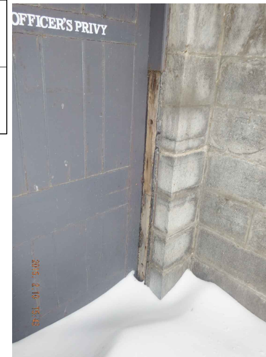
REPLACEMENT OF CASING BOARDS AT JAMBS- RIGHT SIDE SHOWN
