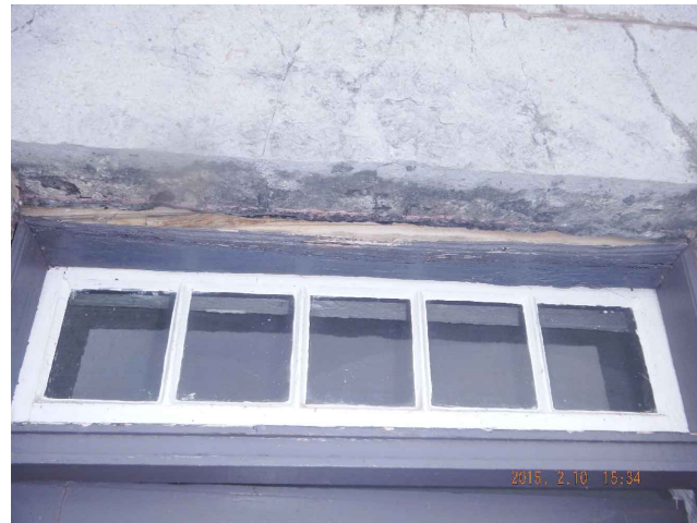
TYPICAL HEAD JAMB CASING REPLACEMENT
