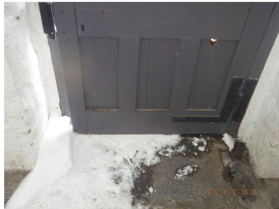
REPLACEMENT OF SPLIT PANEL & TYPICAL HERITAGE HINGES
