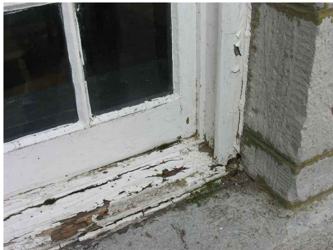
TYPICAL 1938 ORIGINAL WINDOW CONDITION - W9-01 N.T.S.
