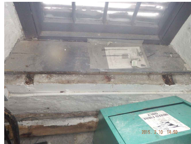
TYPICAL INTERIOR SILL REPLACEMENT N.T.S.
