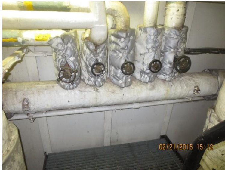
Steam Header pipe with 5 distribution/isolation valves
