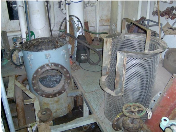
Port sea strainer opened up with basket removed.
