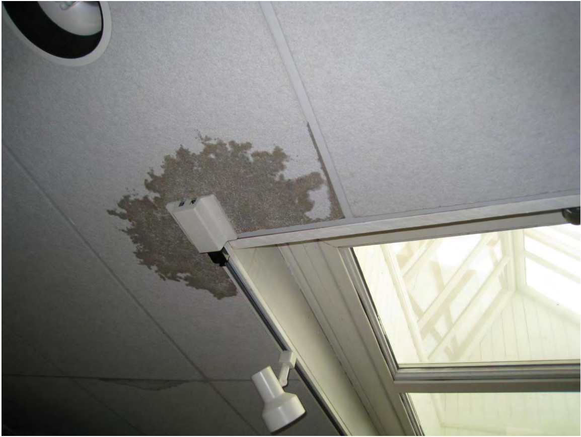
Figure 3: Skylight Leakage
