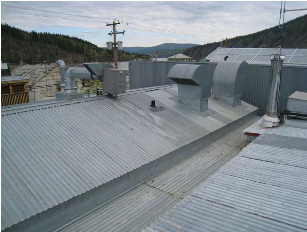
Figure 17: Transition zone between Annex and front of building
