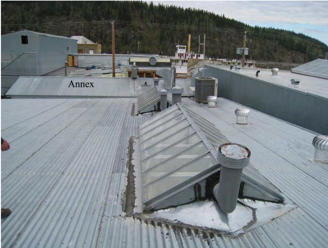
Figure 13: Roof looking back to Annex
