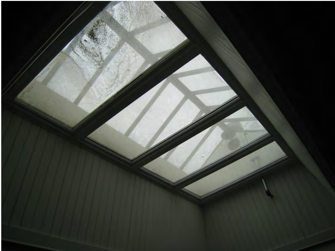
Figure 4: Skylight Condensation
