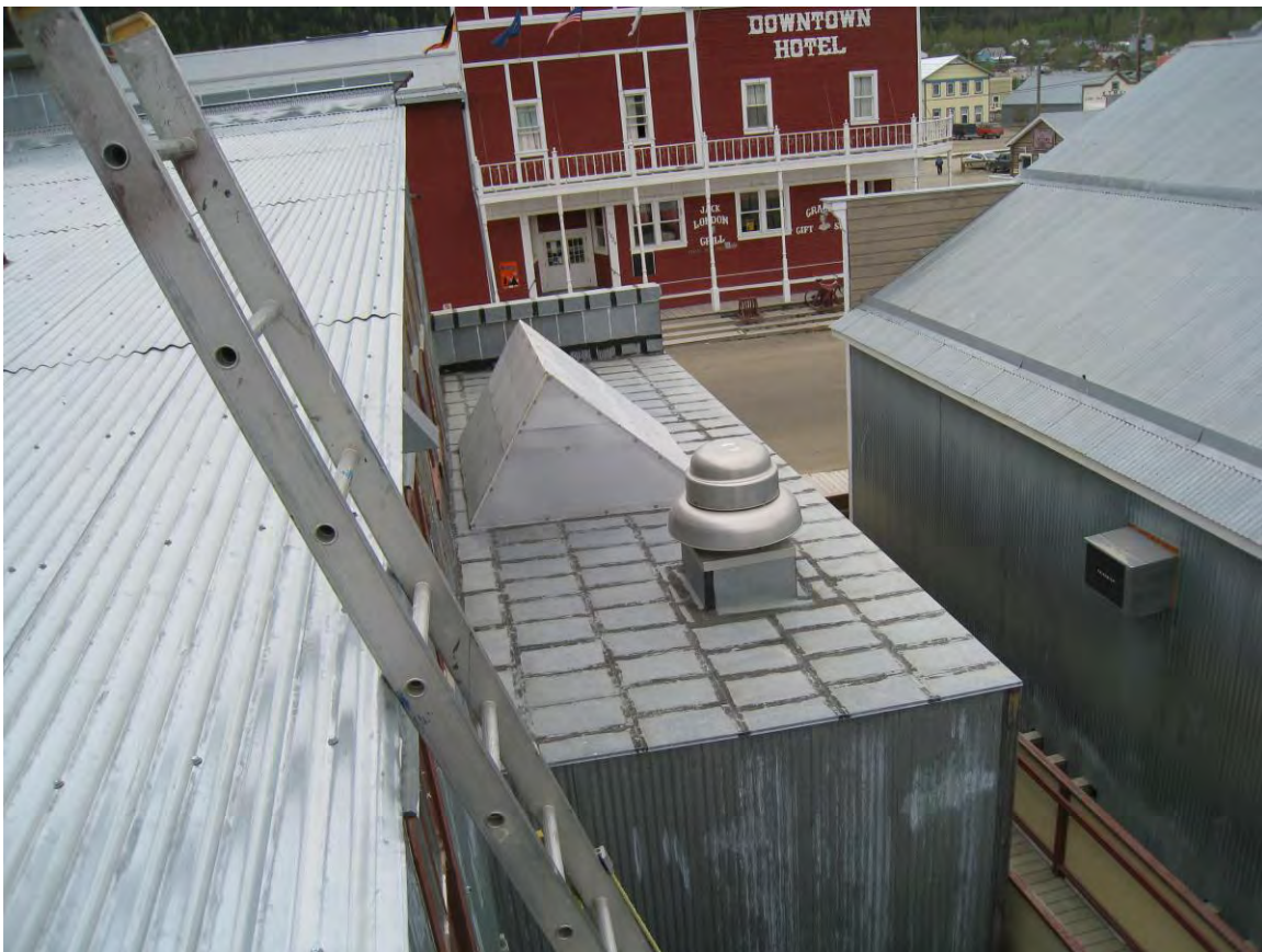
Figure 16: Lower roof with Coroplast frame over skylight
