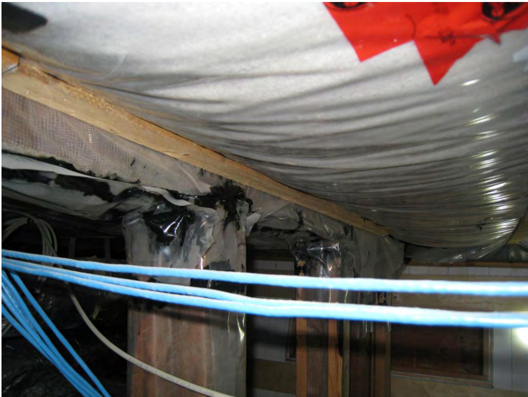
Figure 20: Suspended blown-in insulation in attic space
