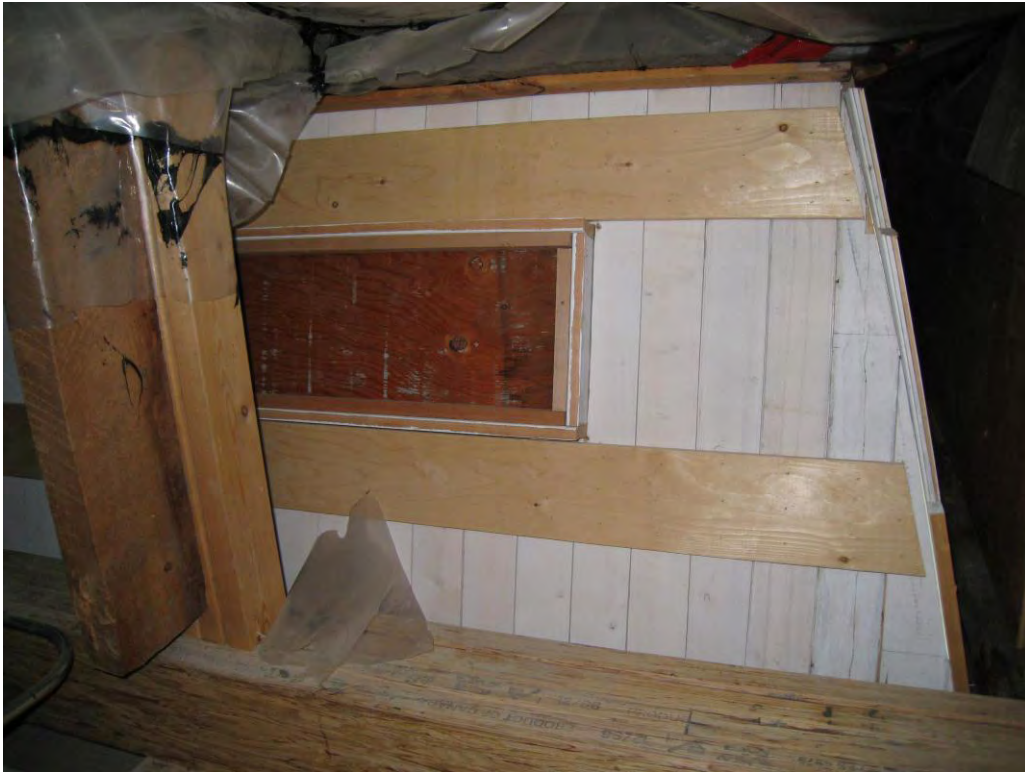
Figure 19: Skylight frame in attic space
