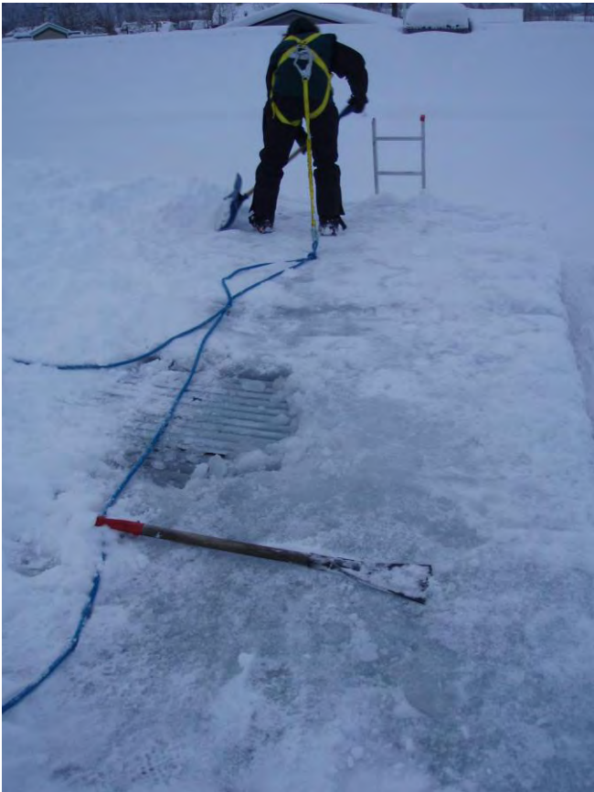
Figure 8: Ice damming at rear of roof (Feb. 2013)
