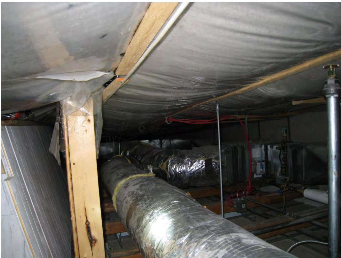
Figure 18: Attic space between suspended ceiling and roof near front of building
