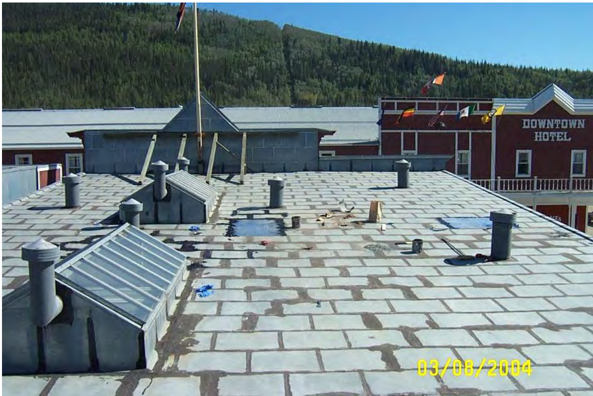
Figure 2: repairs to original roof
