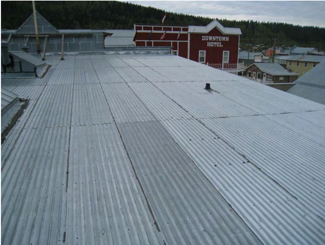
Figure 14: Roof looking towards front
