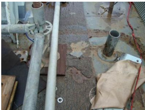
Deteriorated coating on Flag Deck
