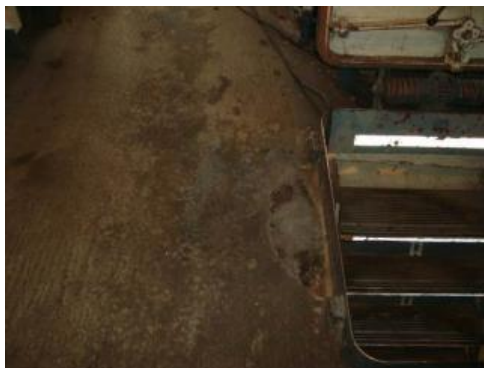
Bare metal and worn coating Port Hangar Lobby
