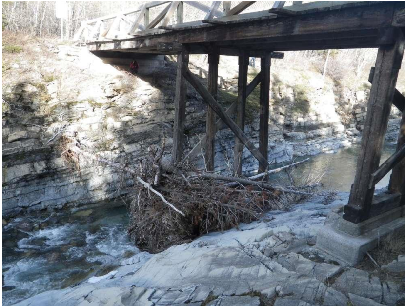
Photo 3: View downstream of the Canyon Church Camp Bridge crossing and flood debris jam on the instream pier (January 27, 2015)
