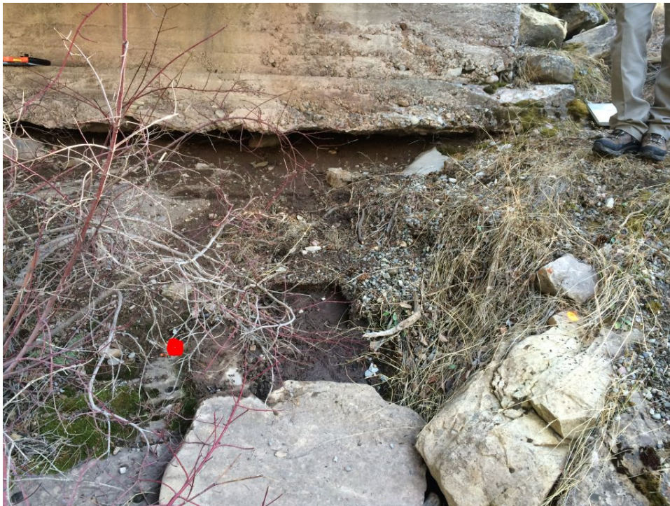
Photo 8 South Abutment West Side (outcrop marked)
