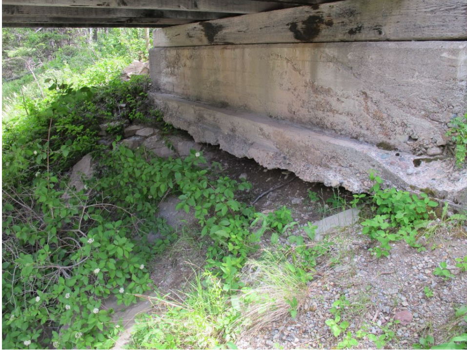
Photo 5 South Abutment Showing Erosion at Face
