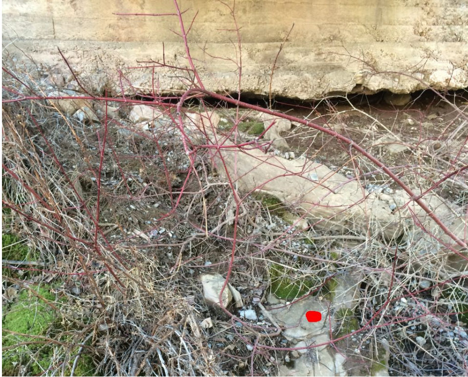
Photo 7 South Abutment East Side (outcrop marked)
