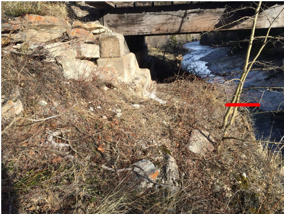
Photo 4 North Abutment (outcrop marked)
