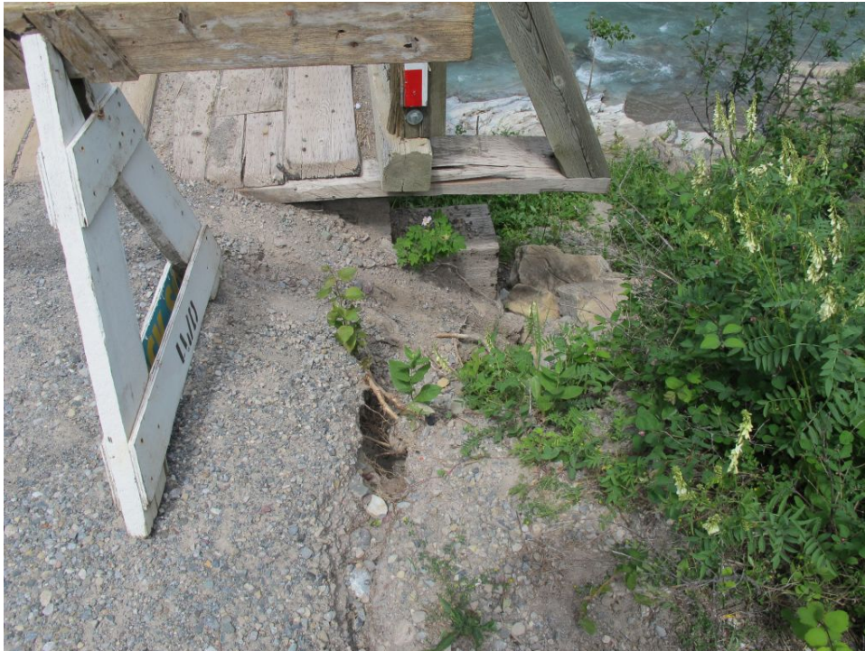
Photo 6 South Abutment Showing Erosion at Backfill
