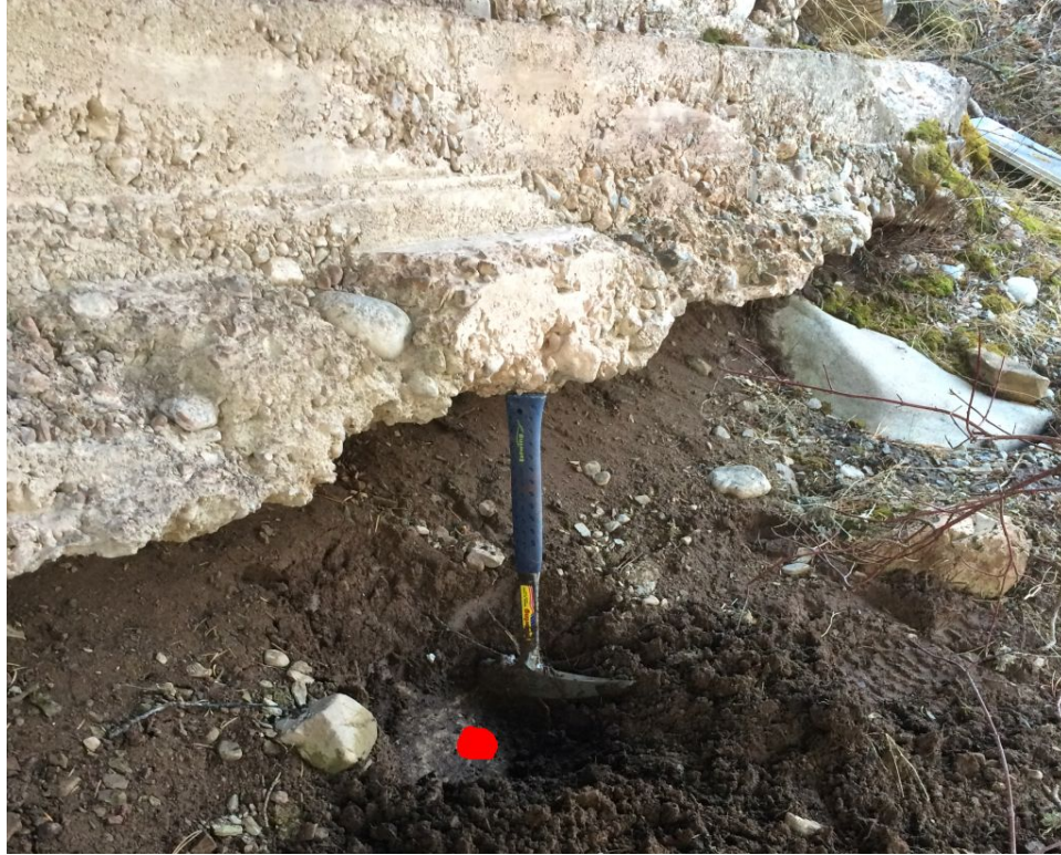
Photo 9 South Abutment West Side (outcrop at face marked)
