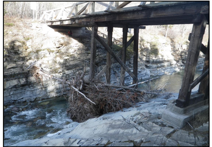
Photo 1: Canyon Church Camp Bridge over Blakiston Creek
