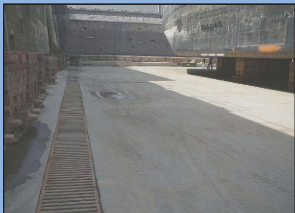
Example of a dock floor that would pass inspection.
