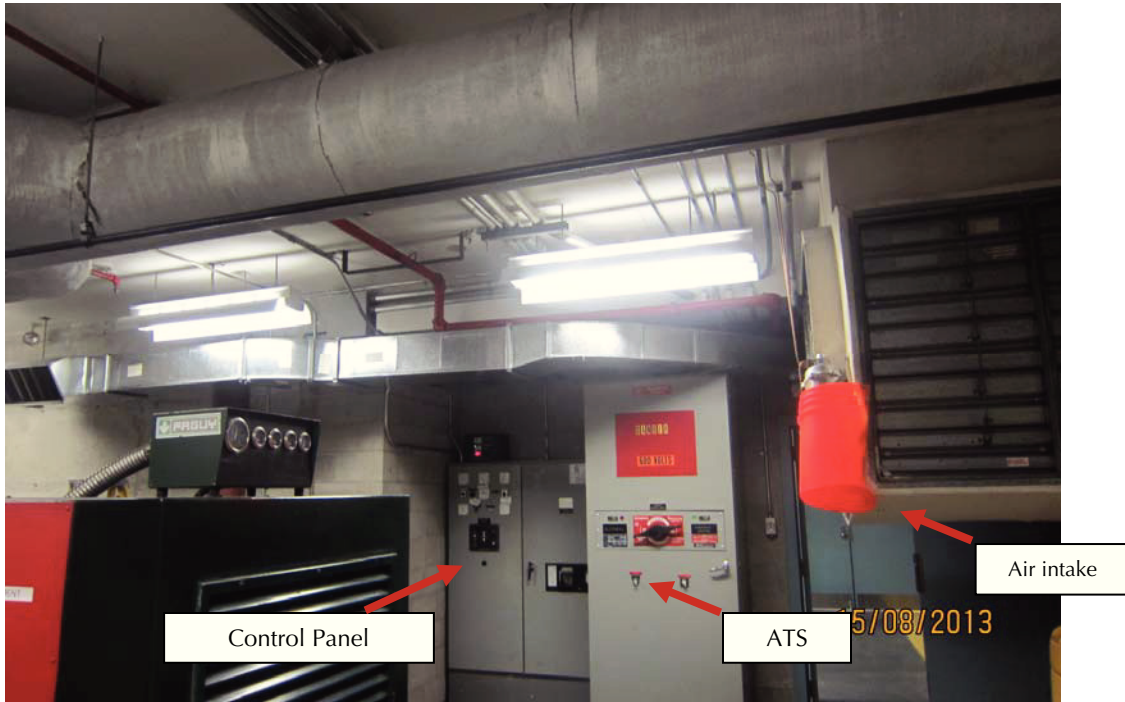
3 – Generator control panel, existing ATS and air intake
