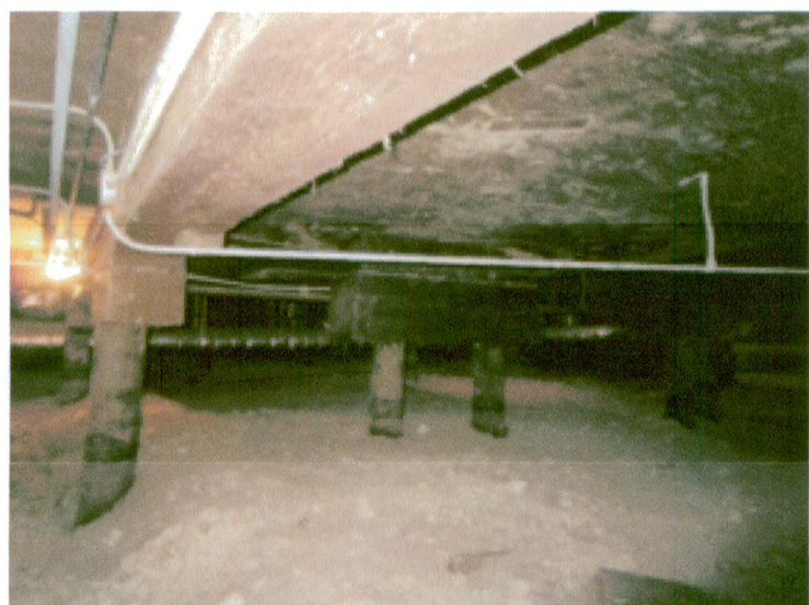
20 VIEW OF PILE SUPPORTING UPPER FLOOR POST
