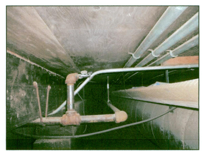
TYPICAL CRAWLSPACE SPRINKLER (2) NTS
