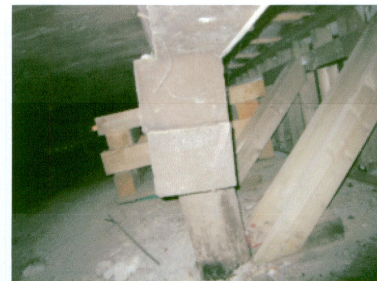
25 GENERAL VIEW OF EXISTING PILE CAP AND GROUND FLOOR BEAM THAT ARE ROTATED
