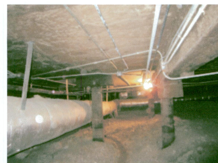
19 VIEW OF PILE SUPPORTING UPPER FLOOR POST
