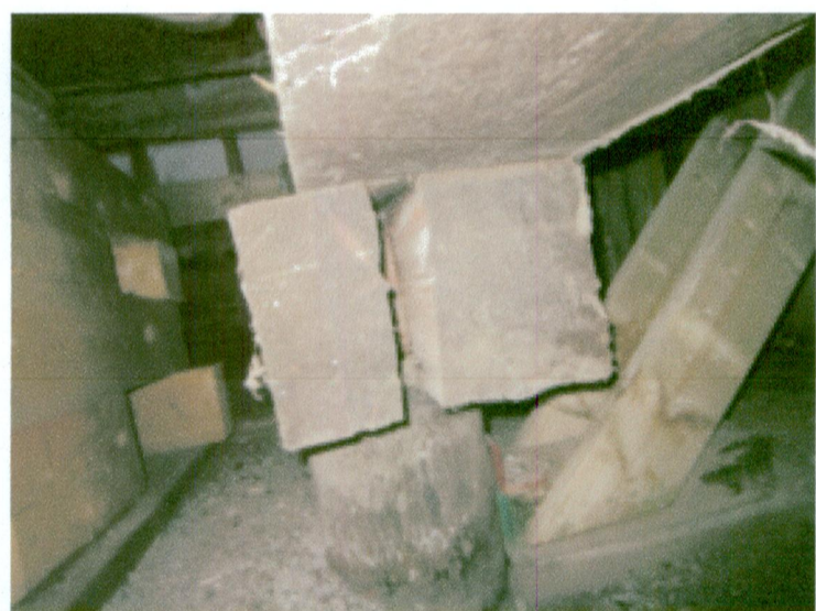
17 VIEW OF SPLITTED PILE CAP AT NORTHWEST CORNER
