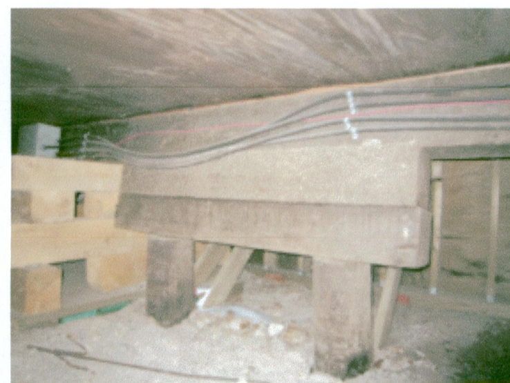
18 VIEW OF TYPICAL PILE SUPPORT AT SOUTH AND NORTH SIDE OF MAIN BUILDING
