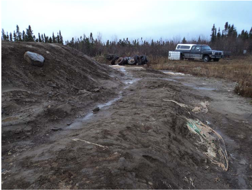
Photo 5. Berm, looking west – slightly weathered with reduced height.
