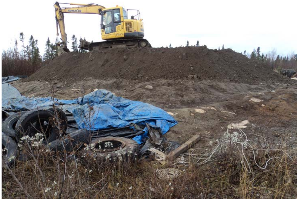
Photo 9. Turning Contaminated Soil Stockpile, looking north.
