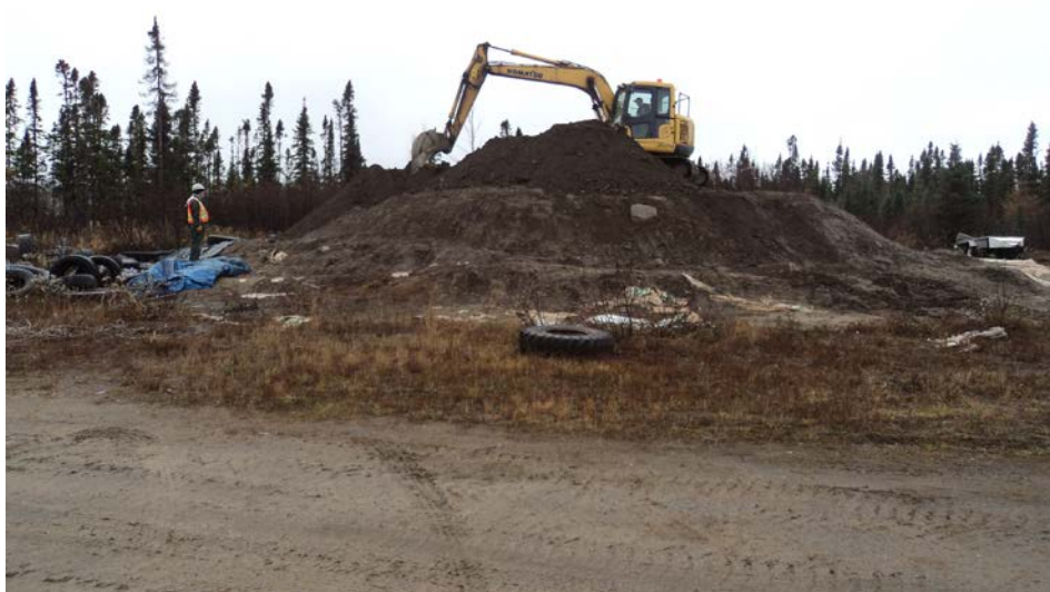
Photo 8. Turning Contaminated Soil Stockpile, looking west.
