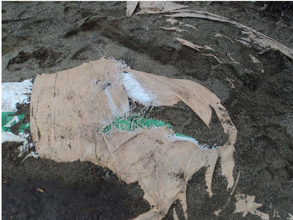
Photo 6. Weathered ripped area of berm.
