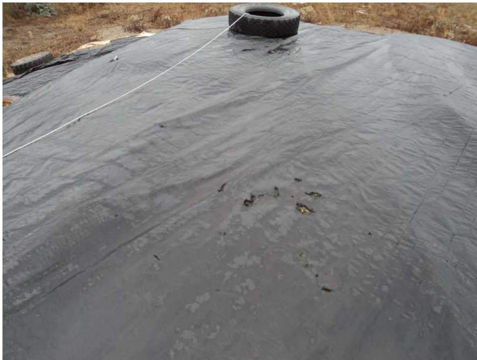
Photo 4. Small tears in covering tarp.
