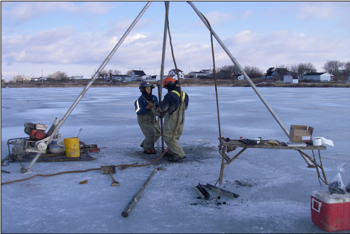
Photo 9 - Boart Longyear Drill Crew Using the Tri-Pod Sampling System PRSS-07BH-28 (Coordinates: 5124163, 4599184)
