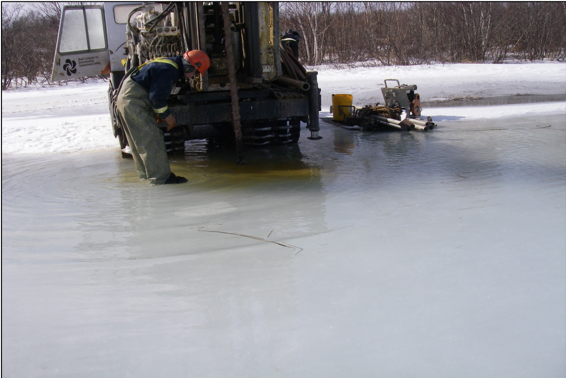
Photo 6 - CME 55 Drill Preparing Borehole For Sampling PRSS-07BH-17 (Coordinates: 5124010, 4599108)
