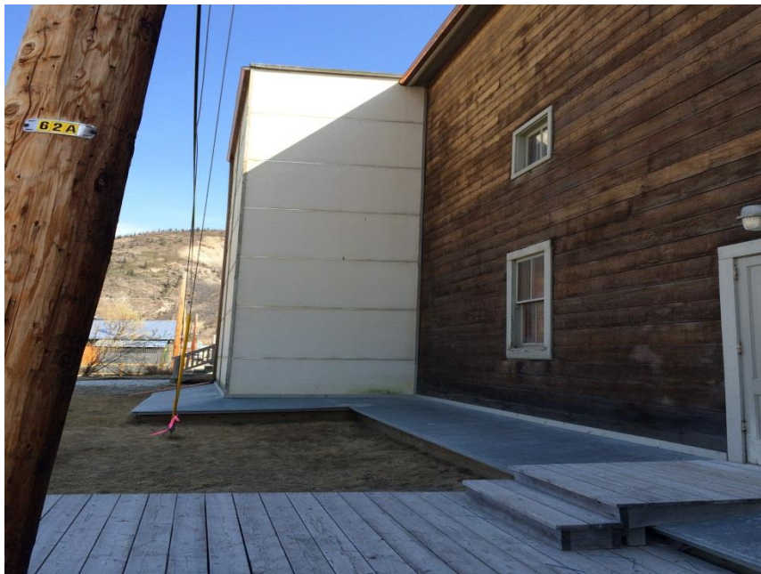
Photo 2: Palace Grand Theater - View of exterior skirting that can be removed to create an exterior access point to the crawlspace.
