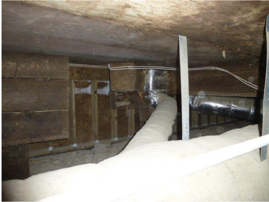
Photo 11: Palace Grand Theater Crawlspace – Typical HVAC ducting locations, insulation and installation.
