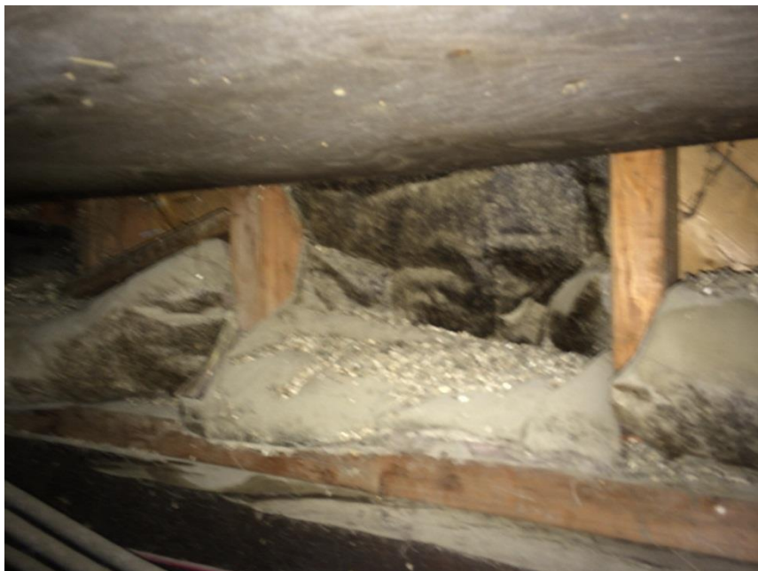
Photo 4: Palace Grand Theater CrawlSpace - Asbestos-contaminated fiberglass insulation in the crawl space at perimeter walls.
