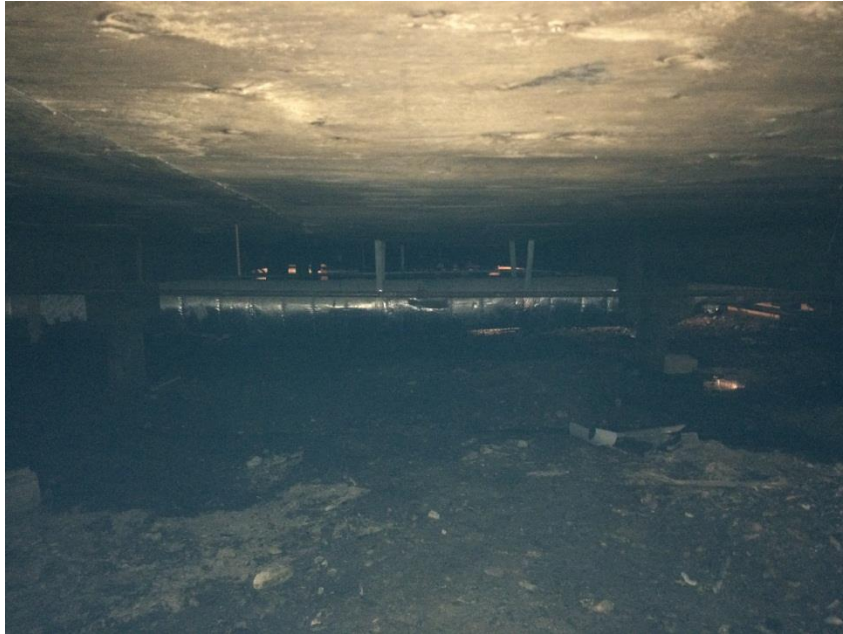
Photo 7: Palace Grand Theater Crawlspace - Plywood attached to underside of main floor joists and HVAC ducts hung from the plywood/joists.
