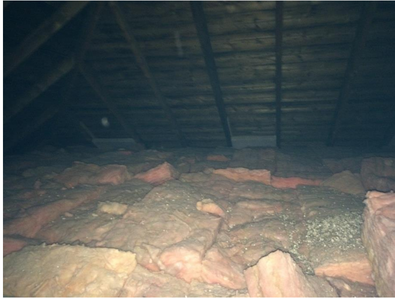
Photo 19: Commanding Officer's Quarters - Fibreglass batt insulation laid on top of asbestos-containing vermiculite insulation in the attic space.
