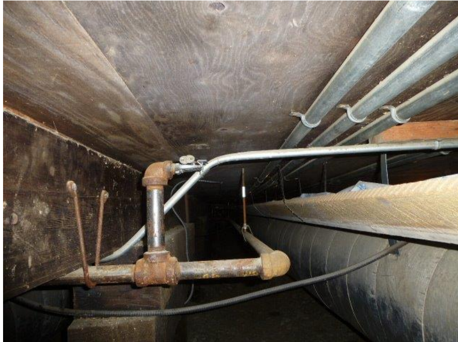
Photo 13: Palace Grand Theater CrawlSpace – Typical HVAC, sprinkler and electrical conduit attached to underside of plywood.
