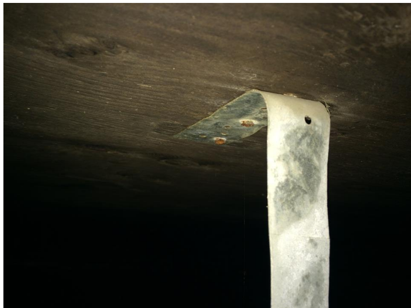
Photo 8: Palace Grand Theater Crawlspace – Typical hanger attachment for HVAC ducting to underside of plywood in the crawlspace.
