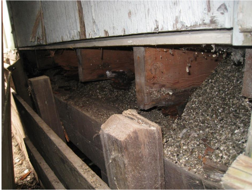
Photo 5: Palace Grand Theater CrawlSpace - Asbestos-containing vermiculite insulation to be removed from the “ceiling” space of the crawl space as seen from the exterior when skirting was removed.
