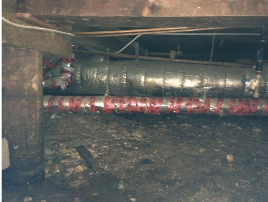
Photo 3 Palace Grand Theater CrawlSpace - Non-asbestos foil-wrapped fiberglass insulation to be removed from HVAC ducting in the crawl space.
