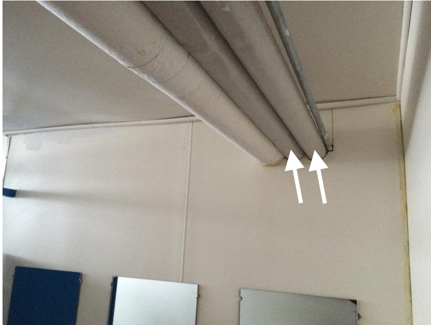
Photo 15: Palace Grand Theater - Asbestos-containing pipe wrap in Room 116 Women's Washroom.
