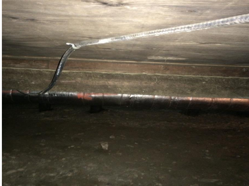
Photo 10: Palace Grand Theater Crawlspace - Electrical wires/conduit and HVAC ducts hung from the plywood/joists.
