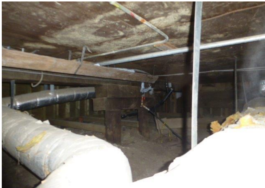
Photo 14: Palace Grand Theater CrawlSpace – Typical HVAC, sprinkler and electrical conduit attached to underside of plywood.
