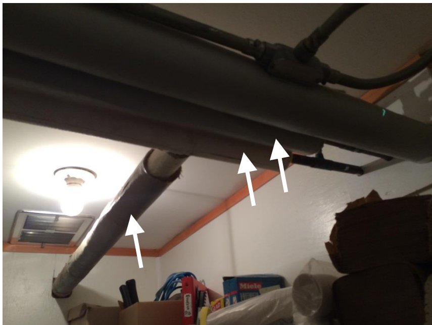
Photo 16: Palace Grand Theater - Asbestos-containing pipe wrap in Room 117 Janitor's Washroom.
