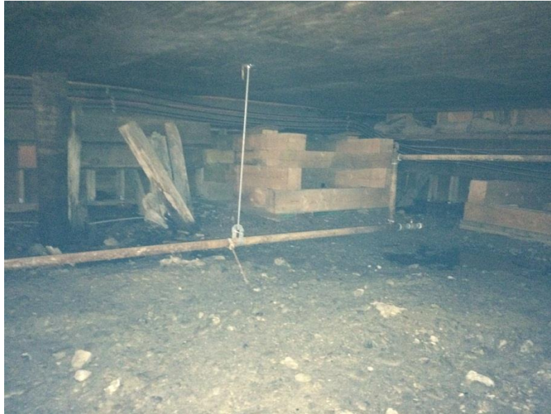
Photo 9: Palace Grand Theater Crawlspace - Fire suppression/sprinkler lines hung from the plywood/joists.
