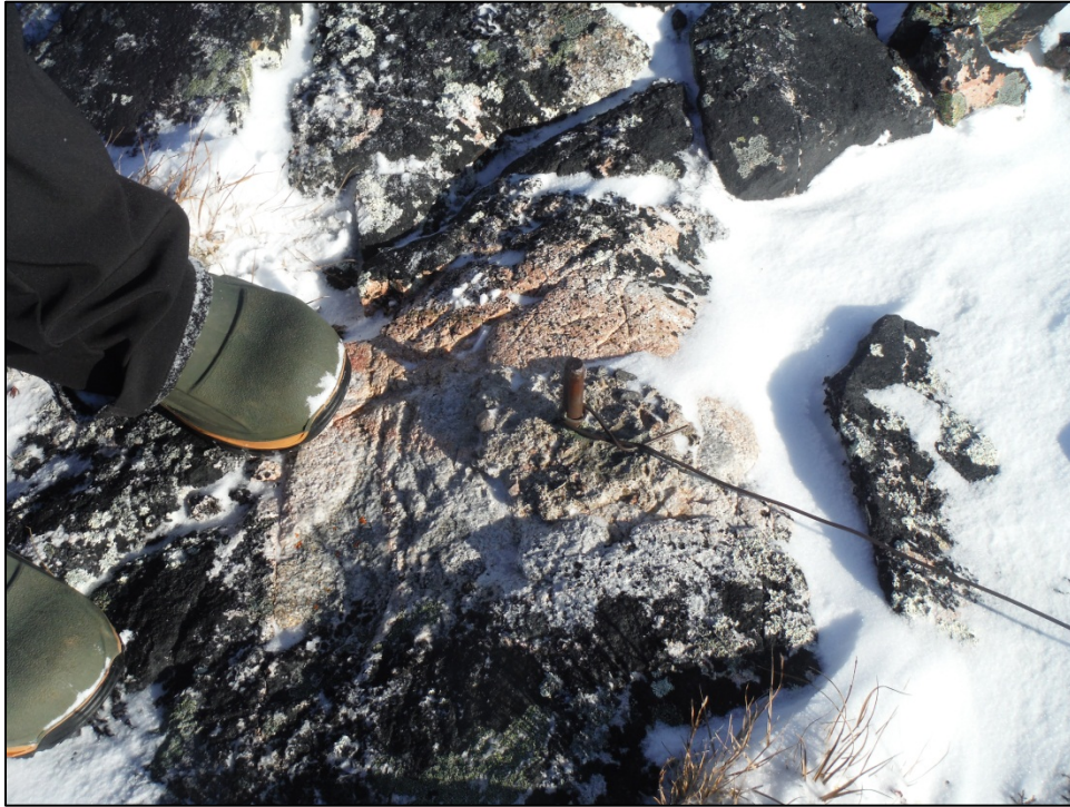
Photograph 13 – Exposed grounding stake for existing tower
