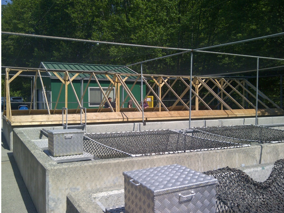
Figure 4 - Existing hoarding forms provided by DFO
