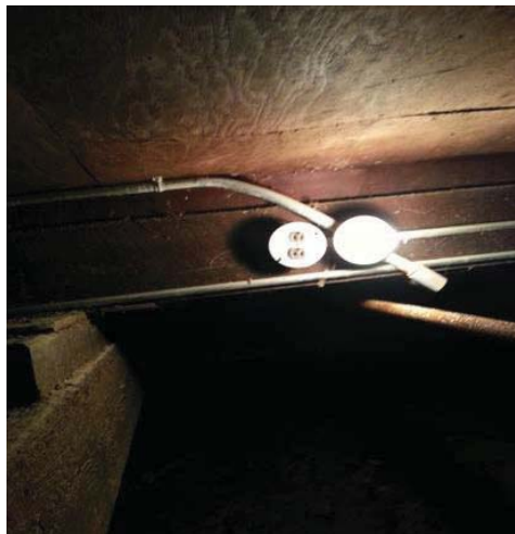
Keyless Light Fixtures and Receptacles in the crawl space
