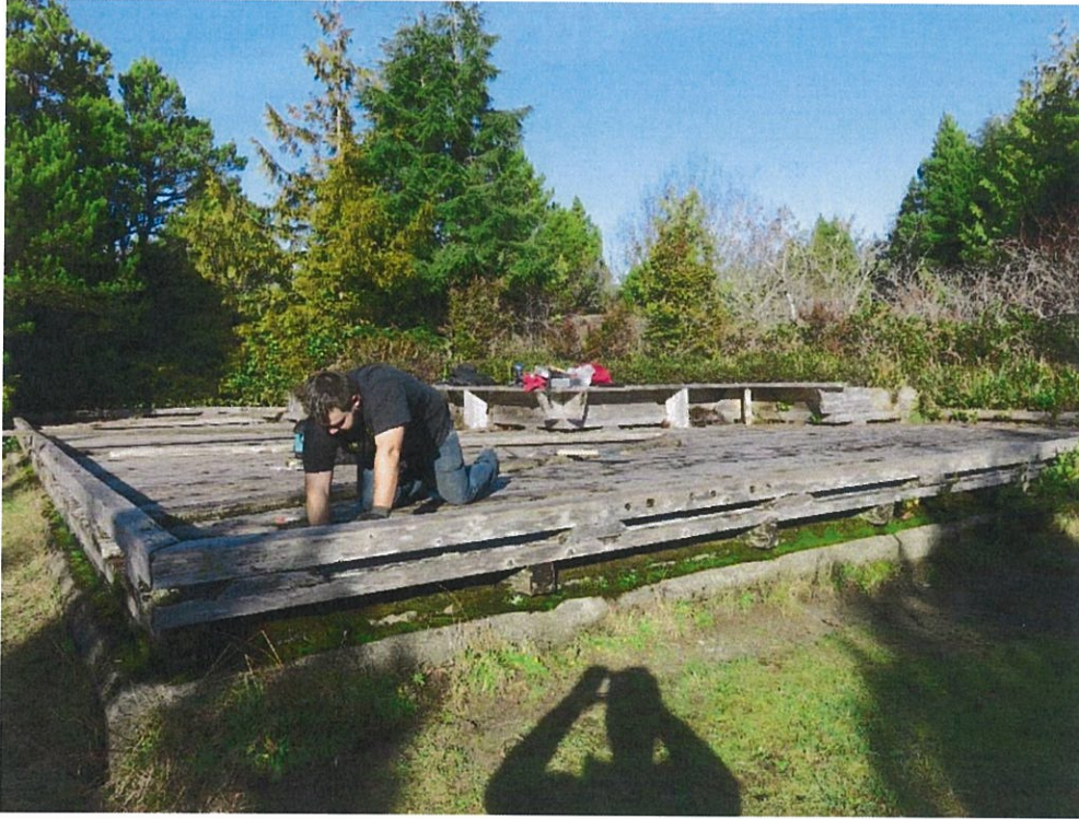
Photo 1 - Top South Platform scanning for reinforcement at location A1.
