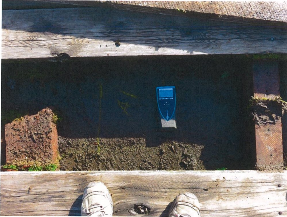
Photo 12 – Profoscope scanning of slab on grade.
