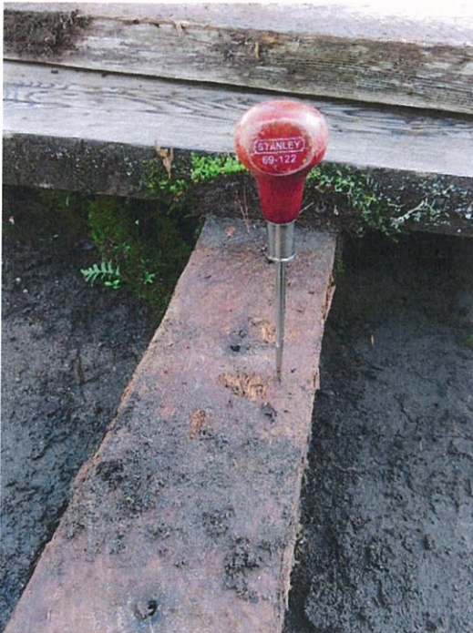
Photo 11 – Timber sleepers typically in good condition in test opening areas.
