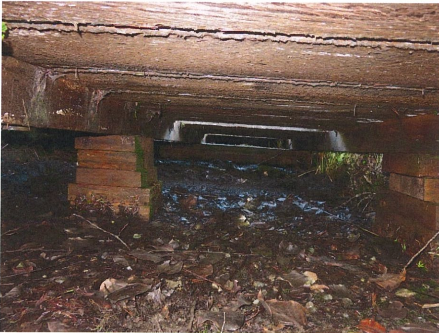
Photo 4 – Supports in area of suspended deck.
