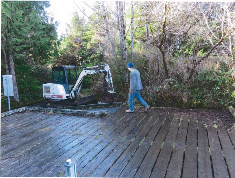
Photo 2 - Lower Northeast Platform – Excavator approaching deck
