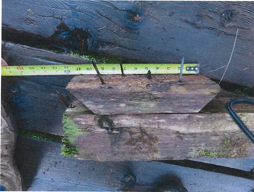
Photo 5 – Fasteners at spacer below top rail.
