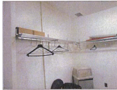
Photo 2, 2 nd floor closet, plaster does not contain asbestos,(sample 0006A-C)
