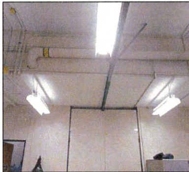
Photo 5 – Cementitious parge at ceiling, beginning of room 120
