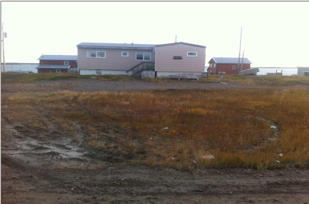
Photo 2: Looking north through the project site at the derelict house currently occupying the site.
