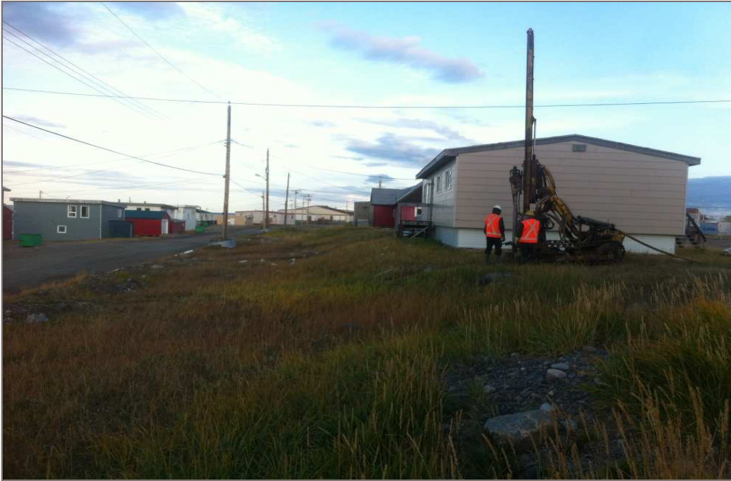
Photo 11: Looking east through the project site as the driller begins to drill Probehole 4 at the western side of the unoccupied house.
