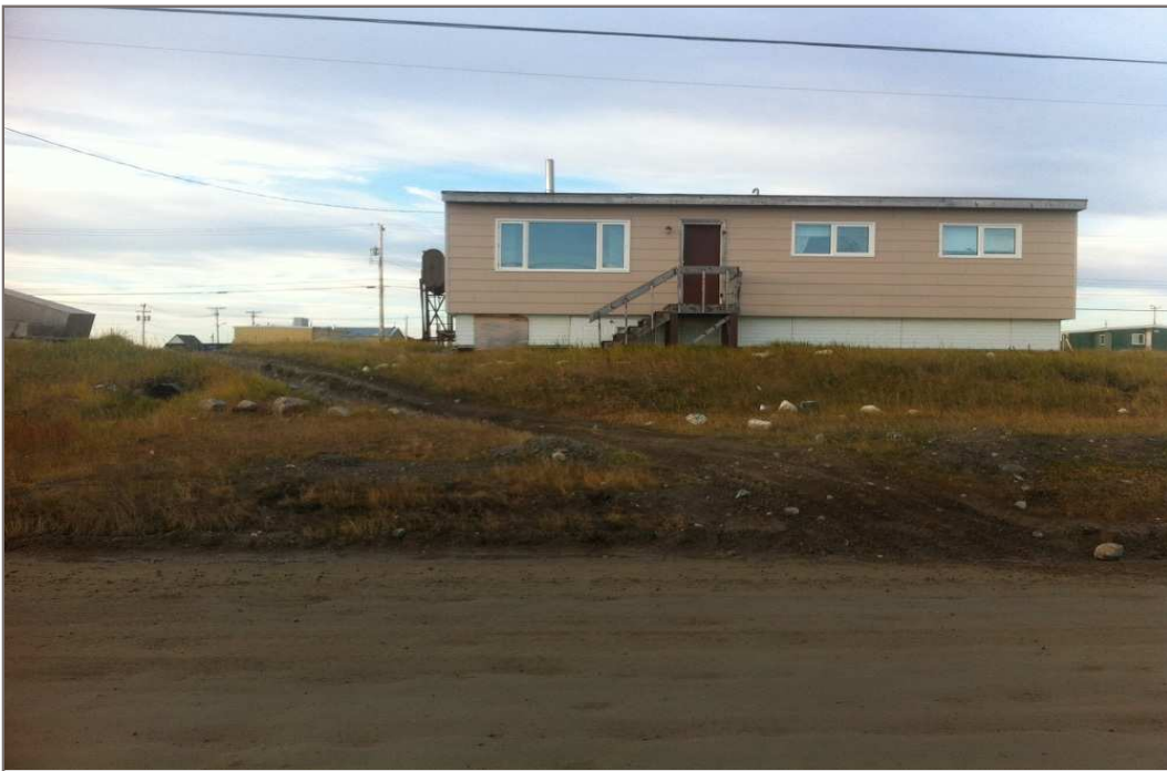
Photo 4: Looking south through the project site. The height of the fill embankment is almost equal to the height of the house on site.
