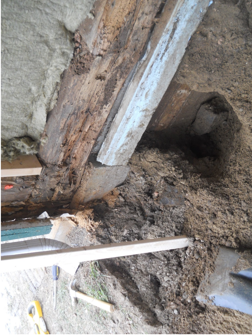
Photo 3 – Northeast corner of the bathroom building (a section of the exposed foundations is shown)
