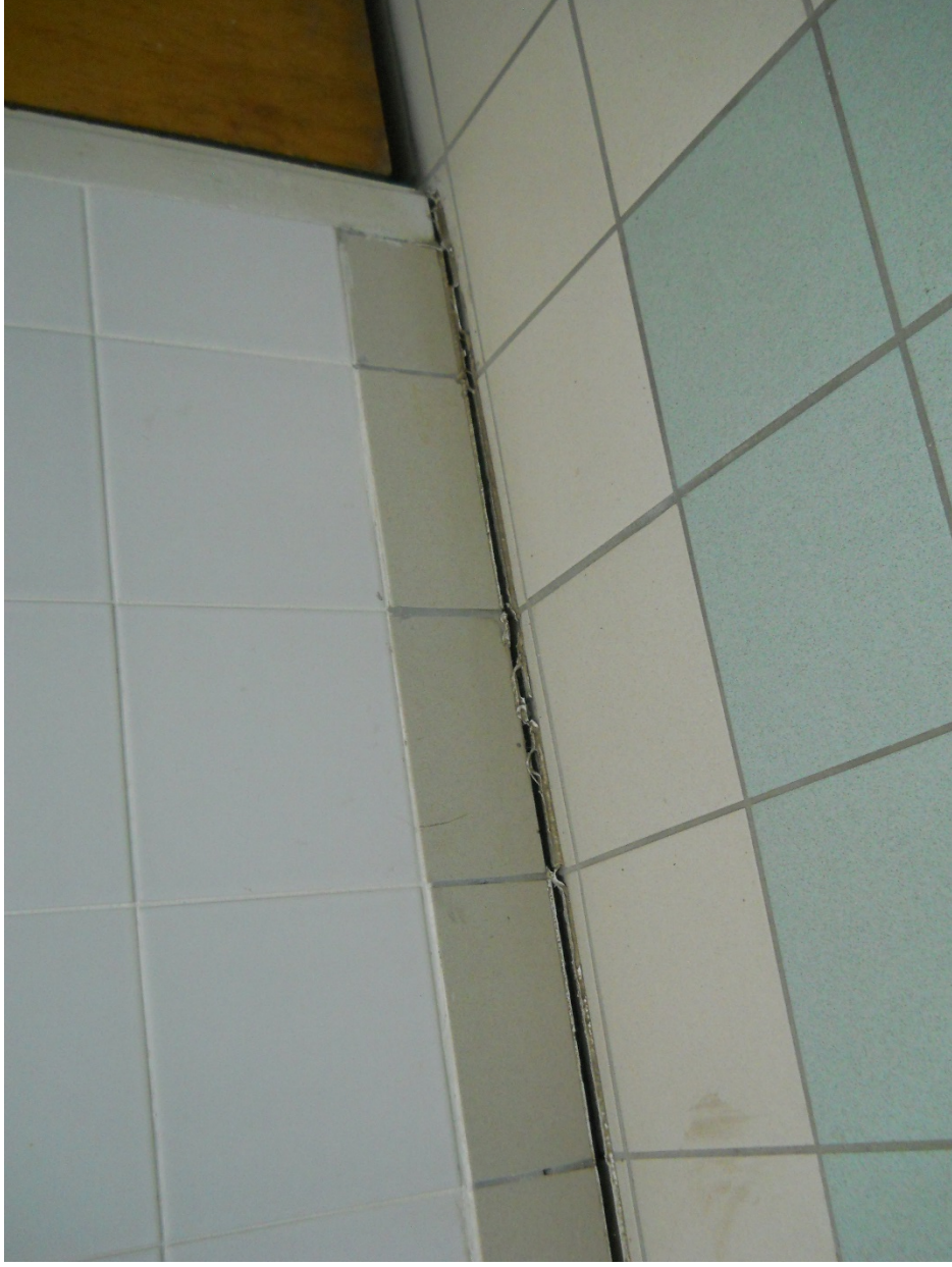
Photo 1 – Separation between the ground slab and the bathroom's interior wall.
