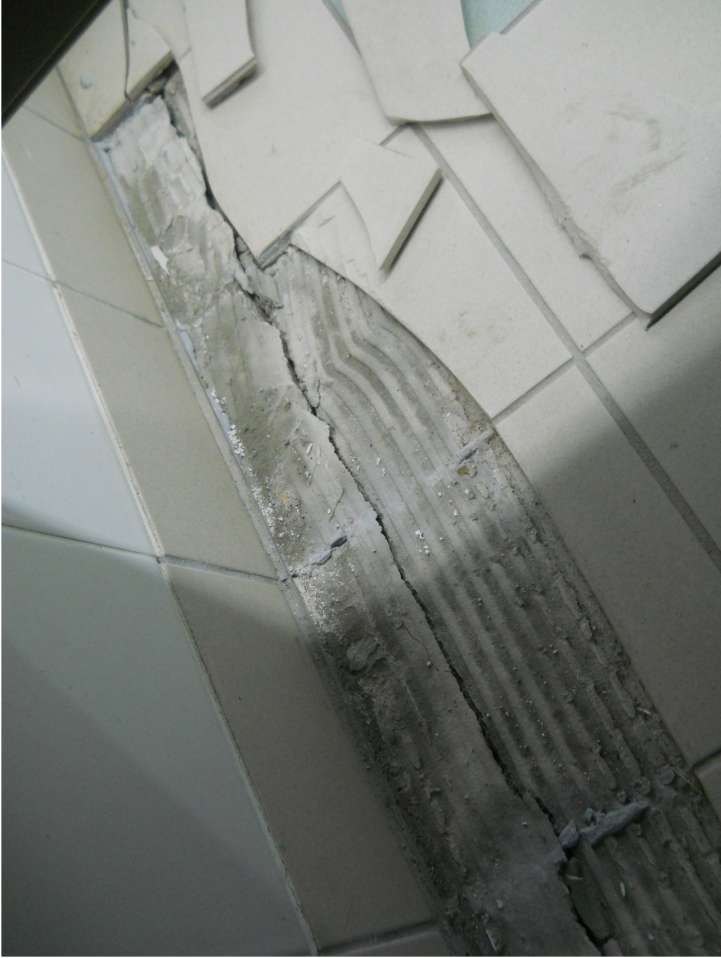
Photo 2 – Crack in the concrete ground slab along the bathroom's north wall.
