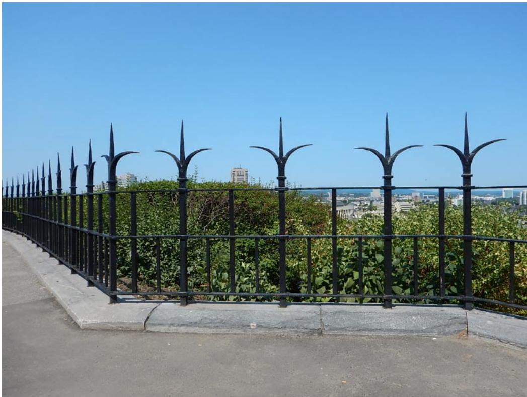
Figure 3 - Showing existing condition at the Lookout with capstones at grade level and uneven ironwork panels.
