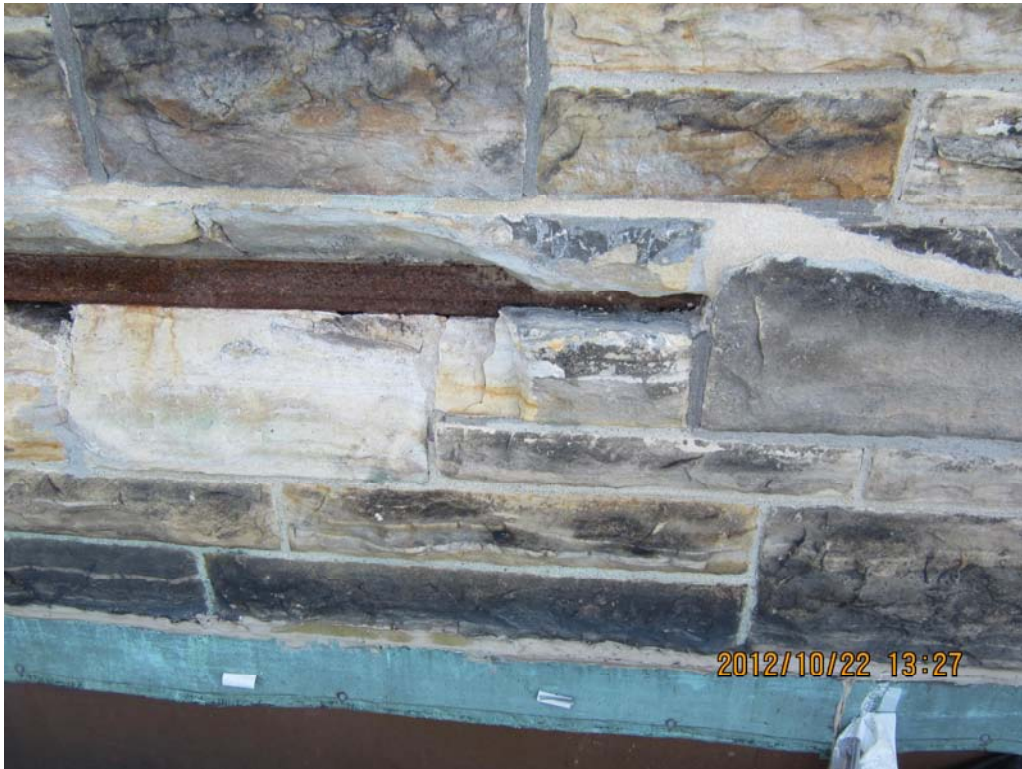
PHOTOGRAPH NO. 7 – Exterior cracked stone repairs and repointed joints.
