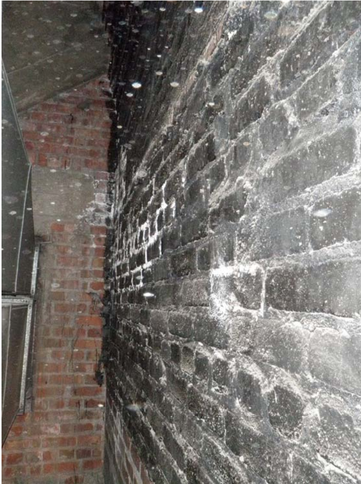
PHOTOGRAPH NO. 9 – Efflorescence of interior face of masonry wall.
