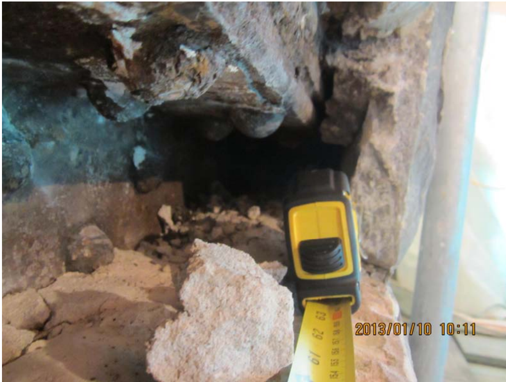
PHOTOGRAPH NO. 13 – Void between exterior stone and steel girder web at west side of North Gable.
