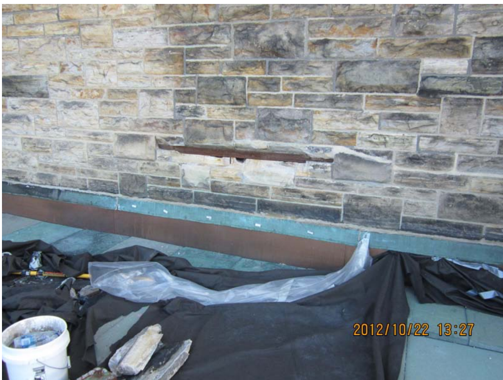
PHOTOGRAPH NO. 2 – Exposed steel girder top flange at the west side of the North Gable.
