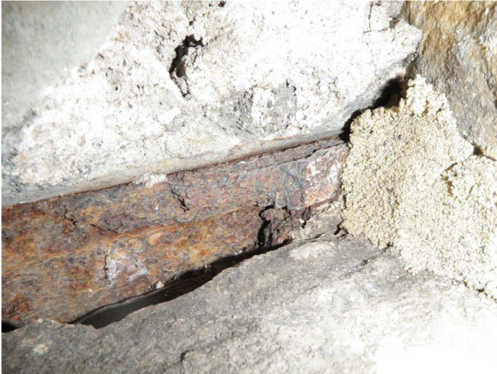
PHOTOGRAPH NO. 5 – Evidence of structural flaking on the edge of the exposed built-up top flange of the steel girder.
