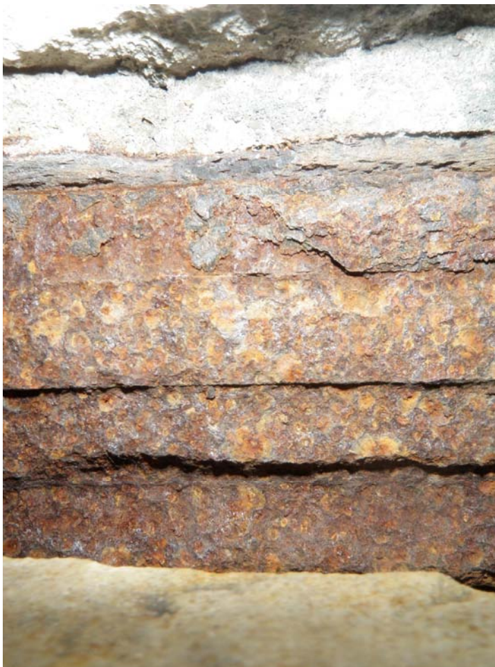
PHOTOGRAPH NO. 4 – Exposed built-up top flange of steel girder.
