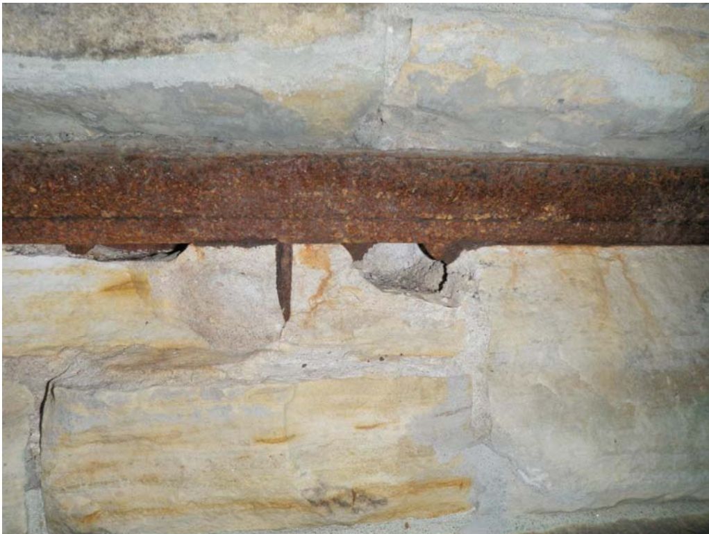
PHOTOGRAPH NO. 6 – Exposed web stiffener of steel girder.
