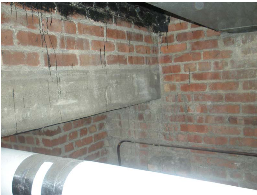
PHOTOGRAPH NO. 8 – Bottom flange of steel girder encased in concrete.
