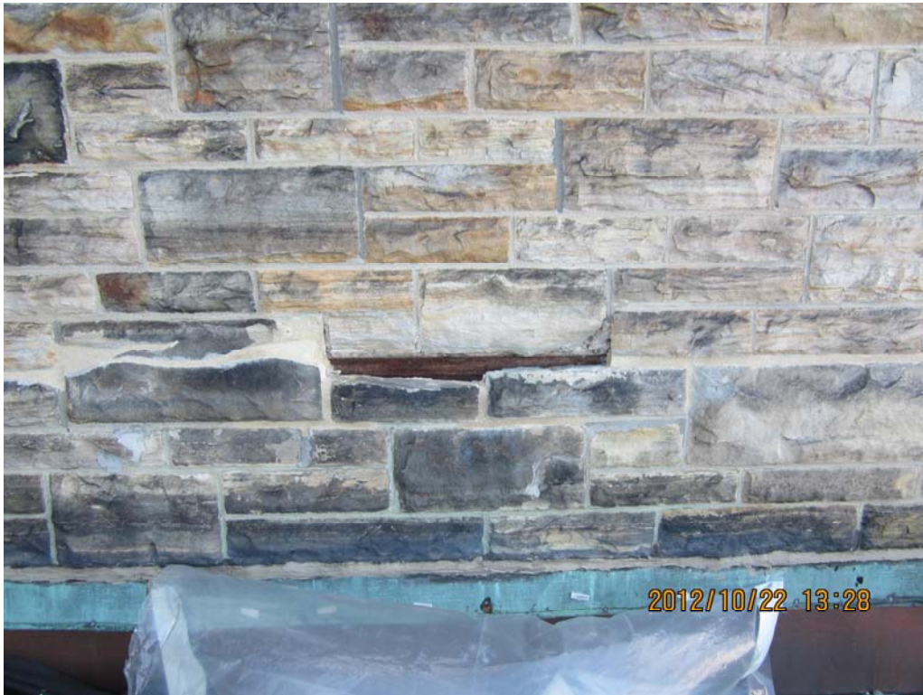
PHOTOGRAPH NO. 1 – Exposed steel girder top flange at the east side of the North Gable.
