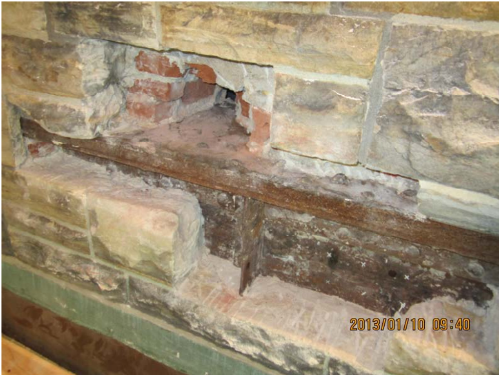
PHOTOGRAPH NO. 11 – Selective dismantling of masonry wall at the west side of the North Gable.
